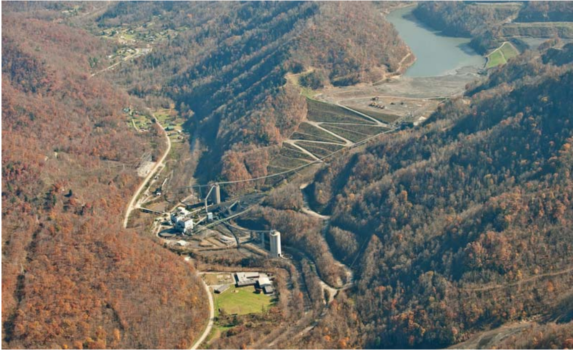
Figure 2: Upstream cross valley impoundment in Raleigh County, West Virginia where Marsh Fork Elementary operated at the base until 2013; photo credited to Carl Galie
