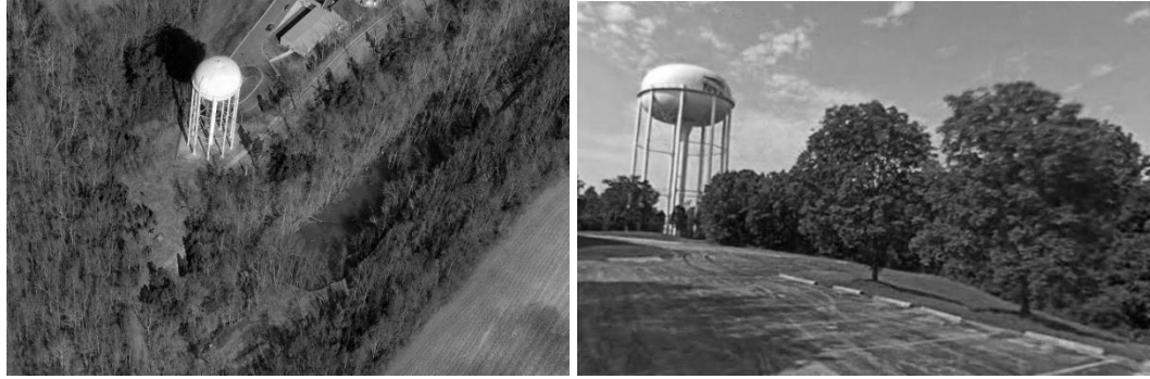
Figure 3.5: Aerial and Street View Images of Storage Tanks.
