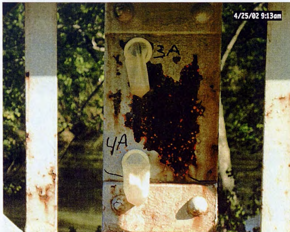
Figure 6 Testing in progress on KY 355 in Owen Co. for obtaining a sample using CHLOR-RID kit for analysis.
