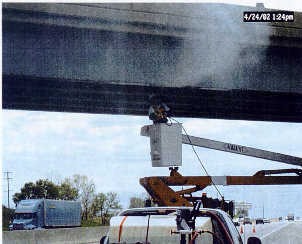
Figure 8 Pressure washing test area on I-71 N overpass over I-75 S.
