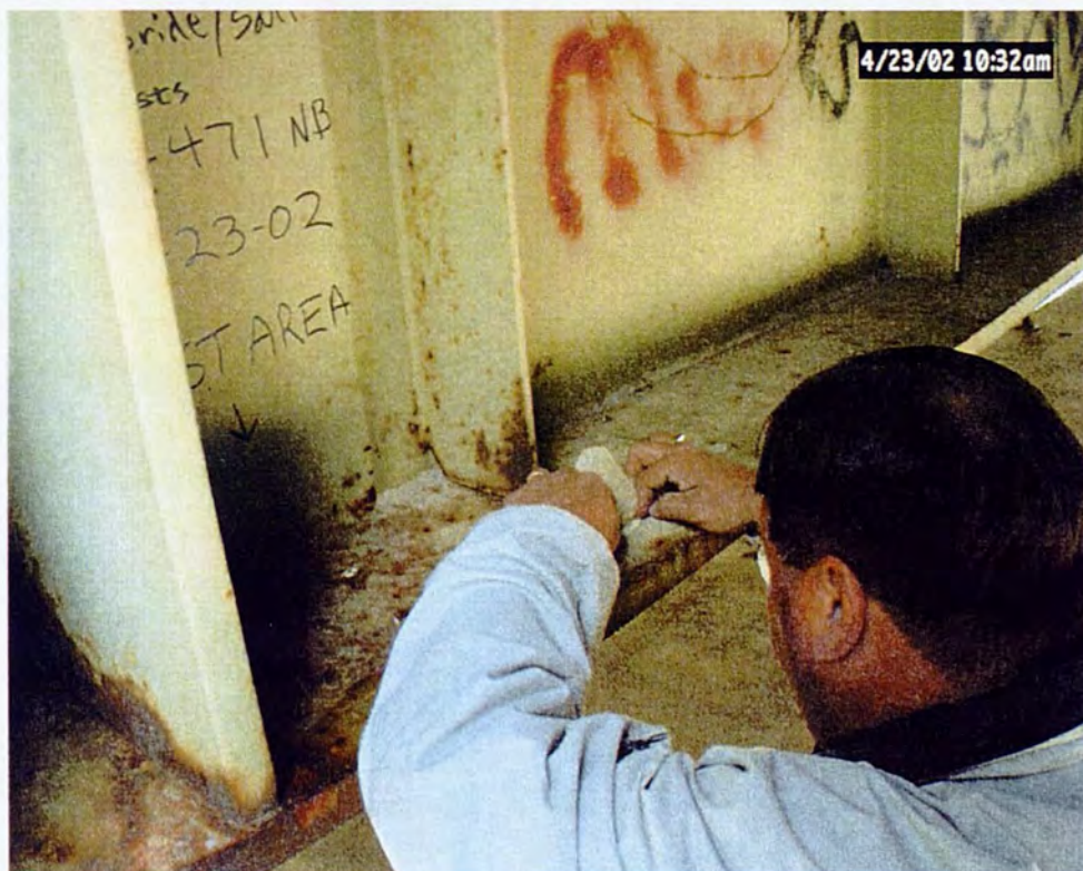
Figure 2 Technician installing sleeve on upper face of lower flange on floor beam (test area 1A).
