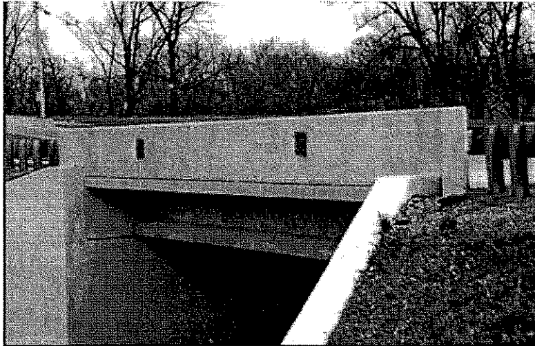
Figure 4.1. Rogers' Creek Bridge - Bourbon County
