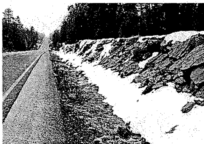
Figure 6 Typical Highway with Roadside Hazard Rating Equal to 6
