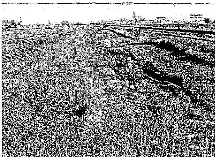
Figure 2 Typical Highway with Roadside Hazard Rating Equal to 2
