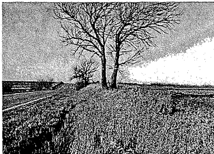
Figure 4 Typical Highway with Roadside Hazard Rating Equal to 4
