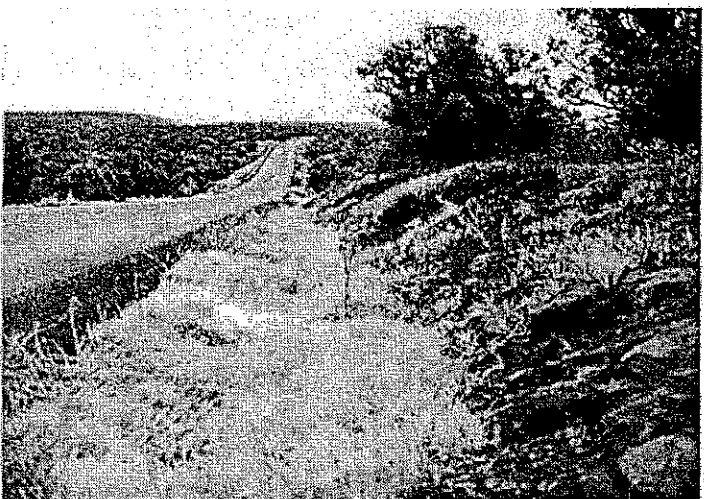
Figure 3 Typical Highway with Roadside Hazard Rating Equal to 3
