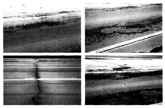
4. Conclusions About Site – From 0-0.29 miles north of US 42, there are many stress fractures of the pavement, although no base failures to report. After this section, the pavement looks better, but there are still many longitudinal and map cracks in a number of areas.
