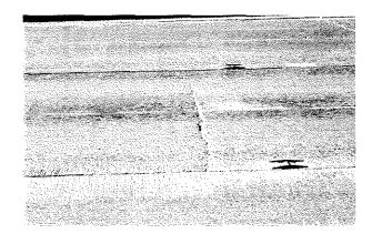
4. Conclusions About Site – Overall the pavement looks to be in good condition. There are a few cracks and many places where the pavement is breaking apart around areas where the pavement markers are missing. There are many bridges or overpasses on this section and consequently much of the pavement is on a bridge or ramp. A lack of shoulder space limits the ability to get more pictures for this site. Recommendation for the future would be to have right lane closed and more pictures taken.
