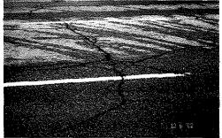
4. Conclusions About Site – Distresses at this site indicate a high volume of traffic. There are many cracks that need to be repaired. There appear to be no structural failures with the road, at this time. Careful monitoring is recommended.
