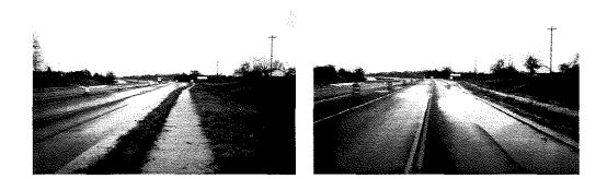
4. Conclusions About Site – The road appears to be in good structural condition. However, water has collected in the right lane and further drainage may be necessary. A follow-up survey should be performed to see how the road handles repeated loading once it is opened to traffic.
