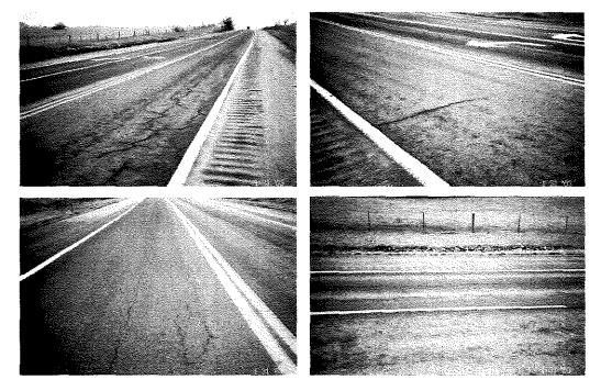
4. Conclusions About Site – Overall the road looks good, but there are many longitudinal cracks over the entire length of the project. These cracks should be patched and the road monitored for future stress problems.
