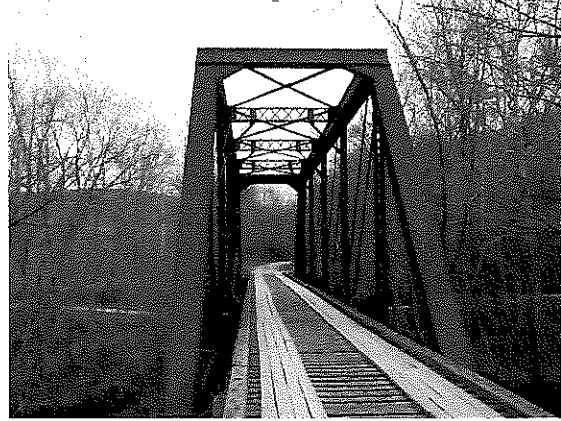
Bridge on Chesapeake & Ohio line, Carter County
