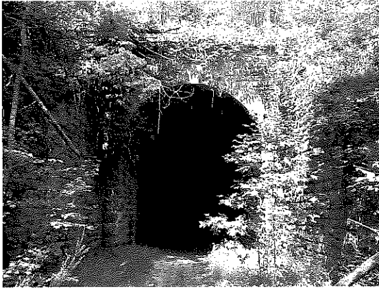
Tunnel south of Burnside on former CNO&TP
