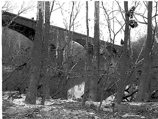
Yamacraw Bridge, McCreary County
