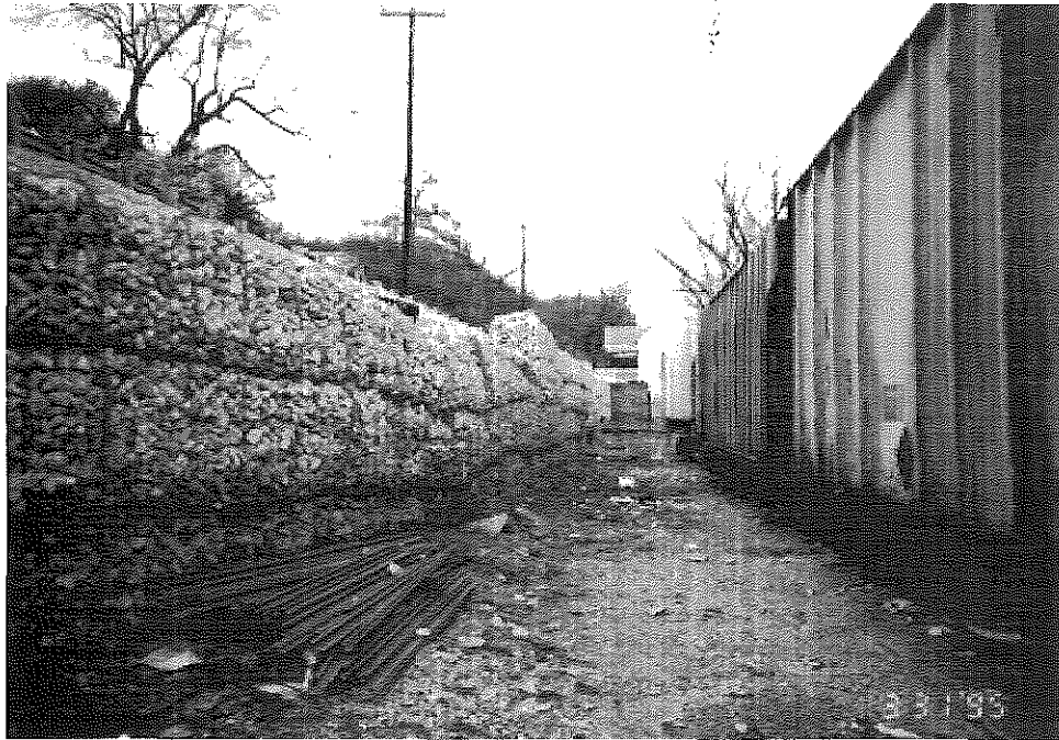
Figure 38: Gabion Wall on KY 8, Mason County
