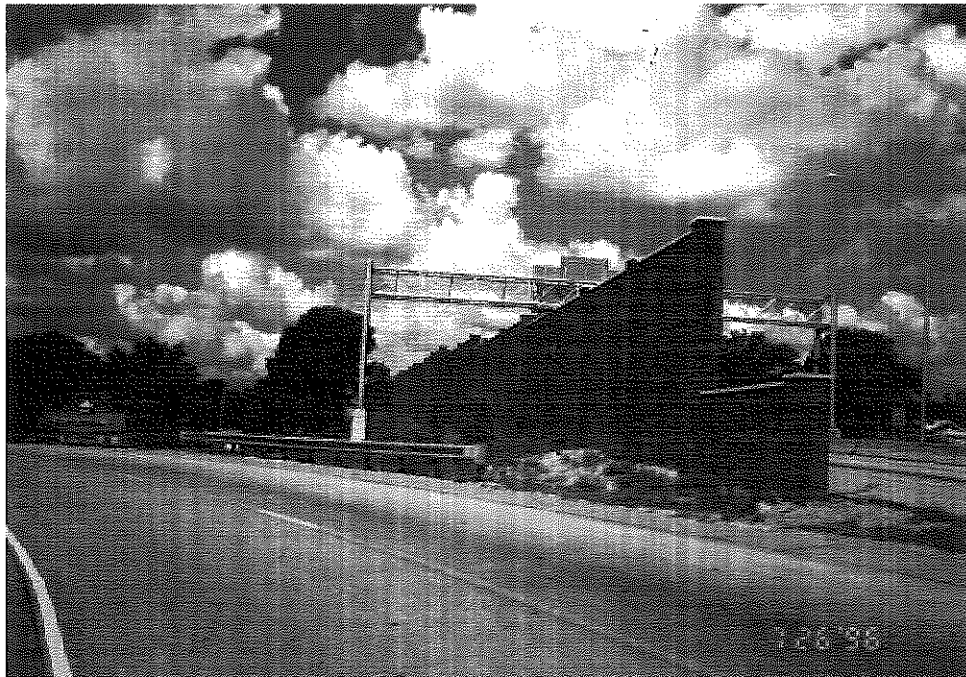
Figure 104: Brick Sound Wall (Jefferson County, I-264)
