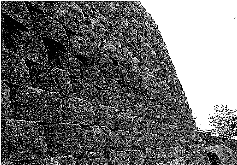
Figure 65a: Forward Displacement between Rows (sliding)
