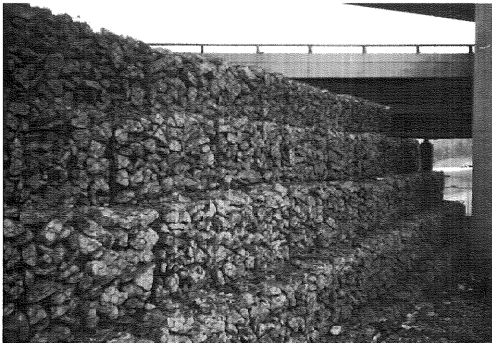
Figure 42: Gabion Wall on I-75, Kenton County
