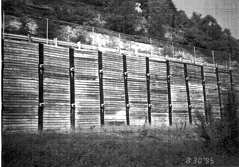
Figure 75: Tieback Attached to H-Pile (Greenup County, US 23)
