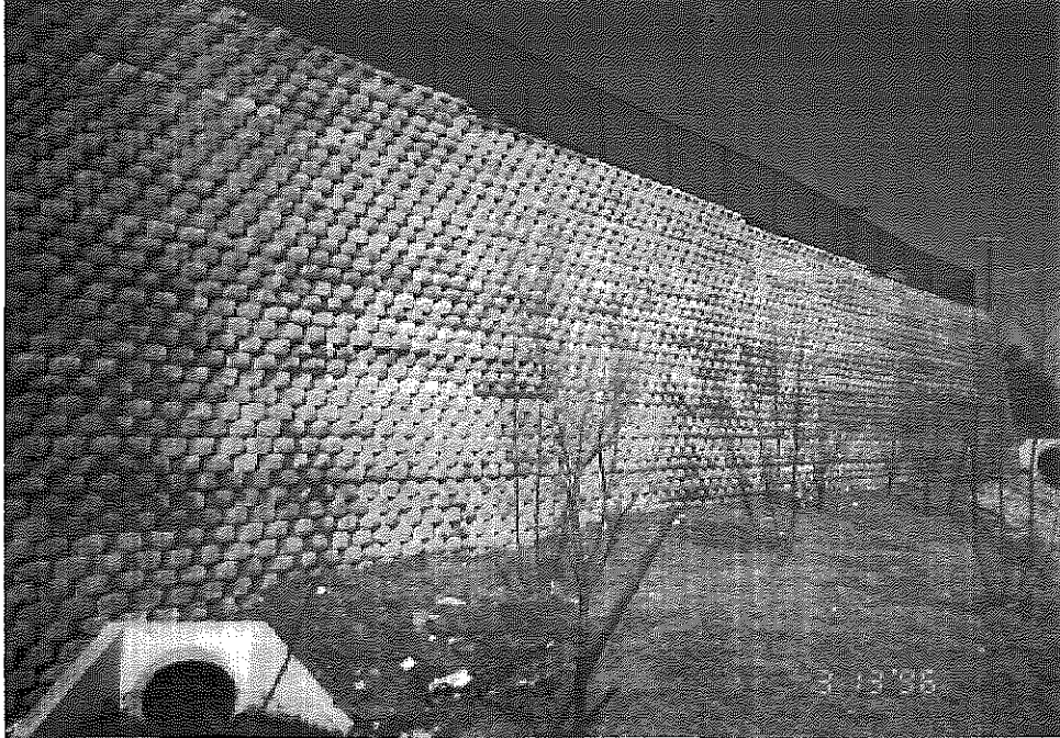
Figure 62: Keystone Block Wall, Richmond Rd. Lexington
