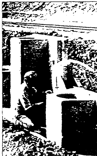
Abutment pier under construction.
