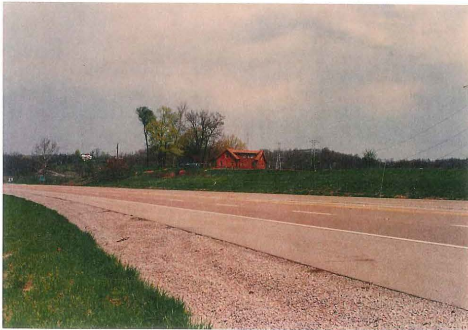
Figure 24. Daylighted, Untreated Drainage Blanket at AA Highway. Little Vegetation after Seven Years.
