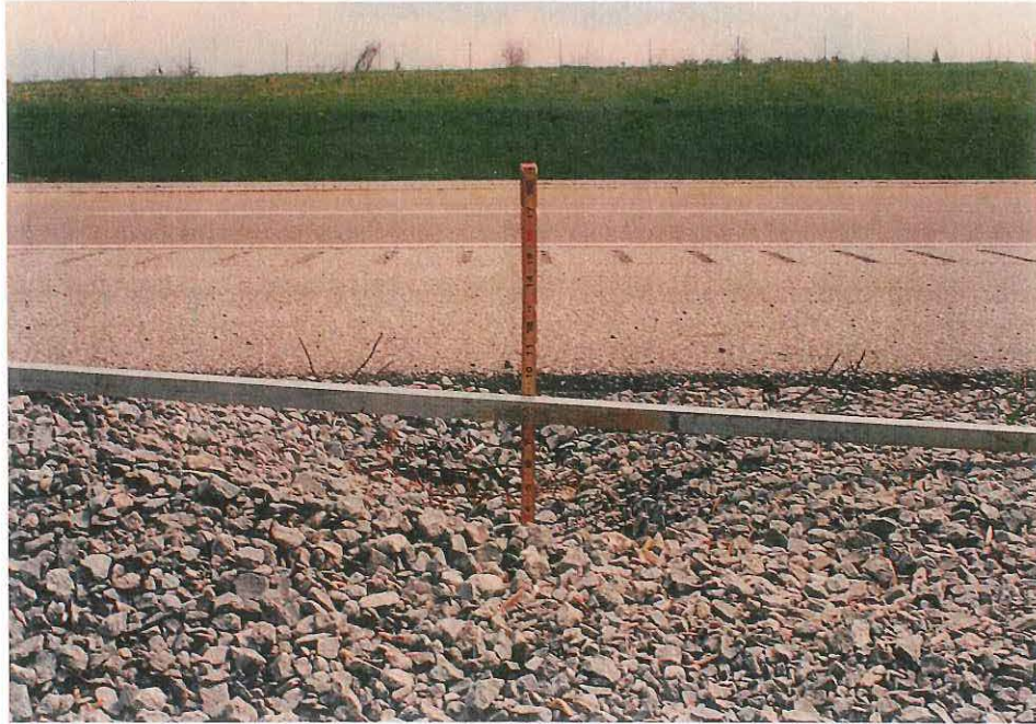
Figure 25. Untreated, Daylighted Drainage Blanket Displaced on Shoulders.
