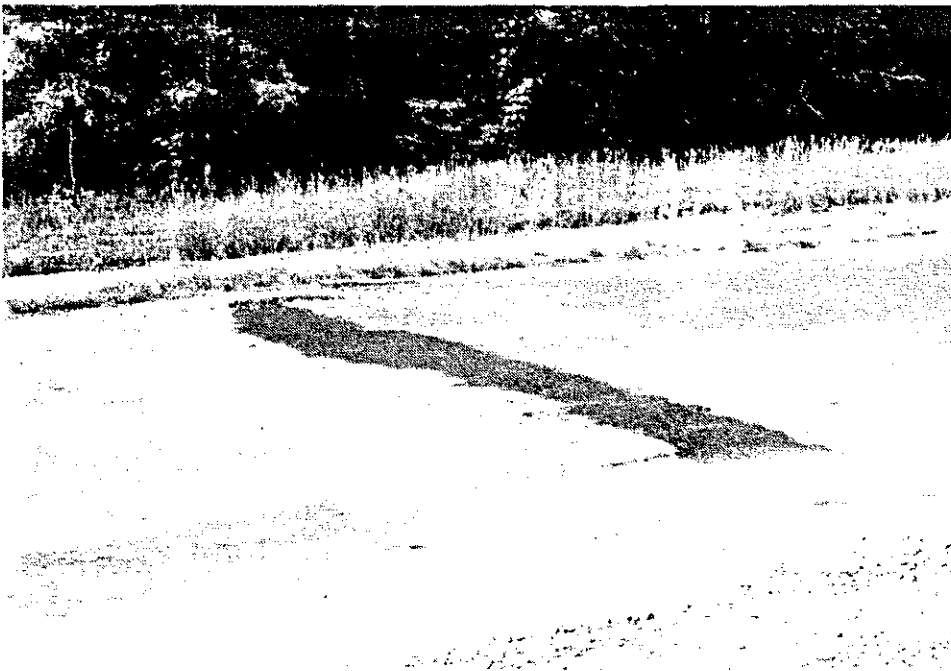
Figure 5. Photograph taken near STA 67+50 in May 1989 shows spot patching that was required after pavement milling activities.
