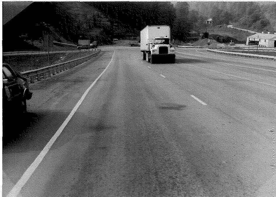
Figure F3. View of Northbound Shoulder Lane near Junction of KY 645 and KY 40.
