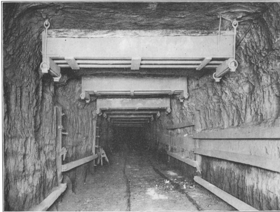
Figure 2.5 Barrier of Six B-2 Boxes in Mine Entry. Rock Dust is Protected by Oilcloth Covers [Rice et al. 1922].
