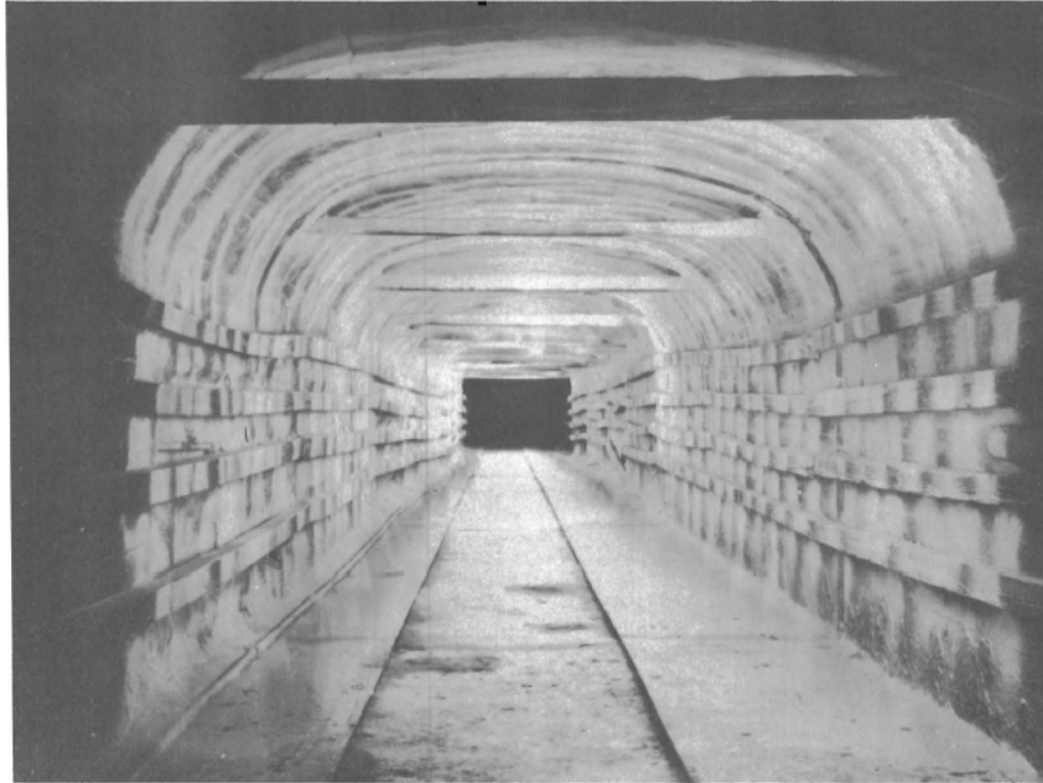
Figure 2.11 Mine Entry After Rock Dusting by Machine [Hartmann et al. 1950].
