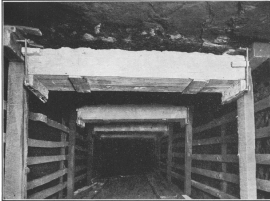
Figure 2.4 Box Barrier Type A Installed in Experimental Mine [Rice et al. 1922].
