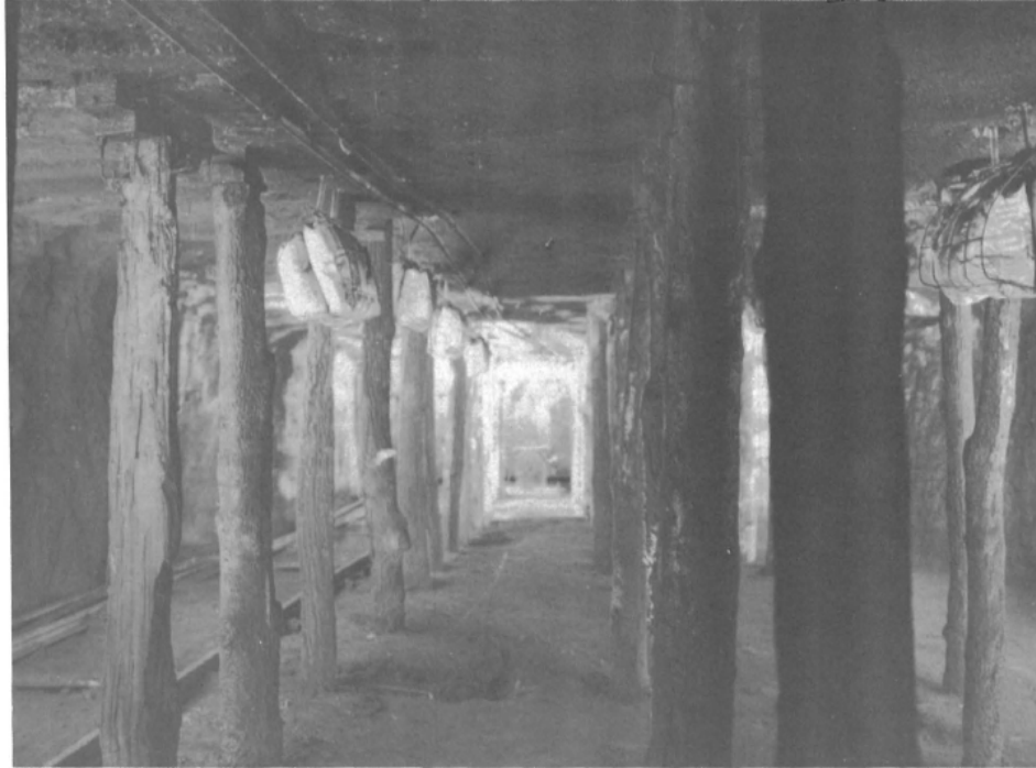
Figure 2.12 View of Room with Double Bag Rock Dust Units [Hartmann et al. 1950].
