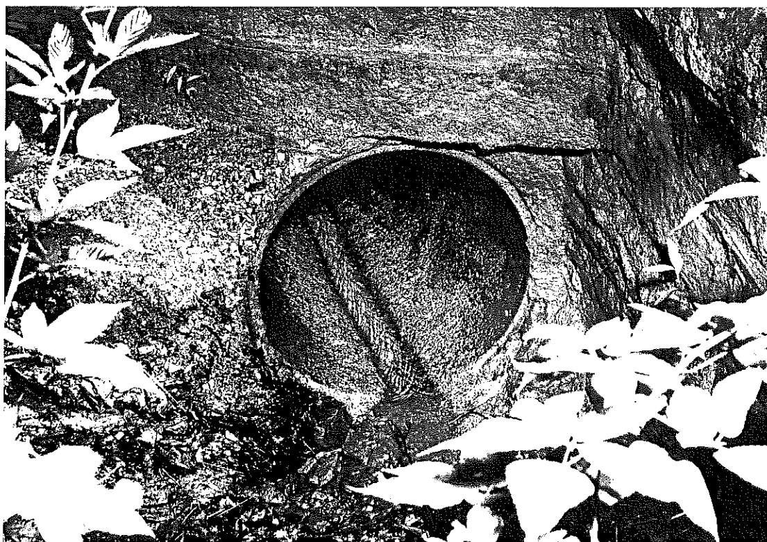
Fig. 6. An etched concrete cross-drain with sandstone masonry headwalls located on Ky. 74 in Bell County, 7 miles from Middlesboro. The source of water here was an abandoned mine and slack-pile. The water was continuous flow as evidenced by the corroded channel. It was not possible to determine how long the acidity had existed or what variations have occurred in the degree of acidity. The pipe, according to records available, has been in service since 1927.
