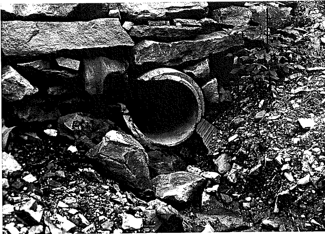
Fig. 10. Undermined culvert on Ky. 15 in Perry County, where water sample No. 1 was taken. The pipe has been pulled apart at joints near the upstream side of the fill, and water passes beneath the pipe to the downstream side during period of flow.
