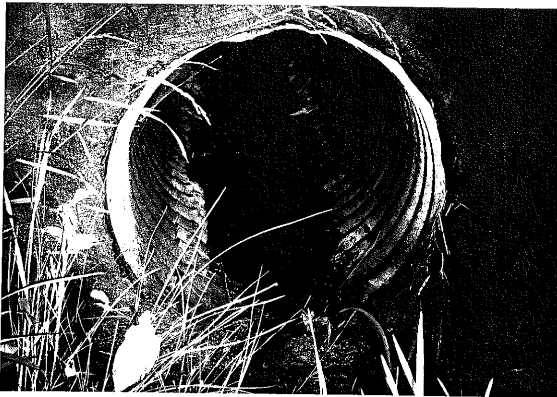
Fig. 7. Corrugated metal cross drain on US 60 at Bluestone. This culvert, for which the records indicate service-life of twenty-nine years, was replaced in the process of reconstructing the road shortly after this photograph was taken in June, 1950. The invert has been eaten away and water is standing in the channel. This static water (sample No. 16) showed a specific resistance of 930 ohms and positive qualitative tests for sulfates, chlorides, and calcium. It is not known definitely what the source of contamination has been or how long the corrosive agents have been active. There is a building-stone quarry above the road which has been operated intermittently over the past several years. Also, the location is on the very edge of the eastern coal field.
