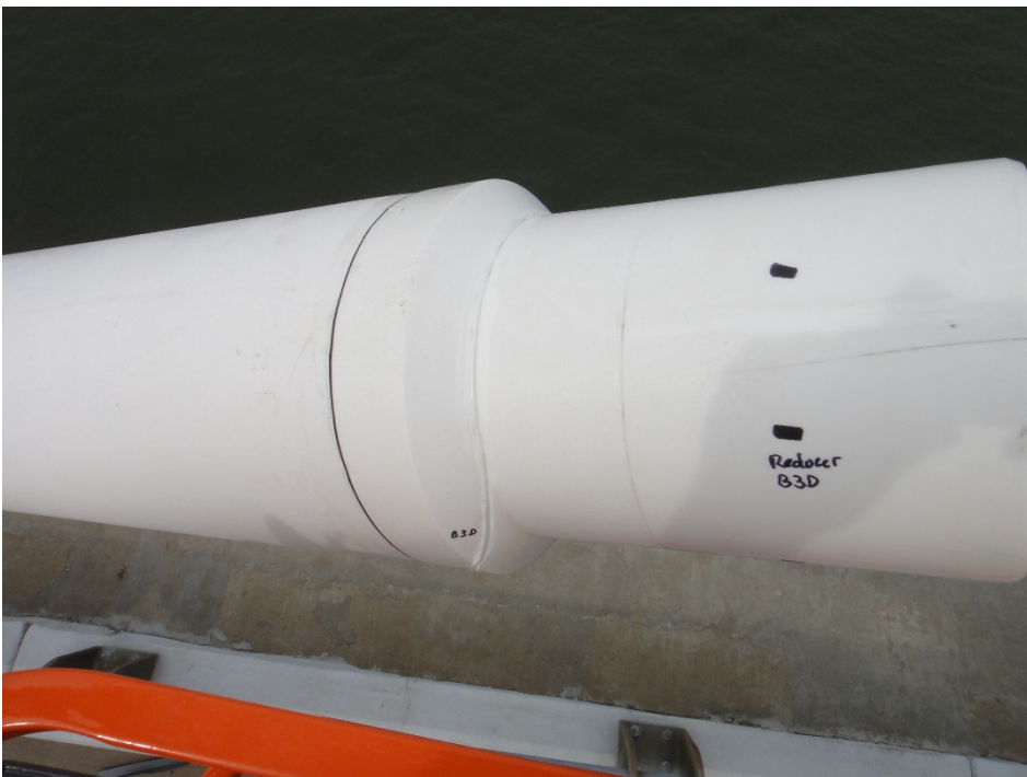
Figure 93. Completed Weld Repair in a Previously Cracked Reducer.
