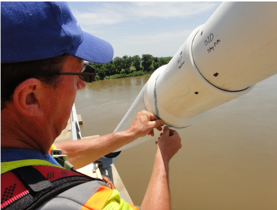
Figure 95. Applying Stopaq® Paste to a Seal Crack in a Reducer.
