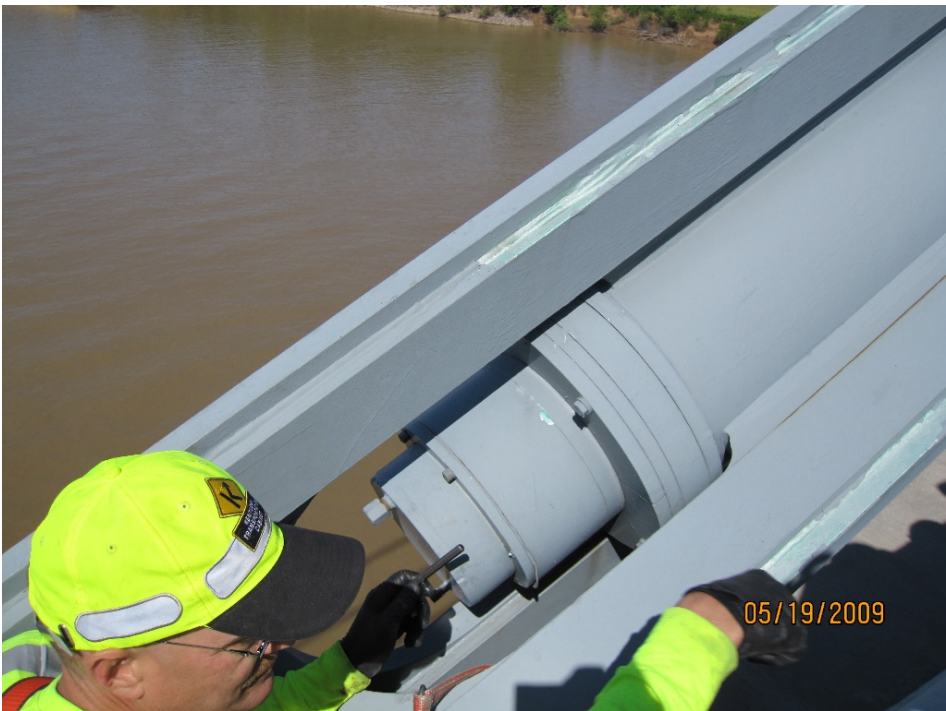
Figure 9. Protective Cap on Deck Anchorage during Removal.
