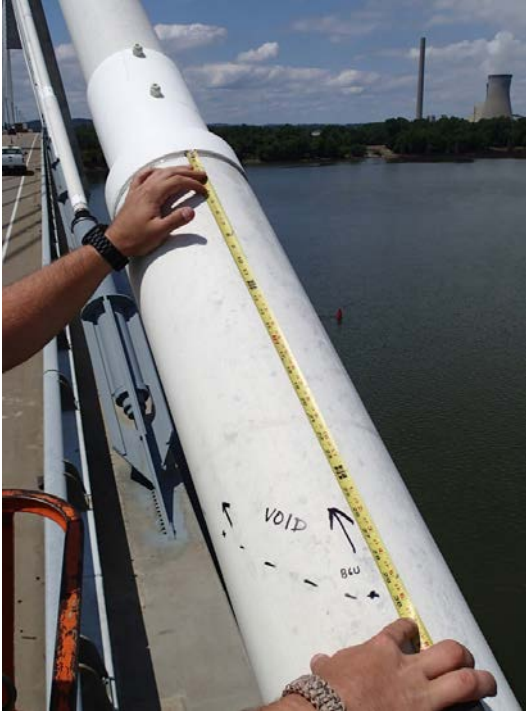
Figure 24. Measuring Grout Voids Based upon GPR and Sounding Tests.
