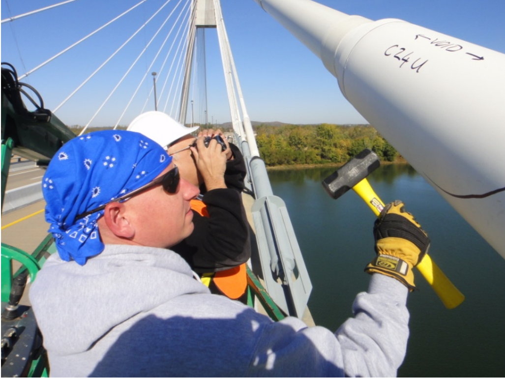
Figure 16. Locating Voids in Deck Anchorage Piping Using Sounding (October 2010).
