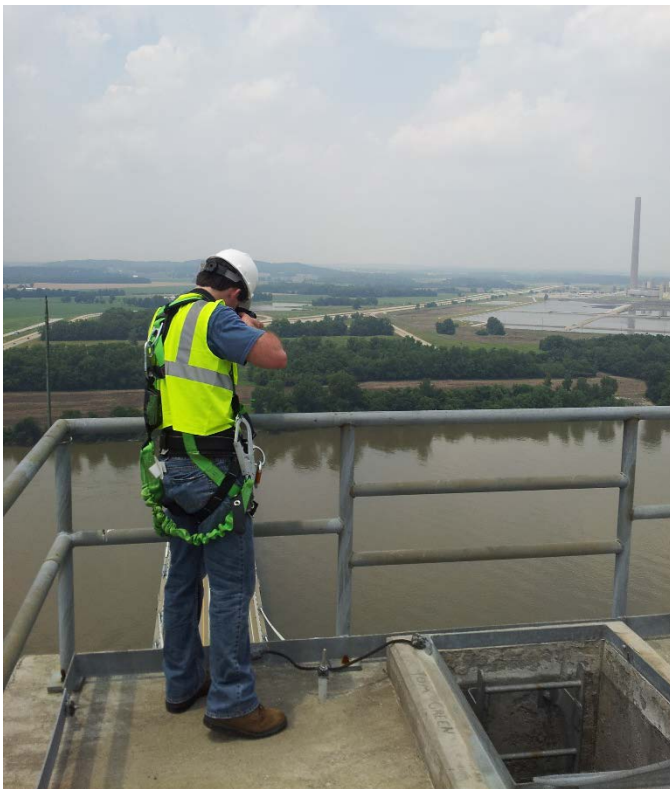
Figure 27. Camera Operator Taking Thermal Images of Anchorages at the Tower Decks.
