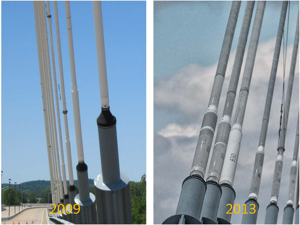
Figure 73. Contrasting Appearance of the Stay Cable HDPE Piping between 2009 and 2013.
