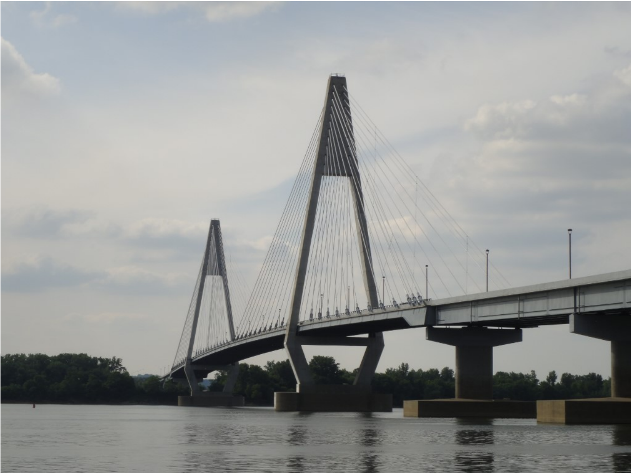
Figure 1. US 231 William H. Natcher Bridge over the Ohio River near Owensboro, KY and Rockport, IN.
