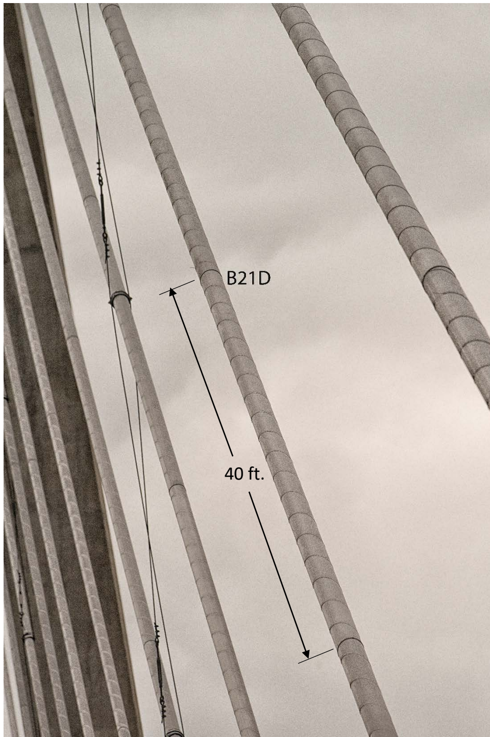
Figure 61. Typical 40 ft. Stay Pipe Segment with Helical Ribbing Intact.
