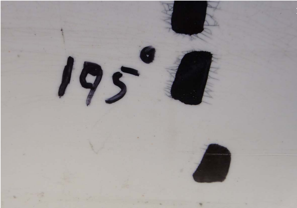
Figure 76. Close up Picture of Ink Marks on the Bottom Side of the Connection Sleeve at B20U Showing Signs of Minor Micro-cracking (Ink Bleeding).
