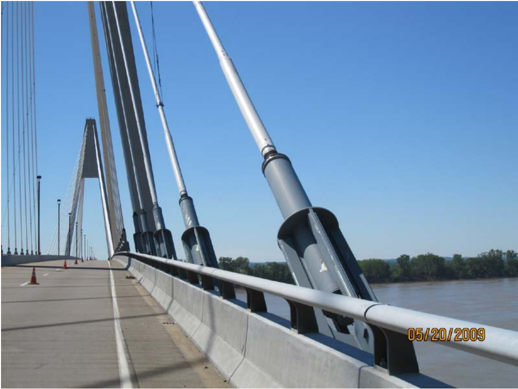
Figure 4. Deck Anchorages.
