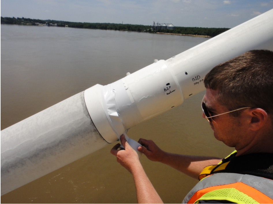
Figure 96. Covering the Stopaq® Paste Seal with Tedlar Tape.
