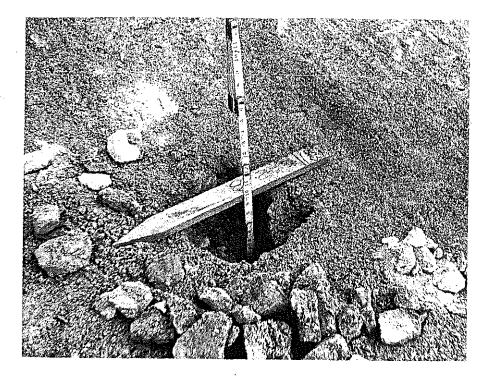
Fig. 7. Near view of a hole excavated in the finished base course. Note the distribution of screenings throughout the entire depth, and the fact that the original ll-inch depth of stone has been reduced to 8 inches in the compacted base.
