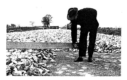
Fig. 2. Coarse stone for the base contained an unusually high percentage of elongated pieces, as can be seen at several points in this photograph. This was not particularly detrimental in the spreading or compaction of the material, and the base was well keyed when final compaction was completed. Note the indicated depth of loose spread.
