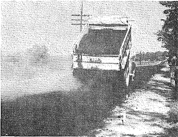
Fig. 13. Distributing by "tailgating", Class I Binder Material on half-width construction.
