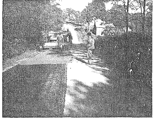
(b) Spreading damp stone (note overlap caused by variable road width).
