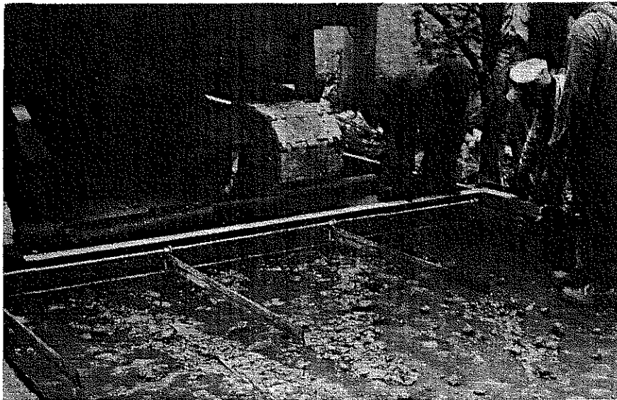
Fig. 18. The apparatus designed to secure the aluminum load transfer device firmly in position during the placement of concrete around the joint. The four members extending parallel to the centerline of the roadway are tong-like devices that grip the horizontal section of the aluminum strip. One arm of each tong is fixed rigidly to the transverse member which spans the forms, and the other arm is pivoted on the first near the free end (a detailed sketch is shown in Fig. 27) and is opened and closed by means of a spring and eccentric mechanism arranged on a rotating circular bar. The circular bar is rotated by a lever and it manipulates the four tongs simultaneously. This apparatus was developed by the company that furnished the joint.
