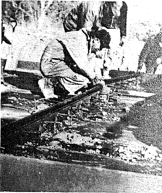
Fig. 2. Installing dowel-bar load transfer joint assembly with neoprene sealers. November, 1948.
