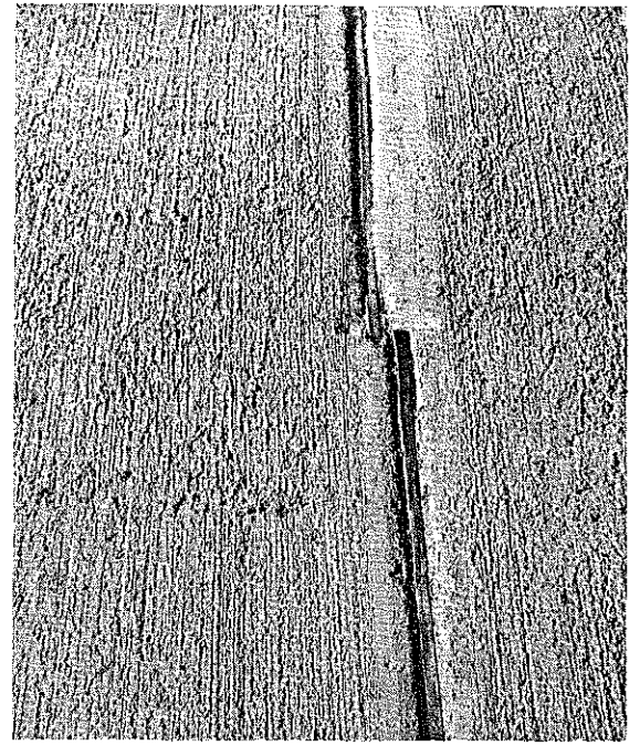
Fig. 3. Closeup of Joint at Sta-622,42 in February, 1949. At the center of the pavement the neoprene sealer did not form a continuous seal.
