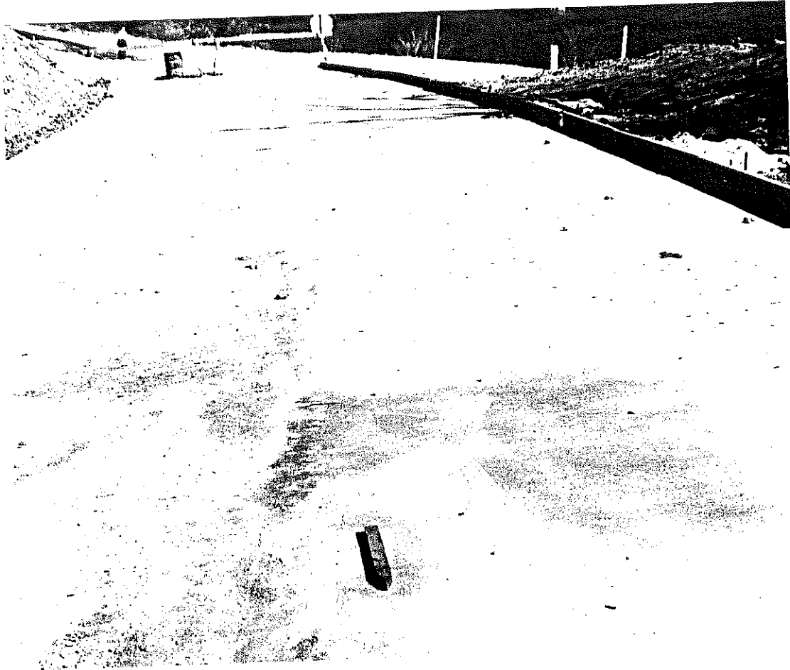
Fig. 6. Finished concrete base on the full-width revision between Sta. 113/77 and Sta. 124/11, about three weeks after placement. At that time only two cracks had developed throughout the 1000-foot section.
