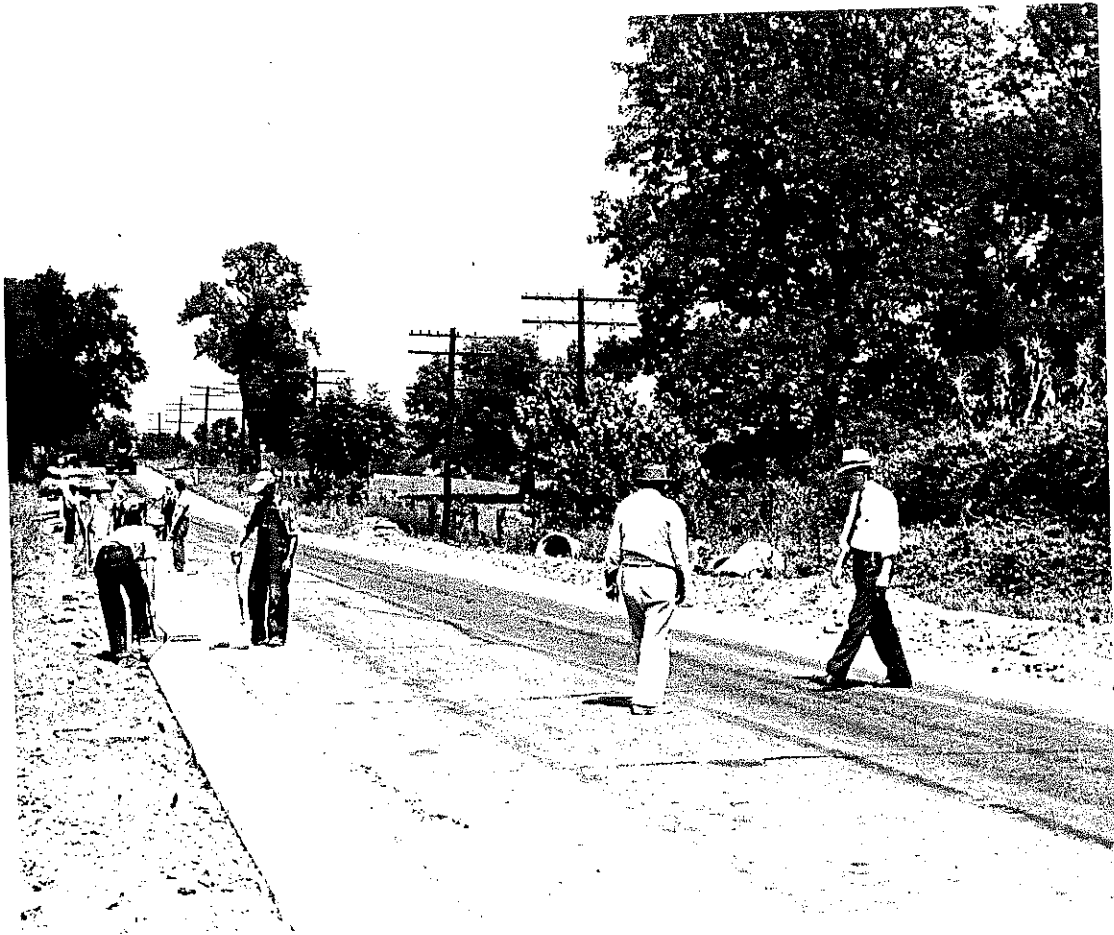
Fig. 1. Mt. Sterling-Winchester Road, U.S. 60, in Montgomery County. The two-foot widening in the foreground was placed on the North side of the old pavement, and contained no contraction joints. On the South side, contraction joints were placed coincident with joints in the existing slab at intervals of 30 feet. The old pavement was built in 1924, and had a 6-8-6-inch section.
