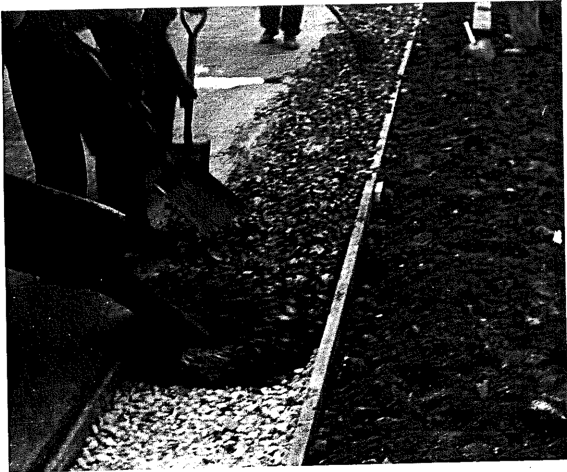
Fig. 2. Placing the lean concrete mix in the widening strip. Note the wooden forms, and the 2-inch stone insulation course beneath the pavement grade. Concrete for both the widening strips and the revisions was delivered by transit mixers from Mt. Sterling. A hand-drawn vibrating screed was used to strike off the surface in the widening strips.
