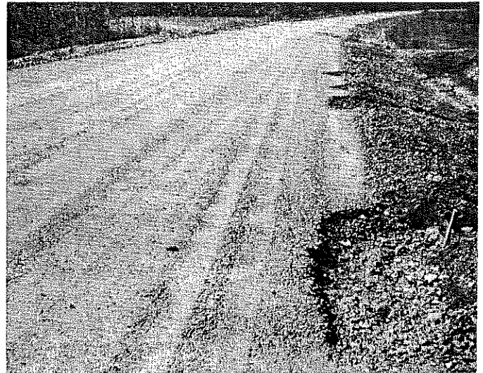
Fig. 16. Erosion of bank gravel base and shoulders following the heavy rainfall of August 28. Only the top 2 inches of base had been treated at the time, and water removed both treated and untreated material as shown. Eroded places were refilled with stabilized gravel and recompacted.
