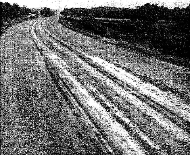
Fig. 17. A section of completed base following a rainfall of 2.40 inches within the preceding 77 hours (September, 10-13). This portion of the base had cured for one week before the heavy rain occurred. There was only slight evidence of softening of the base at this point, although a considerable amount of traffic to and from the Cumberland River Bridge project passed over this base during and following the rain.
