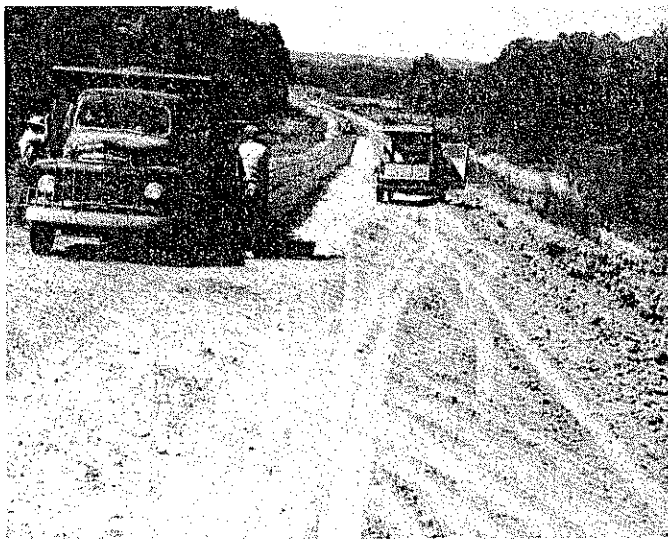
Fig. 7. Placing selected bank-run gravel uniformly with a mechanical spreader. Binder soil to be mixed with the gravel was spread in the right lane prior to the placing of the gravel.
