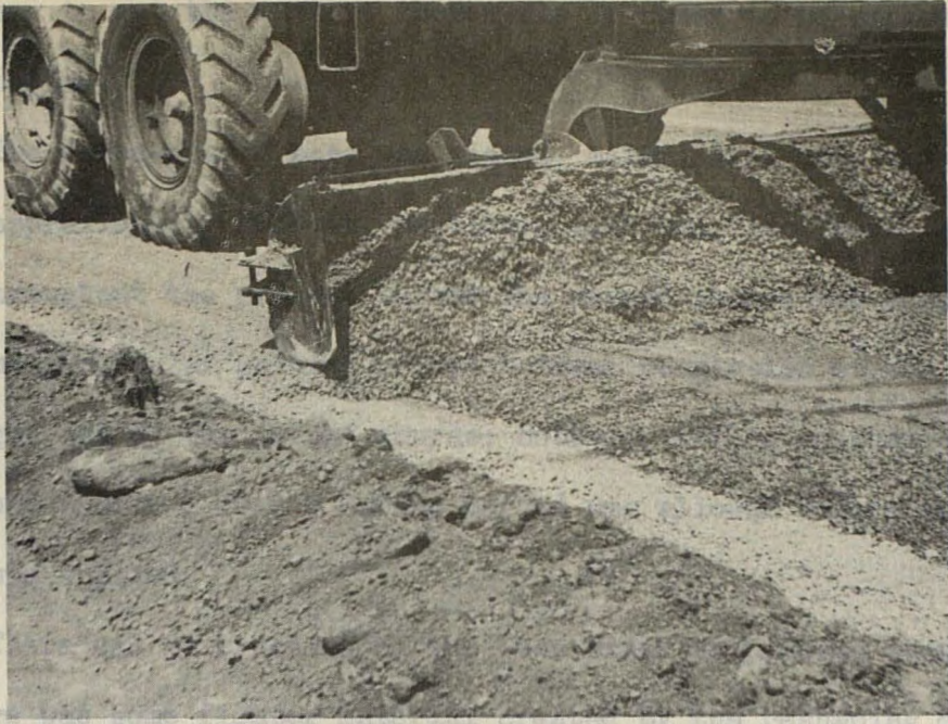
Fig. 9. Placing the edge of the dense-graded base with an edge board that was attached to the blade for the last few passes in the layingout process. This attachment could be easily removed or replaced. A very neat and uniform edge was obtained in this manner.
