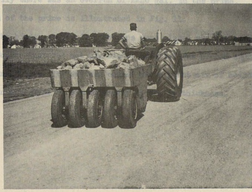
Fig. 10. Pneumatic Rolling. This operation was begun during the final shaping of the blade-spread base.
