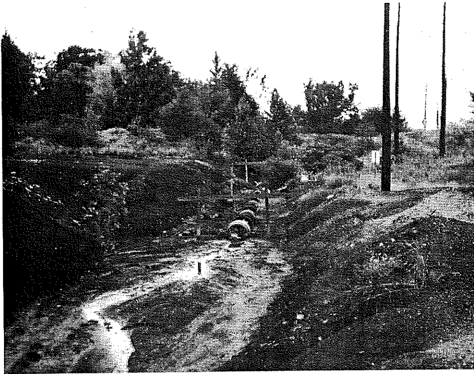
Fig. 13 - Test installation at Mortons Gap
