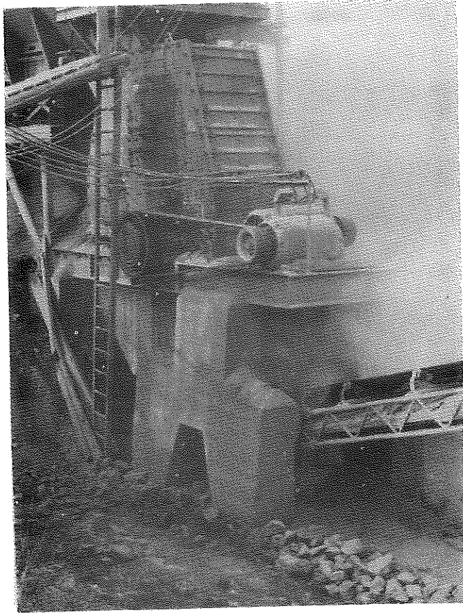
Fig. 1 - Primary crusher in operation. This unit produced 2000 to 2900 tons of stone per day through a 2-in. screen. Quarry trucks dumped material into a hopper (not shown) just above the crusher.
