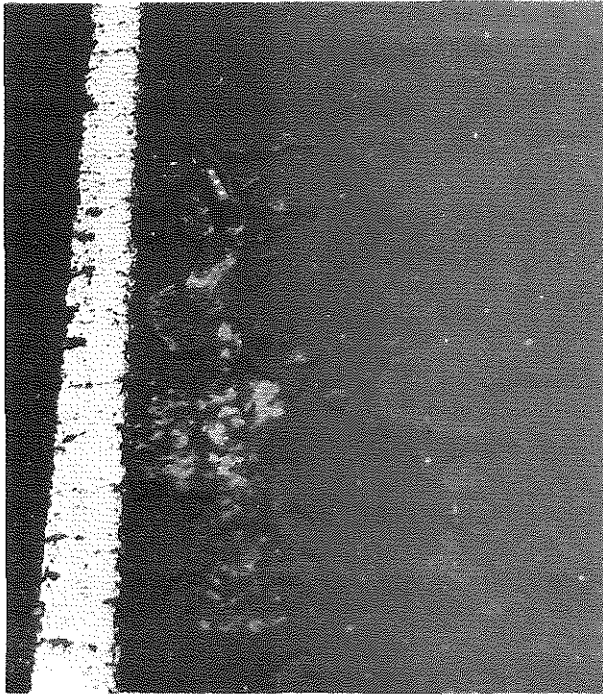
Fig. 7 - U. S. 27, showing two close-up views of an opening in the crust and underlying pockets of stripped sand. Only in a few places was it possible to insert a blade in this manner.
