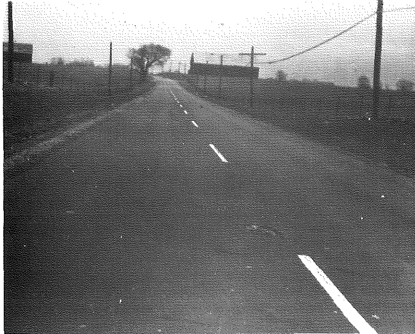
Fig. 1 - U. S. 421 near Midway showing where entrance was made through the crust with a thin blade, crust was easily lifted up revealing small sand pockets between the loosened crust and the lower layer. A scaled section in the wheel track of the left lane is visible, and in the foreground there are indications of wrinkling and shoving.
