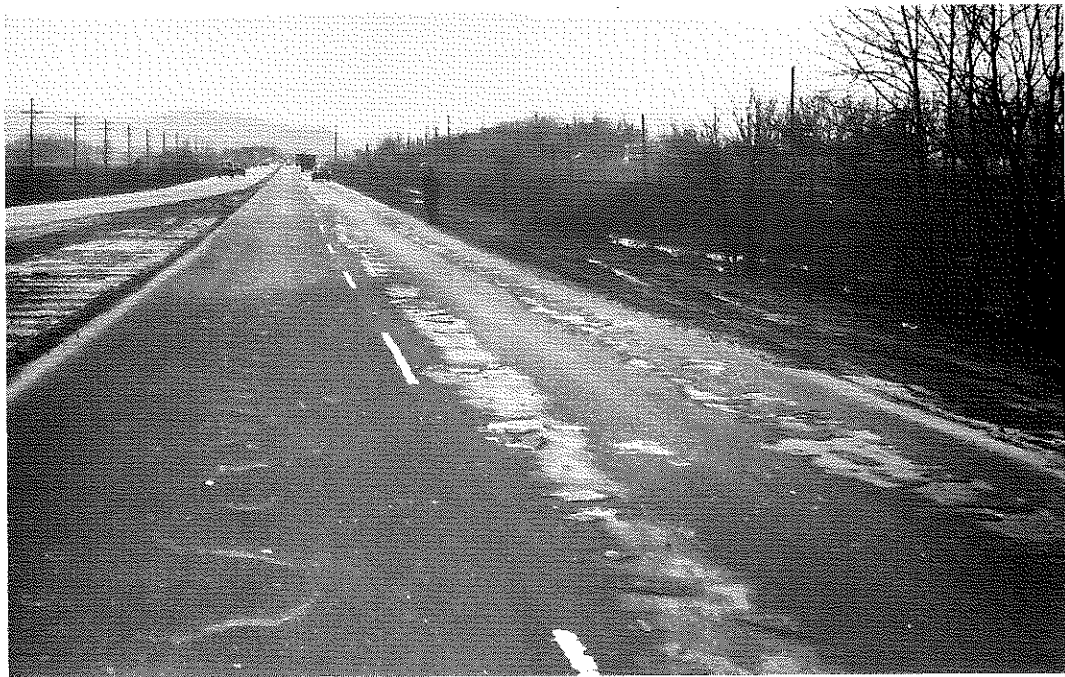
FIG. 51: Section I, Control C, Southbound Lanes: A General View Showing Scaling and Sanding of Overlay Patch. Failure extends only to original surface, which was apparently strengthened and toughened by priming material. Note that inside lanes are still undamaged.
