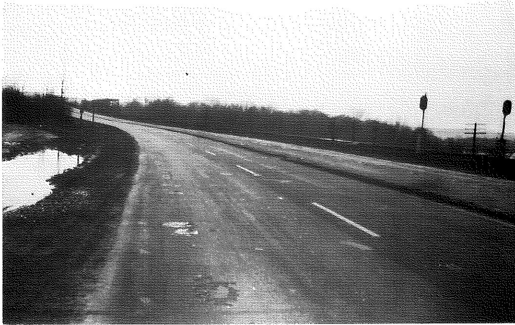
FIG. 58: Section V, 2 Percent PAC-3 added, Dry Heated, Northbound Lanes. Some scaling is evident in outside wheel tracks. Scale is very thin, and affected locations do not appear to be associated with any factor apparent at the time of construction.
