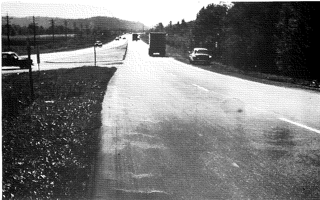
FIG. 28: Section I, Control B: Example of Streaks Caused by the Scouring Action of the Paver Screed Tending to Strip Asphalt from the Sand. The asphalt accumulated on the screed and was sloughed off at intervals, leaving alternately enriched and stripped sand on the surface. This condition was minimized when the screed was hot.
