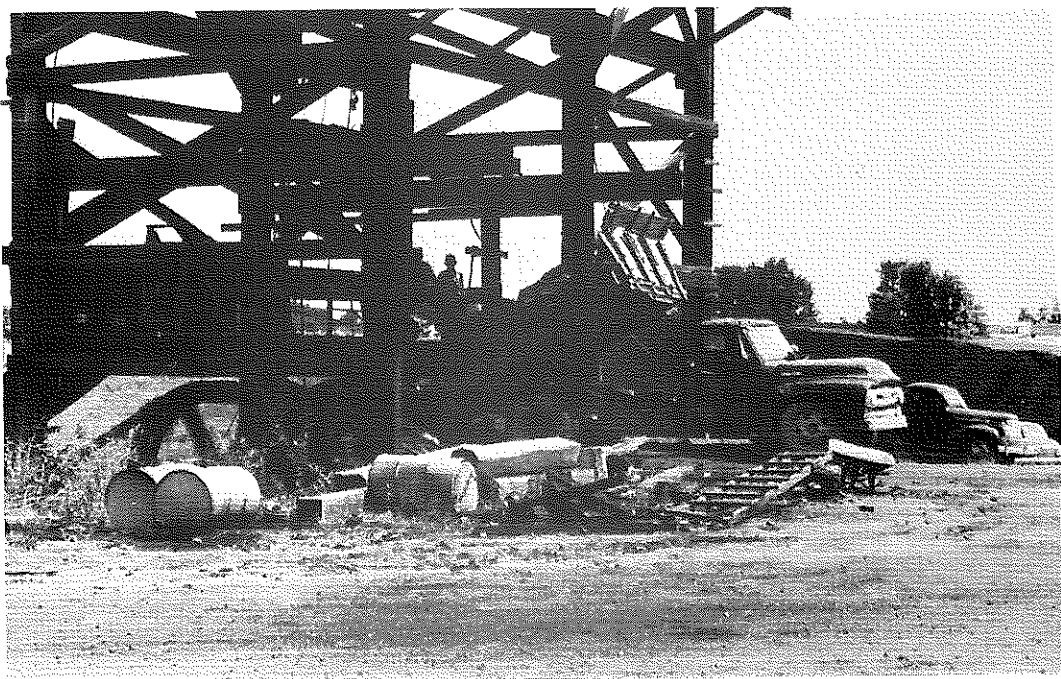
FIG. 11: Delivering Asphalt Rock from the Quarry to the Primary Crusher.
