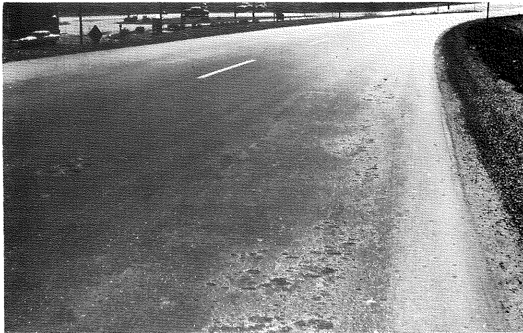
FIG. 34: Section I, Control B. Same section after resurfacing with a thin overlay spread with the paver, and after about two months of service.
