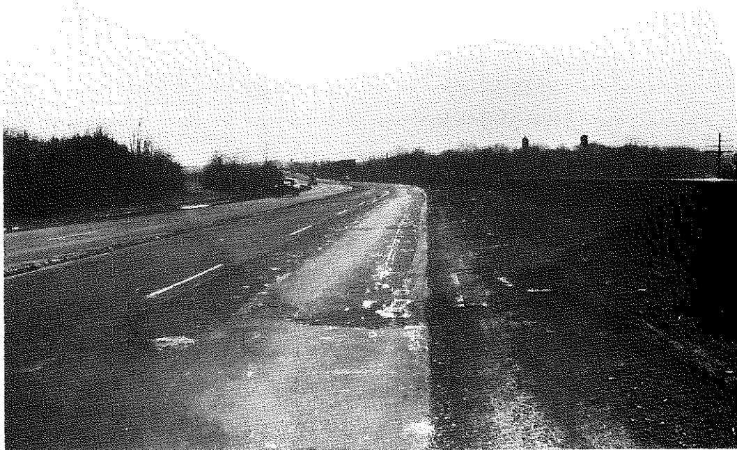
FIG. 56: Unscheduled Section Containing Powdered Asphalt No. 2 Similar to Section III Near West Point, Sta. 107+08 to 115+66. This section was seriously affected by oil from a broken hydraulic cylinder on the paver. Rutting occurred in the wheel tracks almost immediately. These were cut out and replaced in October, 1955. Patches are practically intact but failure continues around them.
