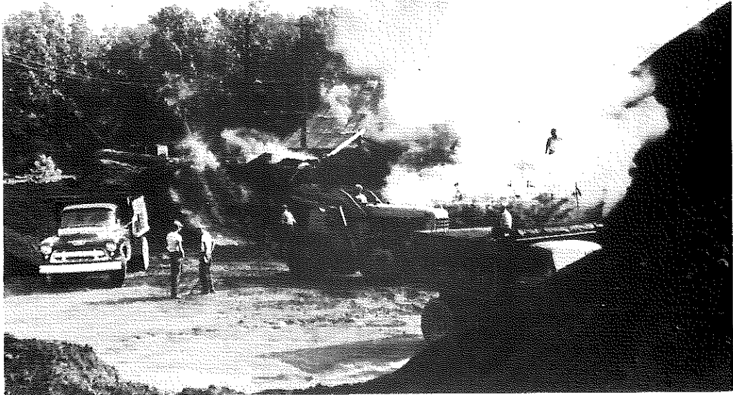
FIG. 12: Steaming and Loading Rock Asphalt at the Stockpile.
