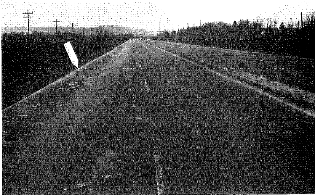
FIG. 50: Section I, Control A, Northbound Lanes. The southern end of the section is shown, with joint at arrow between Control A and section containing Antistrip No. 1. Meandering track down center of outside lane was caused by heater-planer in reworking, during October. Obviously, attempts were unsuccessful in effecting permanent restoration. Traffic tends to avoid these areas because of roughness.
