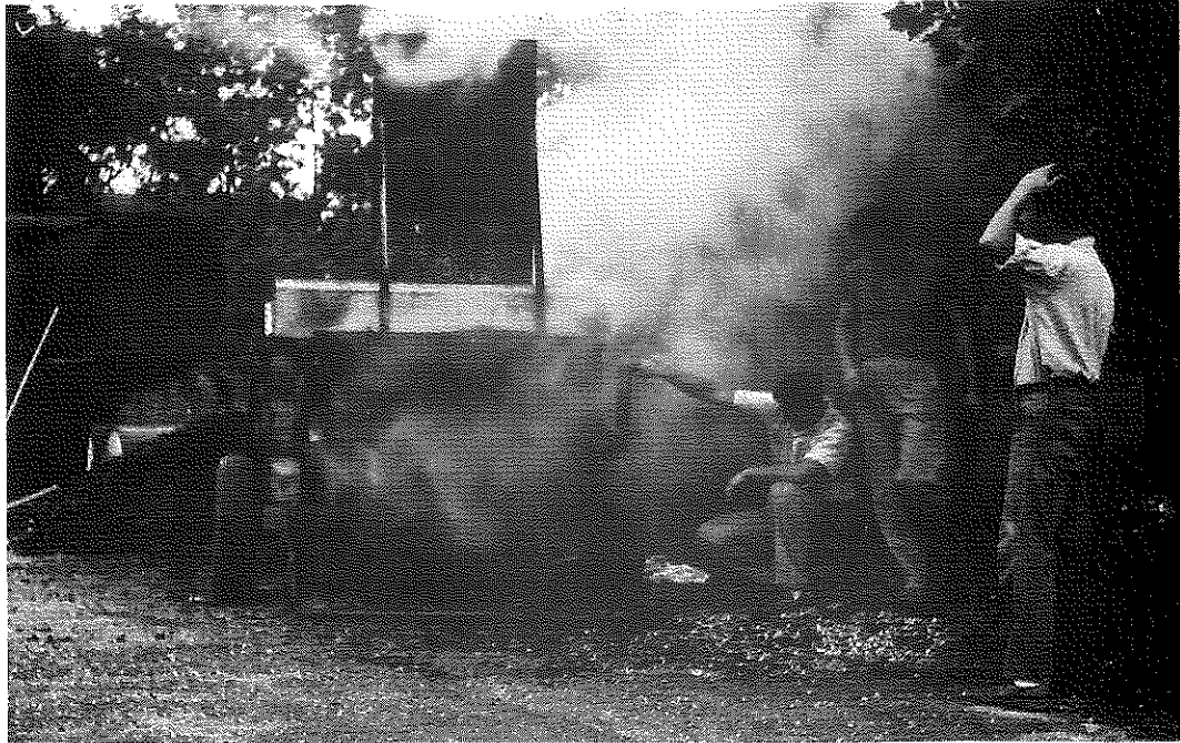
FIG. 21: HTB Mixer Heating Rock Asphalt in Trial Runs.
