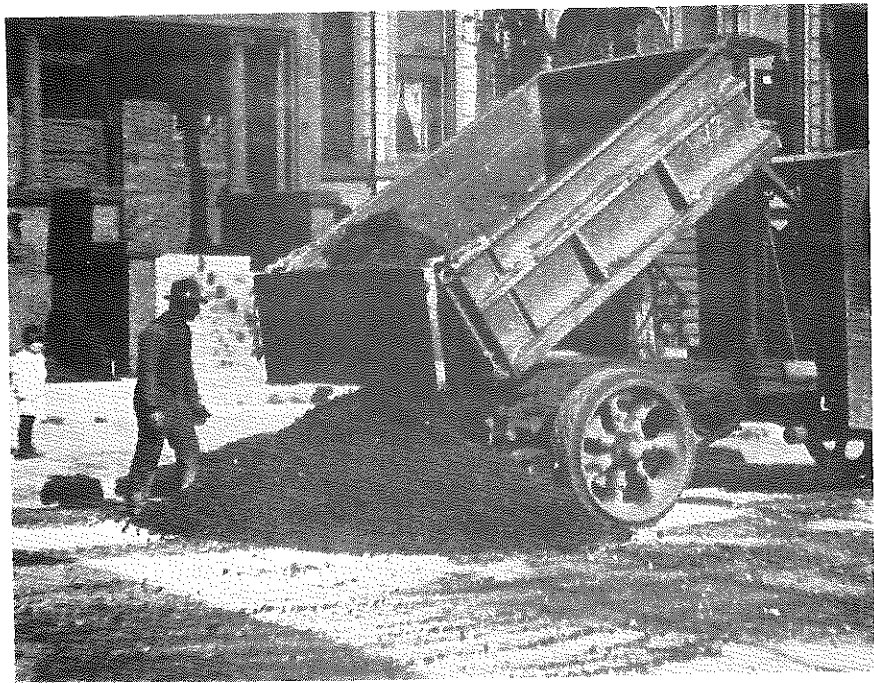
Fig. I-b: Dumping Rock Asphalt for Hand Spreading: 14th Street in Chicago, about 1920.
