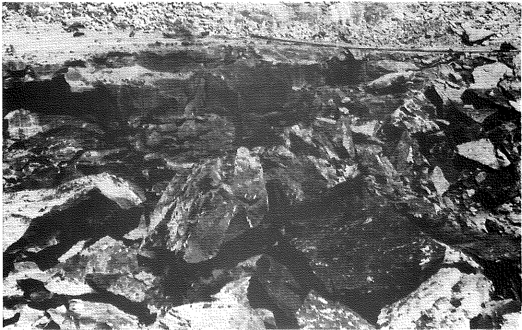
FIG. 7: Close-up View of Freshly Blasted Rock. Pipe is lying on top of the usable ledge.
