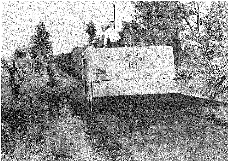
Fig. 21: Ballard Co.: Pneumatic Roller Making First Pass After Final Blending. Following compaction, the base was bladed smooth and finished with a steel flat-wheel roller. (10-12-56)
