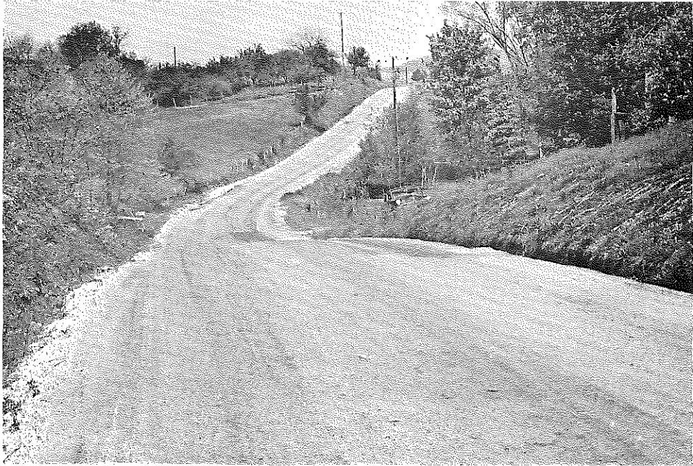
Fig. 46: Wayne Co.: Typical Section after 7 Months. Note patching. (4-24-57)
