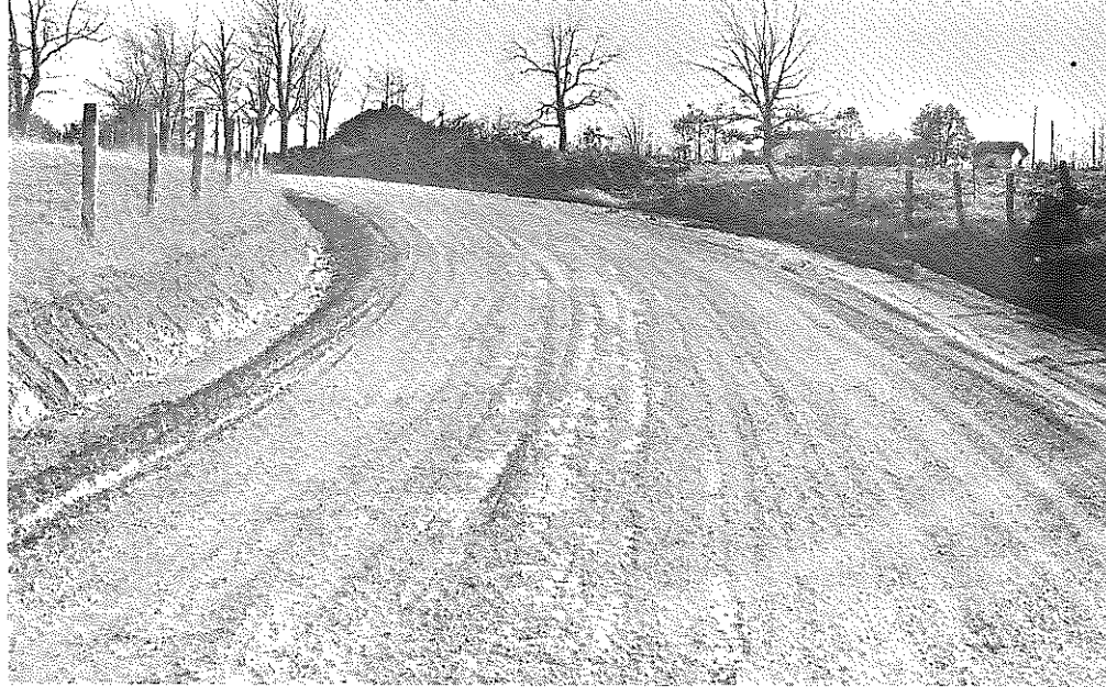
Fig. 10: Breckinridge Co.: Failure of Seal. Soil cement should probably have been primed with diluted emulsion and cured before applying seal. (1-3-57)
