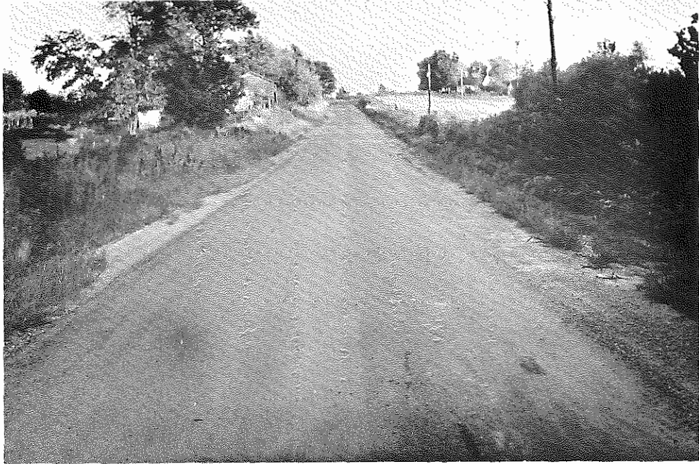
Fig. 16: Webster Co.: Soil-Cement Section after 10 Months. (8-4-57)
