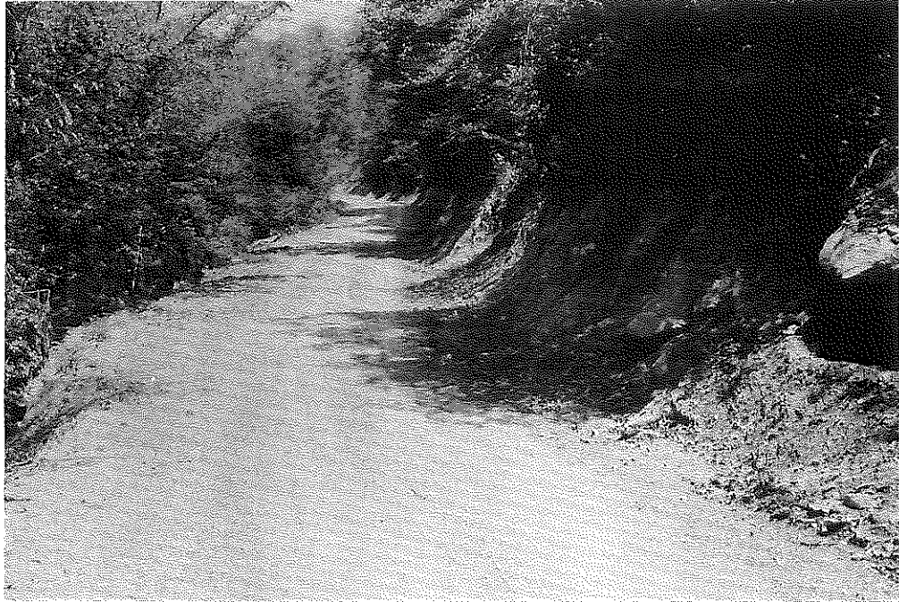
Fig. 70: Lawrence Co.: Narrow Section along Creek Bluff, Badly Eroded. (5-2-57)
