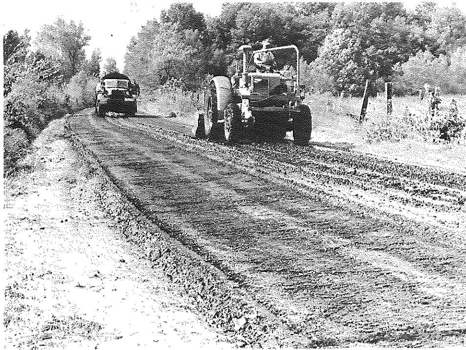
Fig. 20: Ballard Co.: Traveling Mixer, Designed to Spray the Proper Amount of Asphalt Directly from Distributor into the Mixing Pug in a Single Pass. Pump was not operating during this project, however, and several passes with the distributor were necessary for application and blending. (10-12-56)
