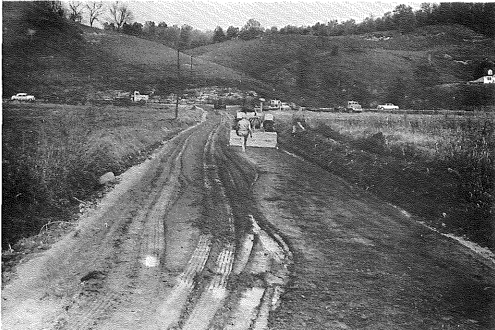
Fig. 64: Lawrence Co.: Soil-Cement, Single Seal. Section was narrow, with bedrock outcropping through subgrade on hill in foreground. (10-24-56)
