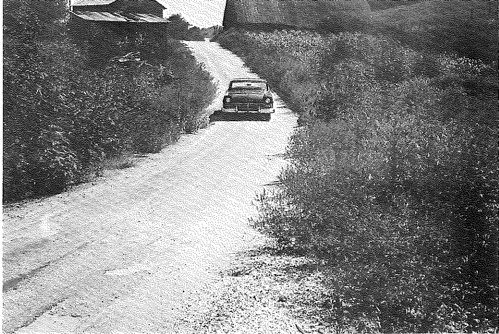
Fig. 74: Lawrence Co.: Narrow Fill and Loss of Seal Coat. Base here is in very good condition. (8-20-57)
