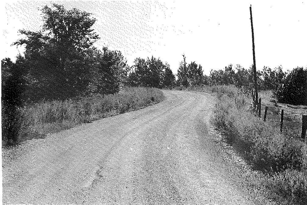
Fig. 34: Marshall Co.: Same View as Above, after 10 Months. (8-4-57)
