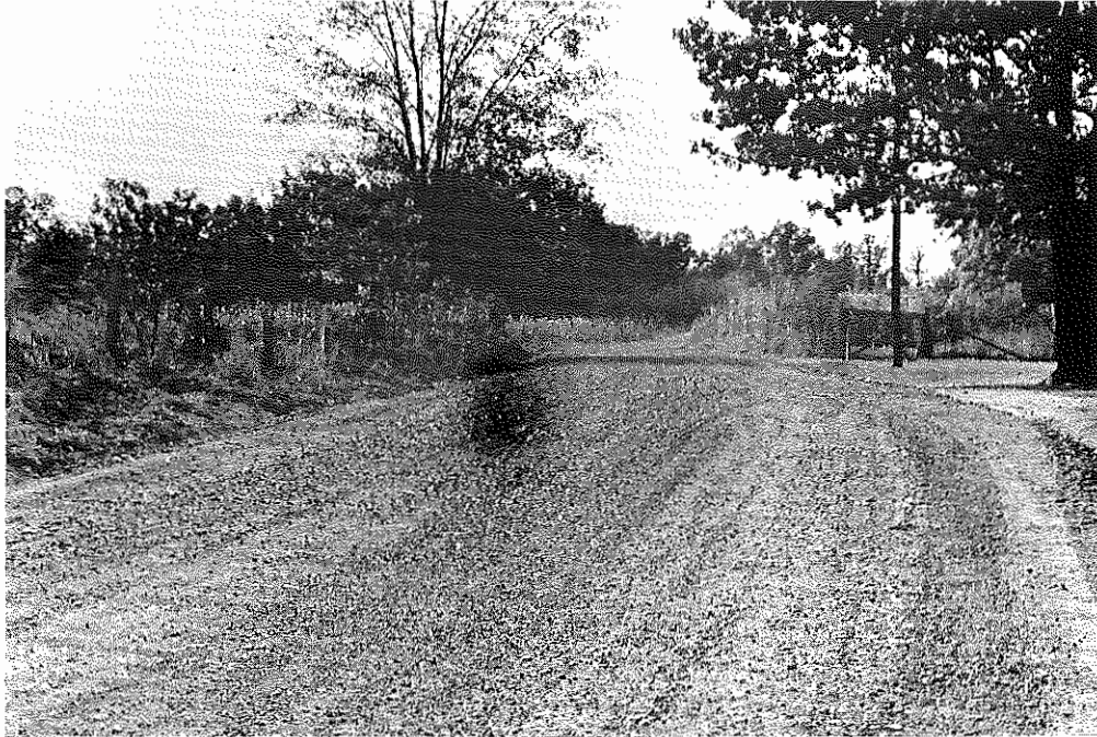
Fig. 29: Marshall Co.: After Stabilizing, before Flat-Wheel Rolling Preparatory to Sealing. (10-18-56)
