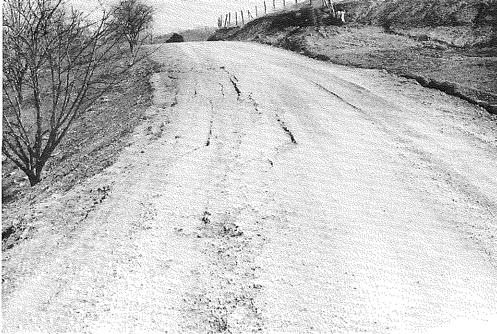
Fig. 66: Lawrence Co.: Showing Unstable Fill near Middle of Project, after 6 Months. (3-13-57)
