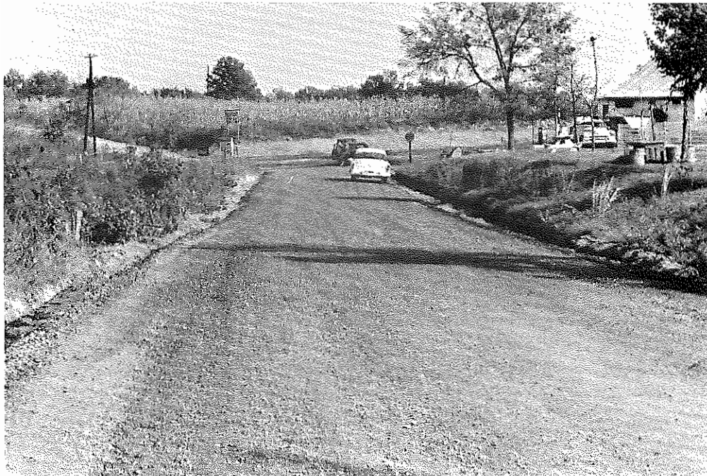
Fig. 29: Marshall Co.: After Stabilizing, before Flat-Wheel Rolling Preparatory to Sealing. (10-18-56)
