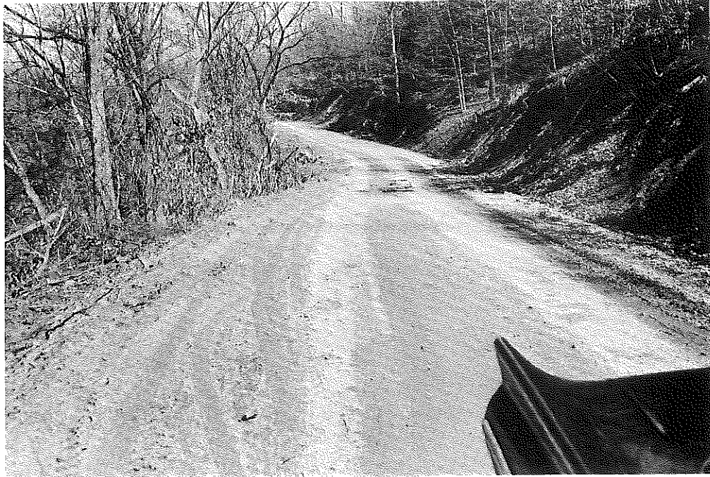
Fig. 68: Lawrence Co.: Similar Section, after 6 Months. Note back slopes sliding onto roadway. (3-13-57)
