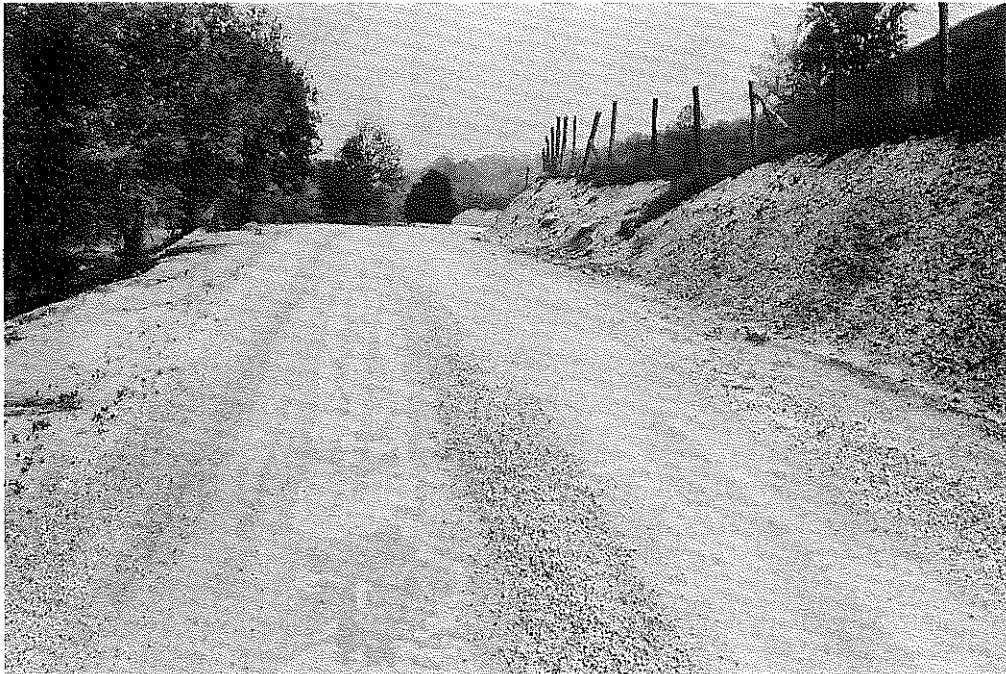
Fig. 70: Lawrence Co.: Narrow Section along Creek Bluff, Badly Eroded. (5-2-57)
