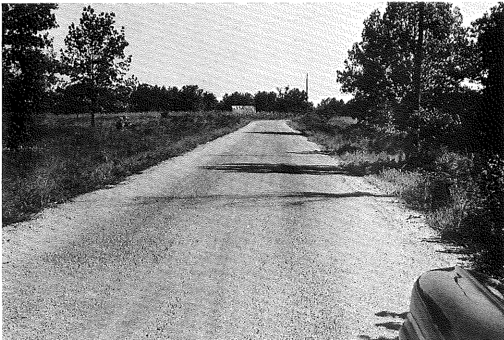
Fig. 36: Marshall Co.: Middle Section of Project after 10 Months. (8-4-57)
