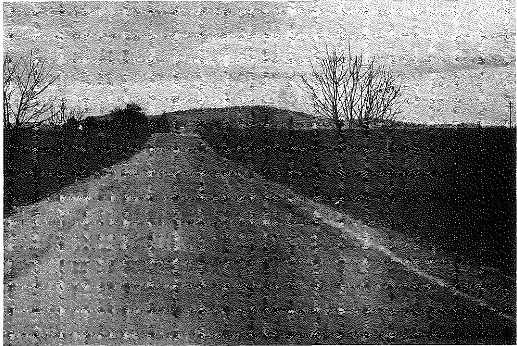
Fig. 44: Wayne Co.: Typical Section after 2-1/2 Months. Granular stabilized soil, \text{CaCl}_2 , double seal. (1-3-57)
