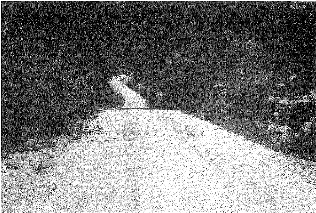
Fig. 74: Lawrence Co.: Narrow Fill and Loss of Seal Coat. Base here is in very good condition. (8-20-57)
