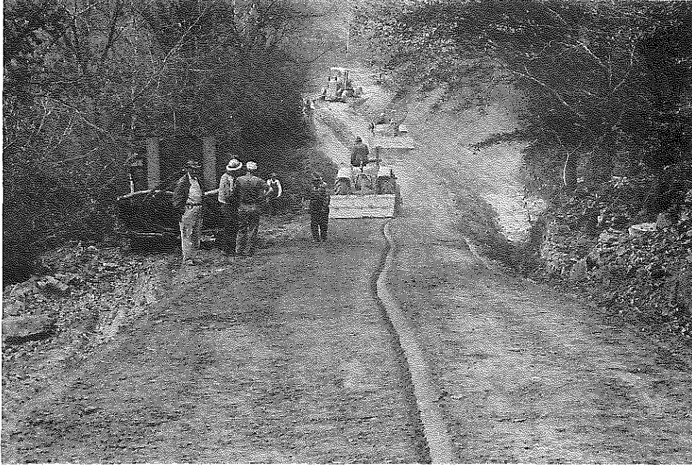
Fig. 64: Lawrence Co.: Soil-Cement, Single Seal. Section was narrow, with bedrock outcropping through subgrade on hill in foreground. (10-24-56)
