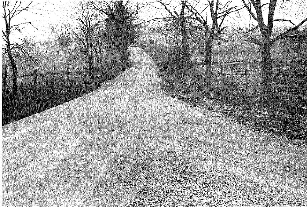
Fig. 56: Montgomery Co.: Granular Stabilization, Single Seal, after 6 Months. (3-13-57)
