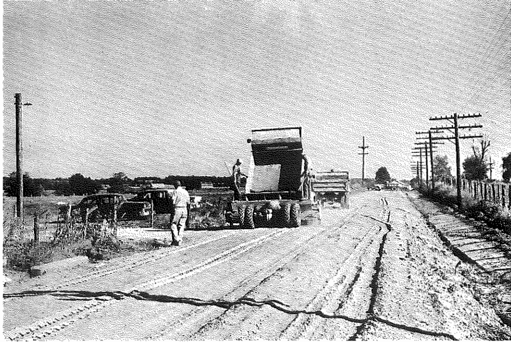
Fig. 4: Breckinridge Co.: Spreading Cement, after Ditching, Grading, and Scarifying. (10-9-56)
