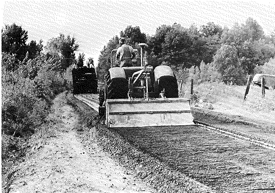
Fig. 18: Ballard Co.: Scarifying ahead of the Traveling Mixer. This facilitated the mixing and blending operation. (10-12-56)
