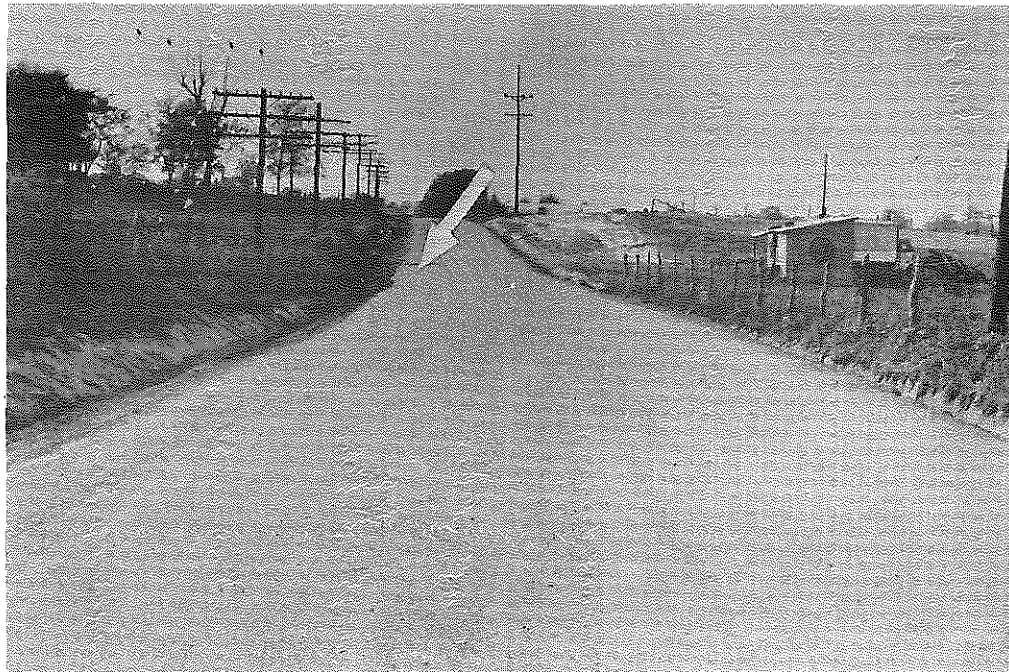
Fig. 6: Breckinridge Co.: Curve at Middle of Project, after Sealing. Arrows point to spots where single seal failed to stick. (10-17-56)
