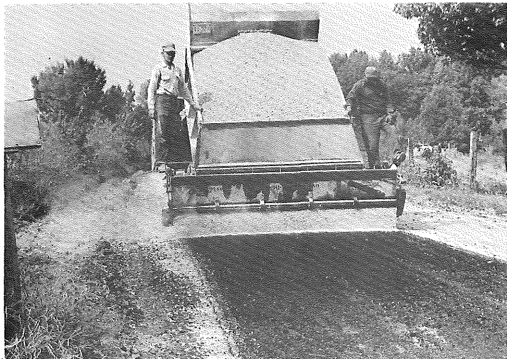
Fig. 23: Ballard Co.: Applying Second Seal. (10-18-56)
