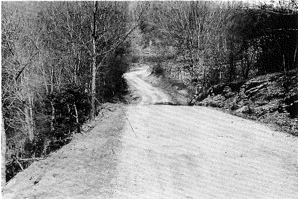
Fig. 66: Lawrence Co.: Showing Unstable Fill near Middle of Project, after 6 Months. (3-13-57)
