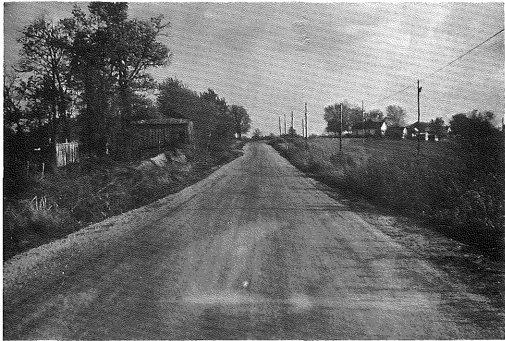
Fig. 14: Webster Co. : Portion of 0.3 mi. Section of Project Where Soil-Cement was Used. The remaining 0.7 mi. was not completed in the time scheduled. (4-24-57)
