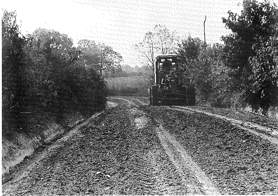
Fig. 18: Ballard Co.: Scarifying ahead of the Traveling Mixer. This facilitated the mixing and blending operation. (10-12-56)
