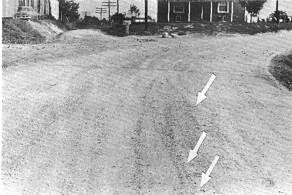
Fig. 6: Breckinridge Co.: Curve at Middle of Project, after Sealing. Arrows point to spots where single seal failed to stick. (10-17-56)
