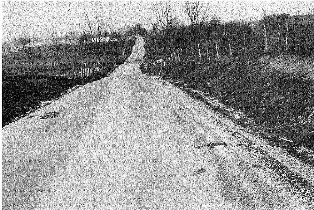
Fig. 56: Montgomery Co.: Granular Stabilization, Single Seal, after 6 Months. (3-13-57)
