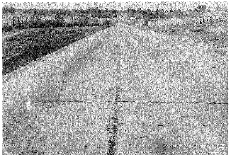
Fig. 11: View to the North in Section 4R.
