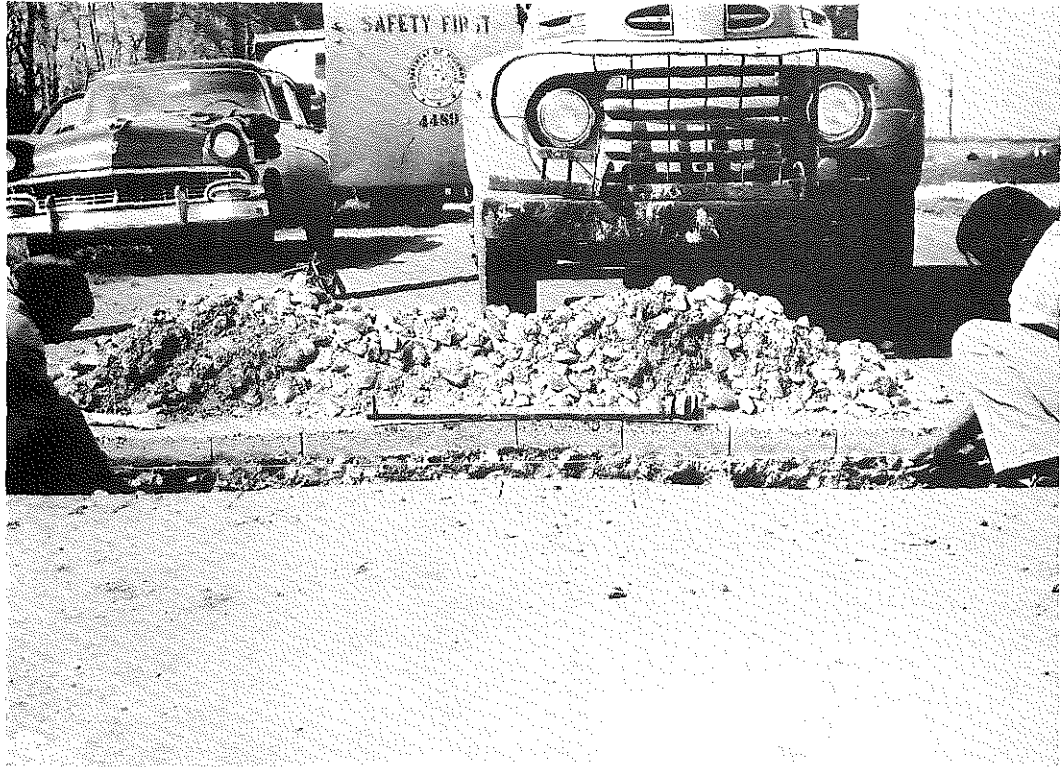
Fig. 18: Photograph Showing Exposed Cross Section of a Rutted Pavement.
