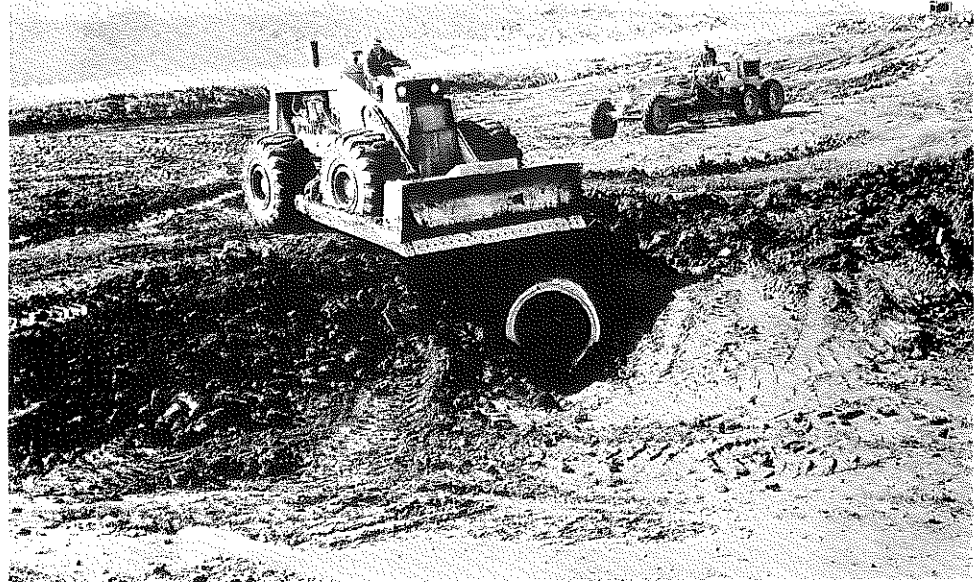
Fig. 20. Placing Backfill before Construction of the Imperfect Trench.
