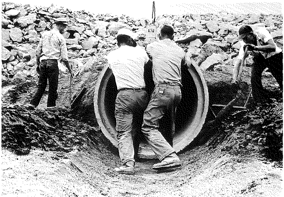
Fig. 19. Placing Pipe in Sand Cushion Bedding.
