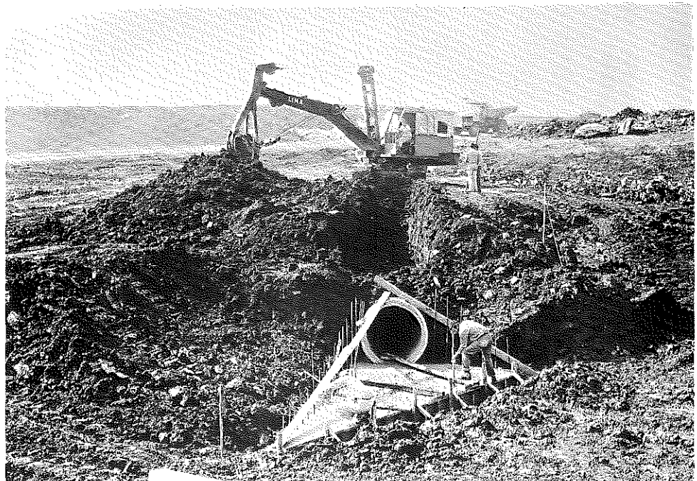
Fig. 21. Construction of the Imperfect Trench.
