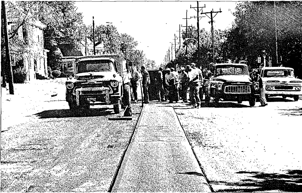
Fig. 6: Euclid Avenue Median. Tests indicated a higher density along the path of the screws -- also evidenced by the finer texture. The surface course has not been placed.
