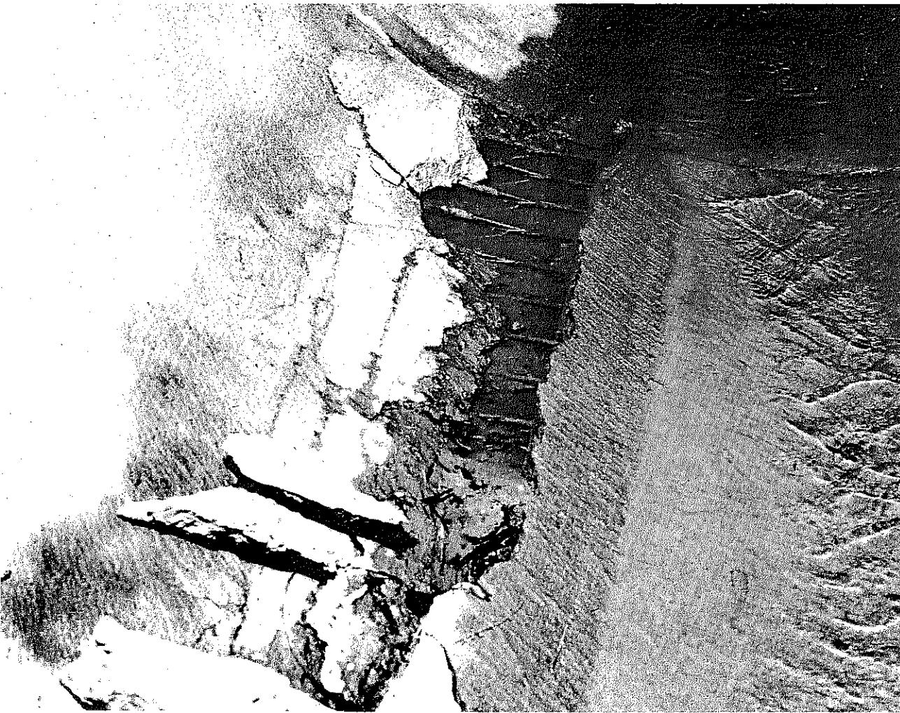
Fig. 1. Failure in Bottom of 60-inch Culvert Under a 28-foot
