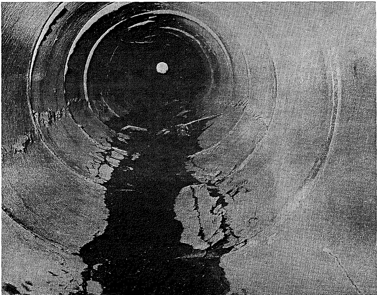
Fig. 5. Failure in Bottom of 54-inch Culvert Under a 53-foot
