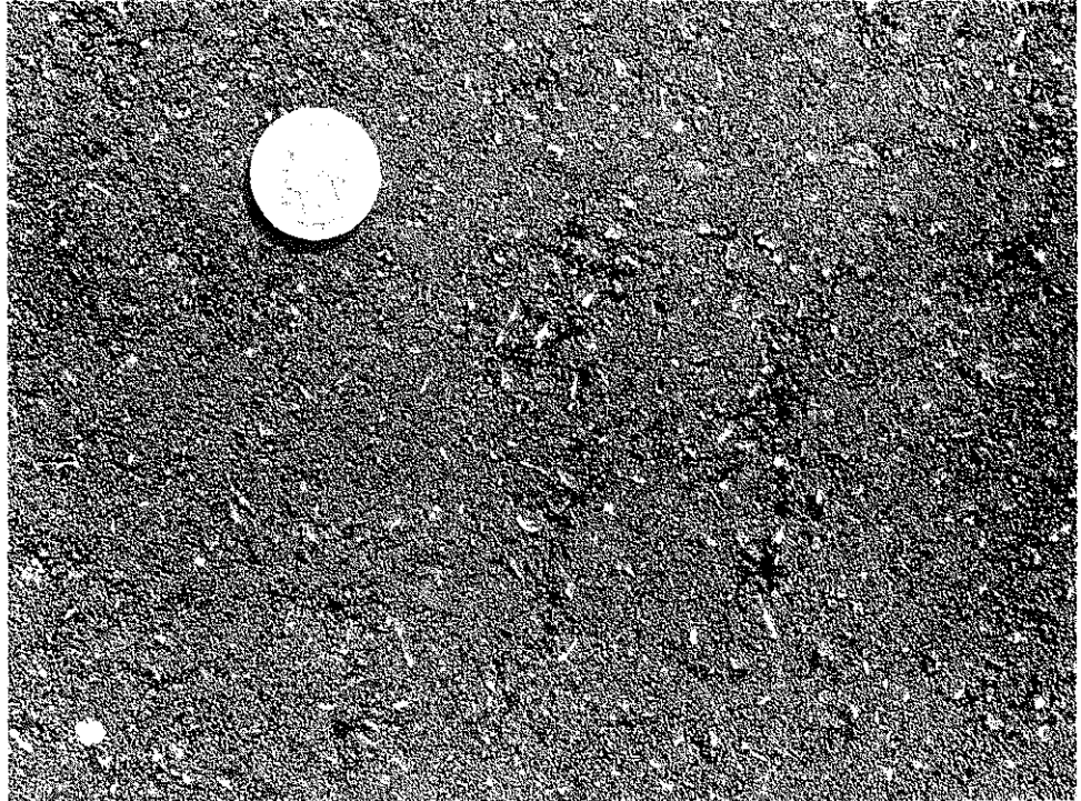
b. After Rolling with Tandem Roller
