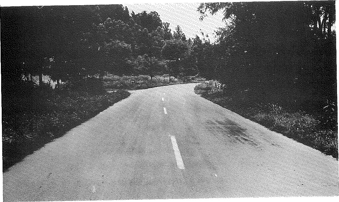
Fig. 1. Ky. 30, Salyersville-Jackson, Constructed with Crushed Sandstone Aggregate in 1951.
