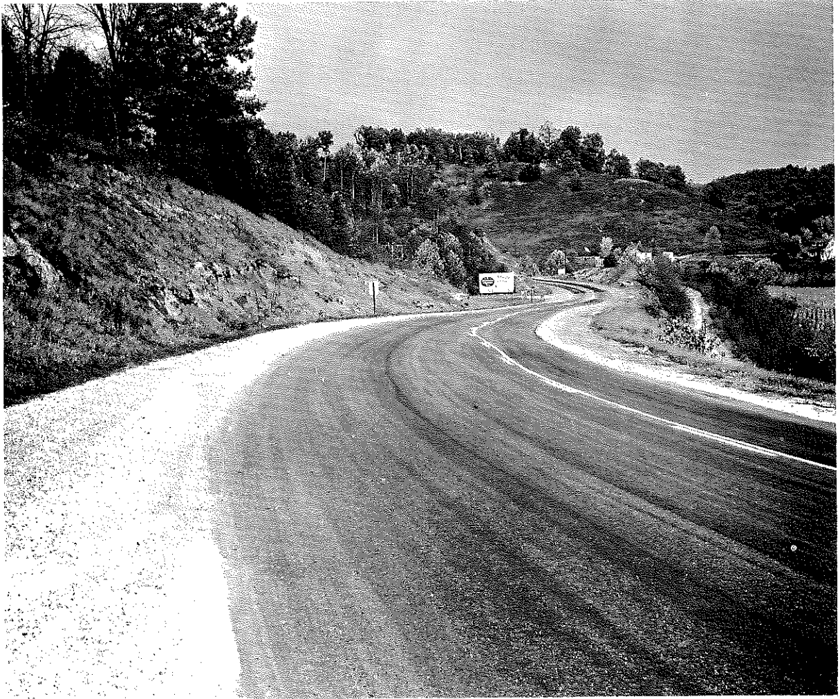
Fig. 8. Conglomerate-Sand Seal, US 25, just North of Livingston, Late December, 1961.
