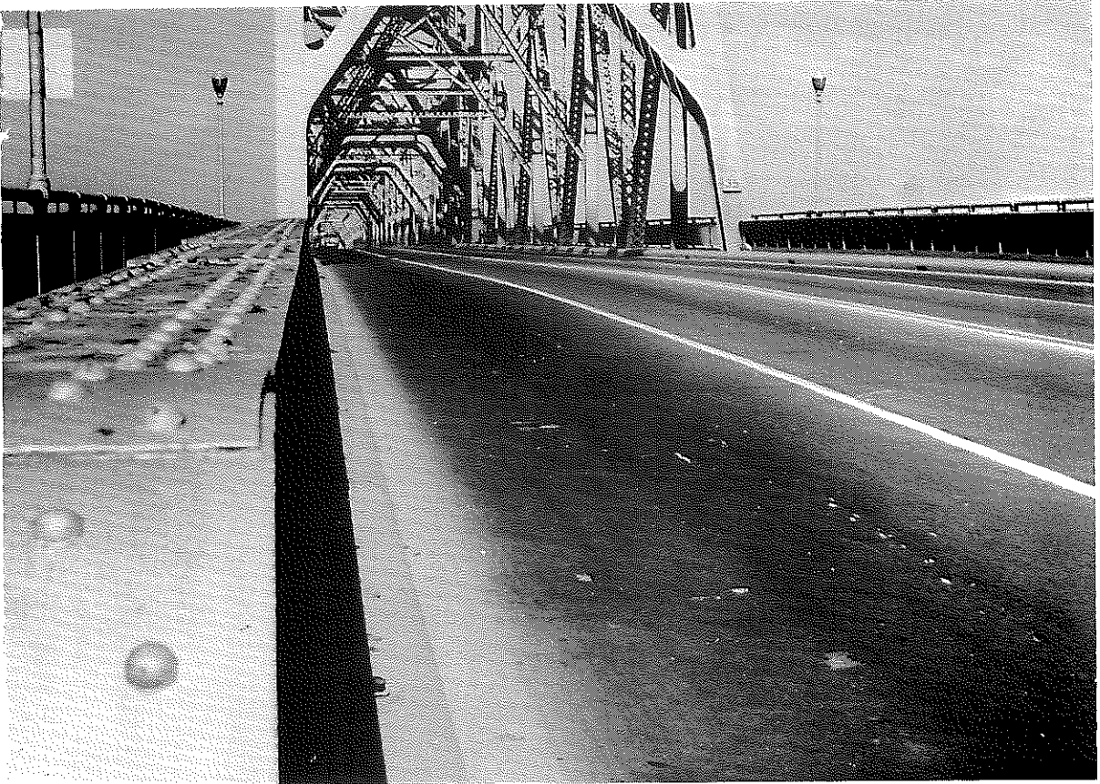
Fig. 7. Clark Memorial Bridge, Louisville; Sand-Asphalt Surface after One Year of Service.
