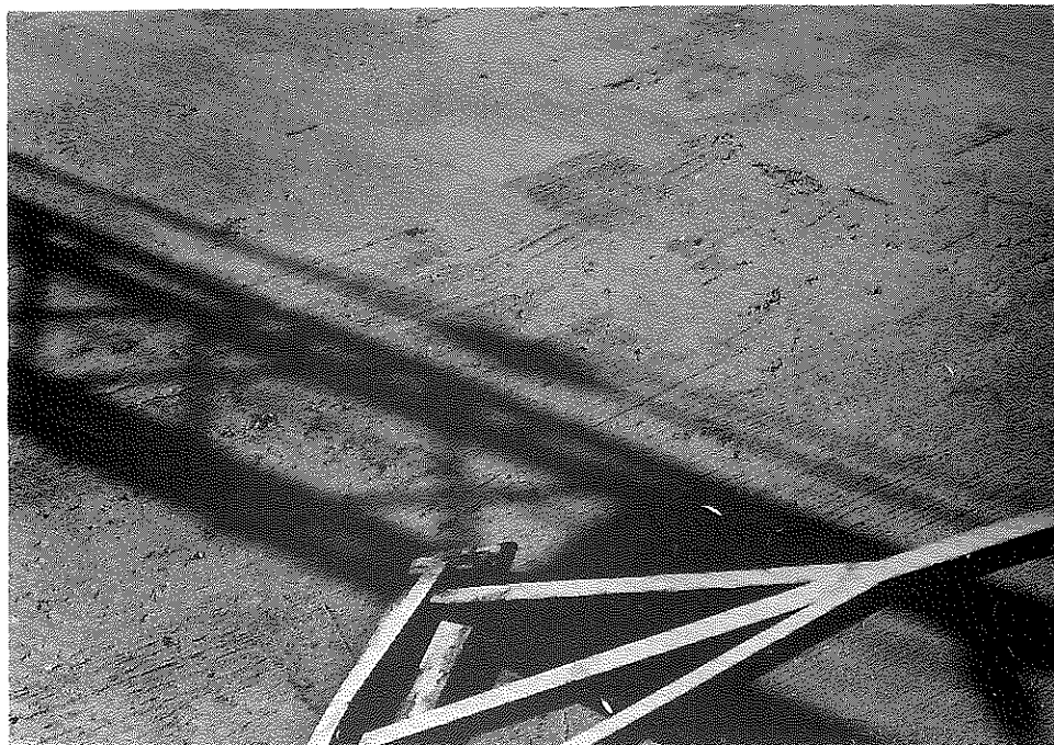
Fig. 9. Openings which could not be closed by floating in one of the ligno sulfonate sections.
