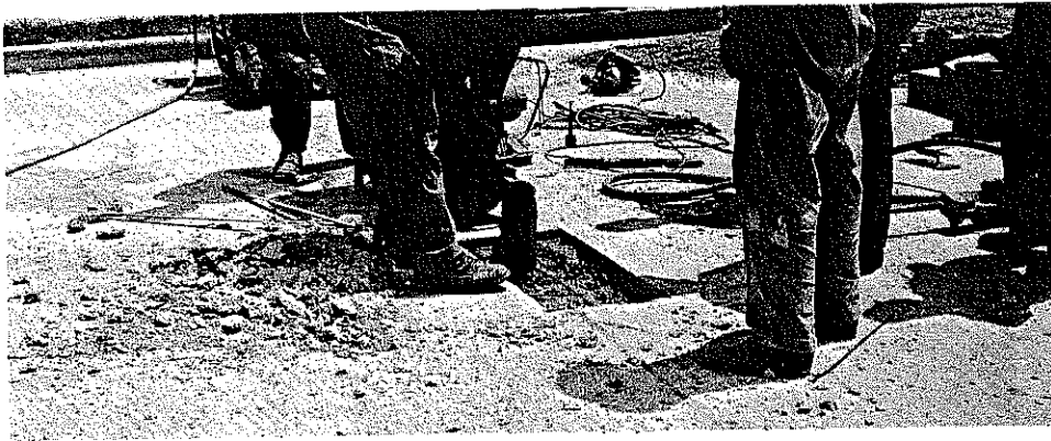
Fig. 2. Station 55 + 75. Hole has been thoroughly cleaned, primed with epoxy, and is receiving the first shovel of "epoxy" patch material, 6-7-62.
