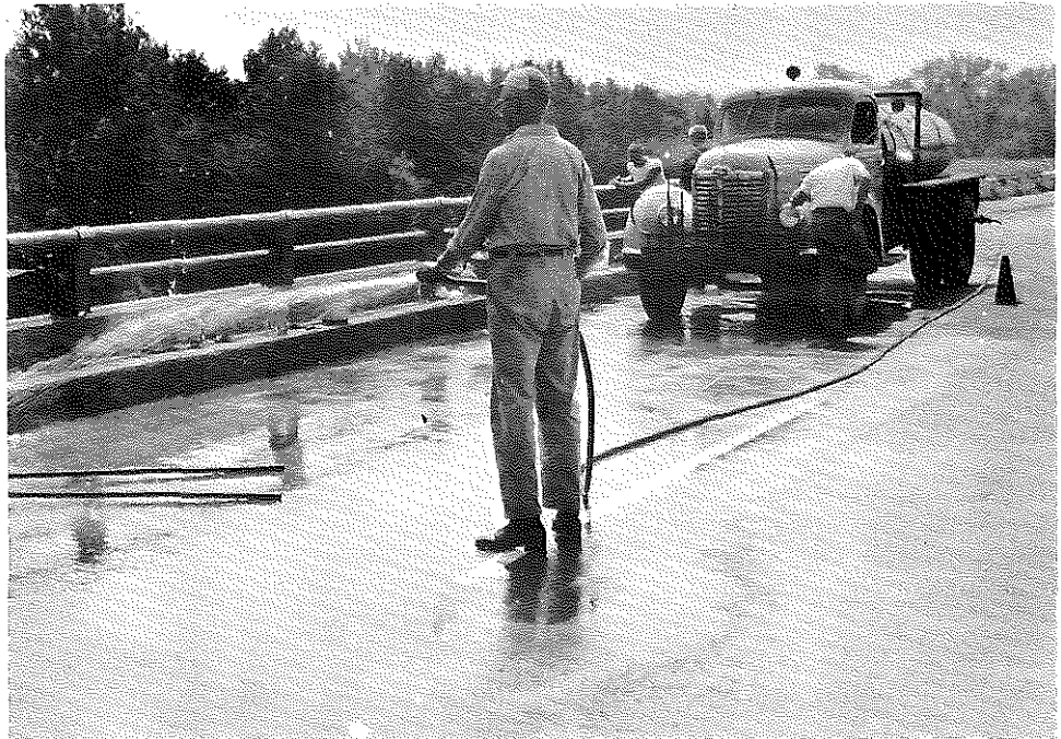
Fig. 71. Salt River Bridge, North-bound, Kentucky Turnpike; Rinsing with Water, After Acid Treatment, August 24-25, 1960.
