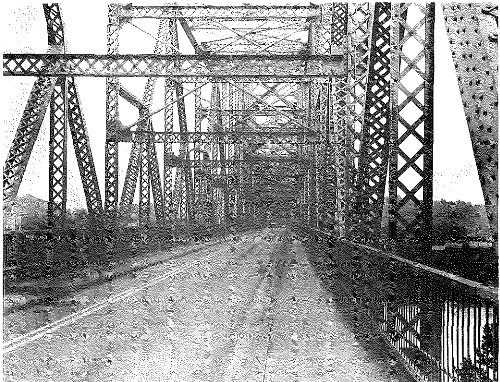
Fig. 32. Ashland-Coal Grove Bridge, Before Surfacing with Sand-Asphalt.
