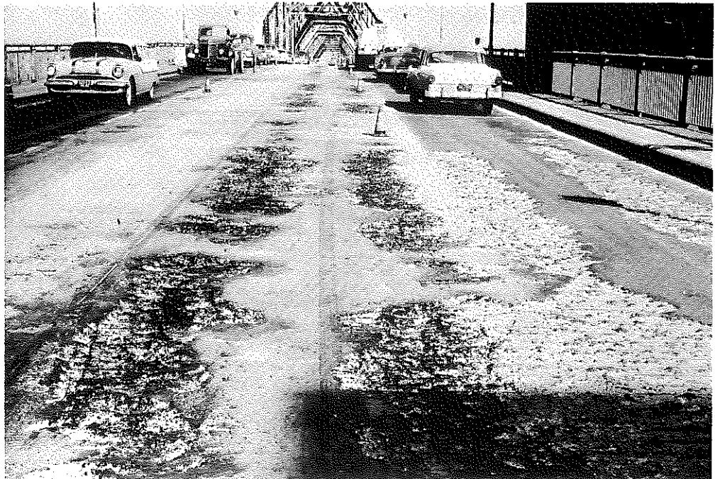
Fig. 20. Clark Memorial Bridge, South Ramp, After Bituminous Patches Removed, October, 1958.
