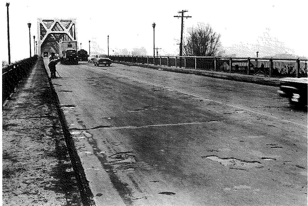
Fig. 24. Clark Memorial Bridge, North Ramp, March, 1960.
