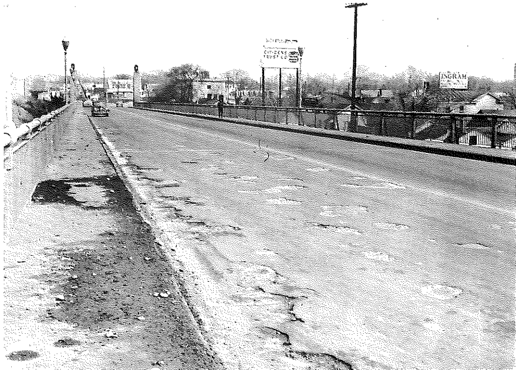
Fig. 23. Clark Memorial Bridge, North Ramp, March, 1960.
