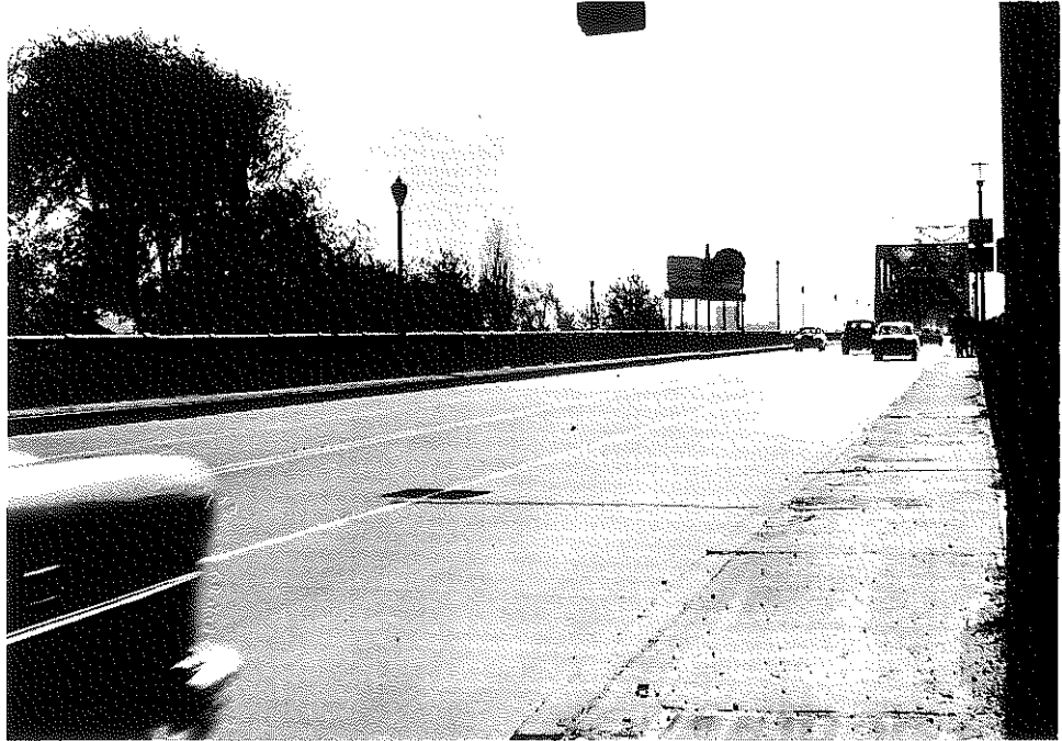
Fig. 21. Clark Memorial Bridge, North Ramp, November, 1959, Sand-Asphalt Surface.
