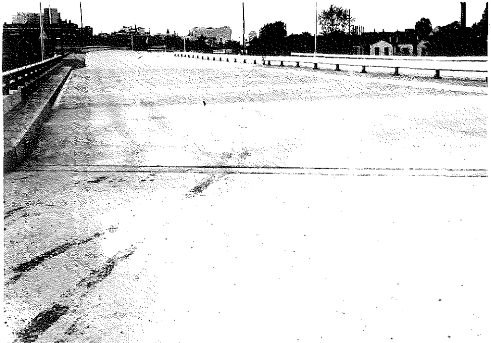
Fig. 38. St. Catherine's Street Bridge, Southbound Lanes, Looking North; Polystyrene Coating in Background.
