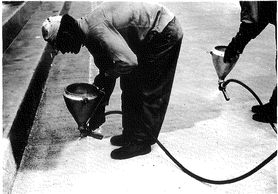
Fig. 47. Salt River Bridges, Kentucky Turnpike; Quickspray Guns (7-13-60).
