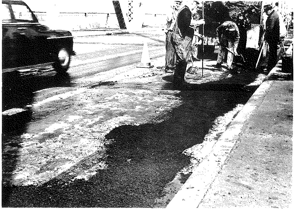
Fig. 27. Clark Memorial Bridge, Patching Deep Spalls, Hot-Mix Sand-Asphalt, March-April, 1960.
