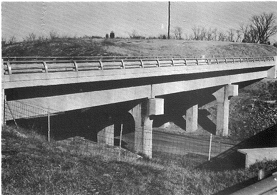
Fig. 105. Evergreen Road Bridge, I-64, Westbound, MP 37-905-HG4; Oblique View, Facing Eastwardly.
