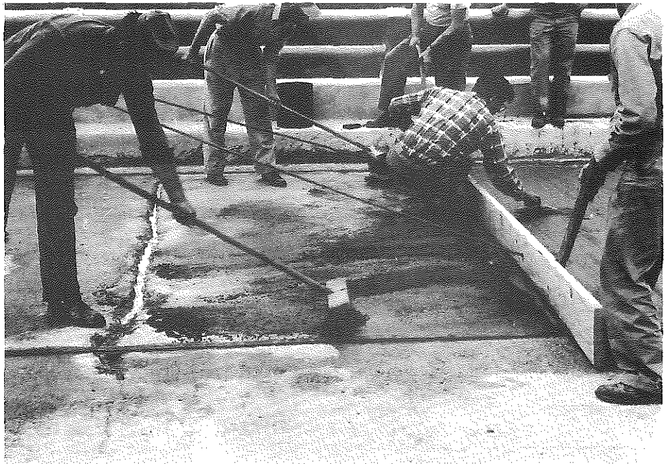
Fig. 59. Salt River Bridge, Kentucky Turnpike; Placing Latex (Dow 2144)-Mortar Overlay; Approximately 1/4 inch, October, 1960.
