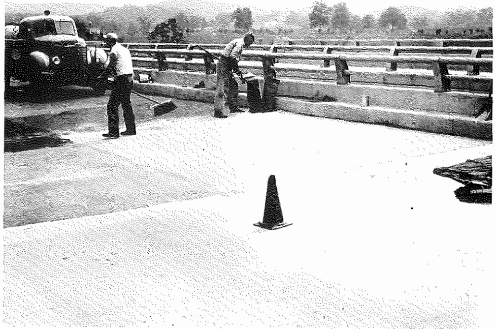
Fig. 74. Salt River Bridge, North-bound, Kentucky Turnpike; Brooming-Off Excess Sand, August 24-25, 1960.
