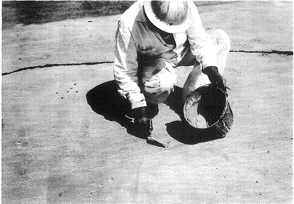
Fig. 55. Salt River Bridge, Kentucky Turnpike; Pointing-Up Pop-Outs with Penntrowel Mortar.
