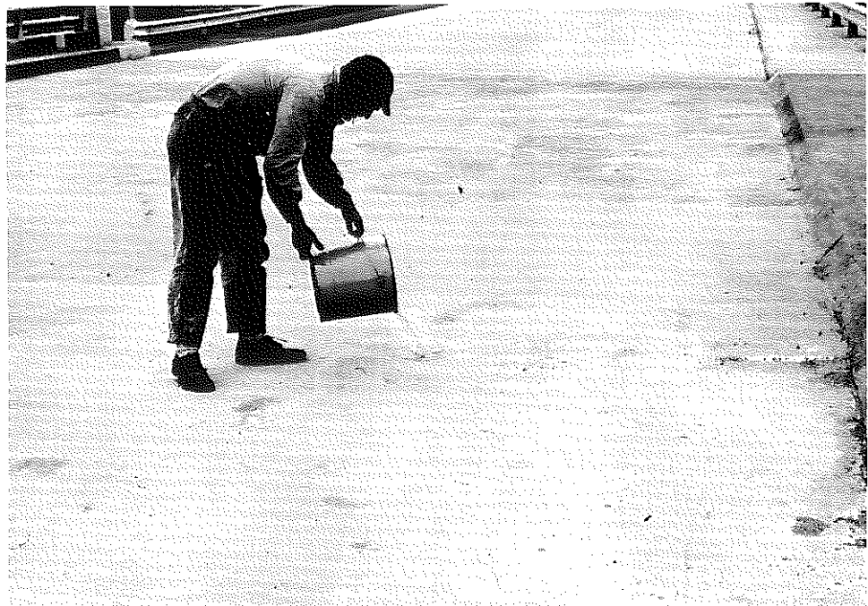
Fig. 36. St. Catherine's Street Bridge, Southbound Lanes, Looking North; Material Spread as Shown in Fig. 37.
