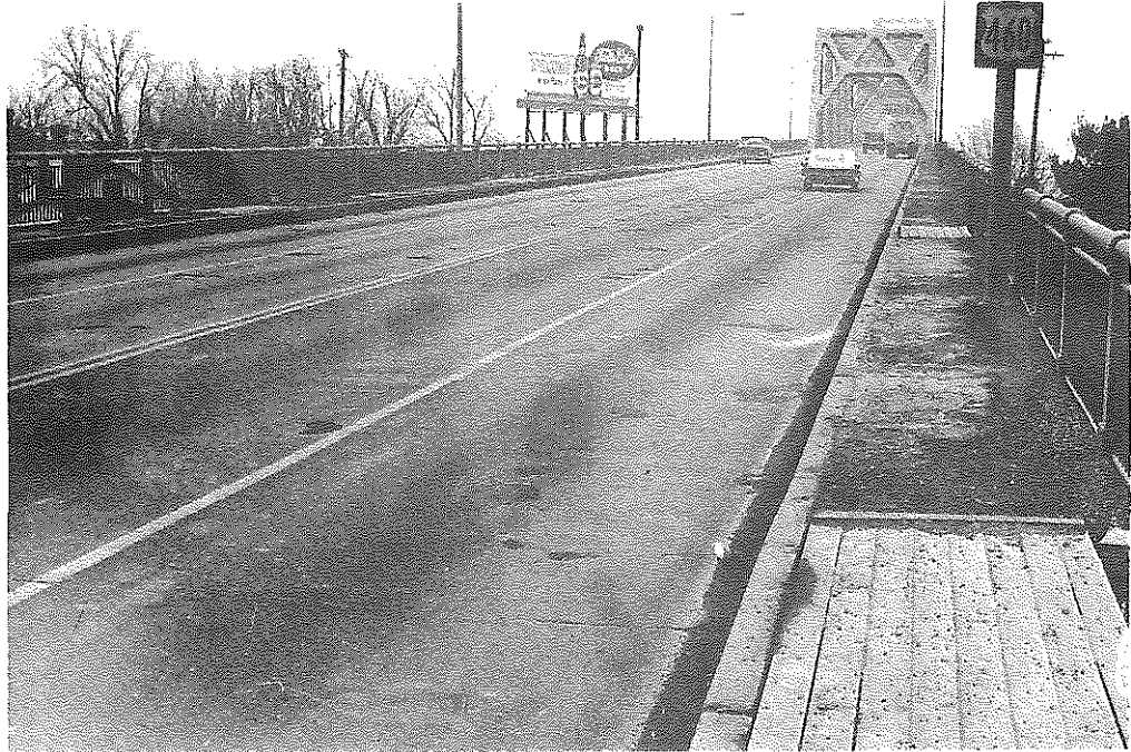
Fig. 29. Clark Memorial Bridge, January, 1962, After Black Beauty Slag Seal. Note Patches and Deterioration of Sidewalk.
