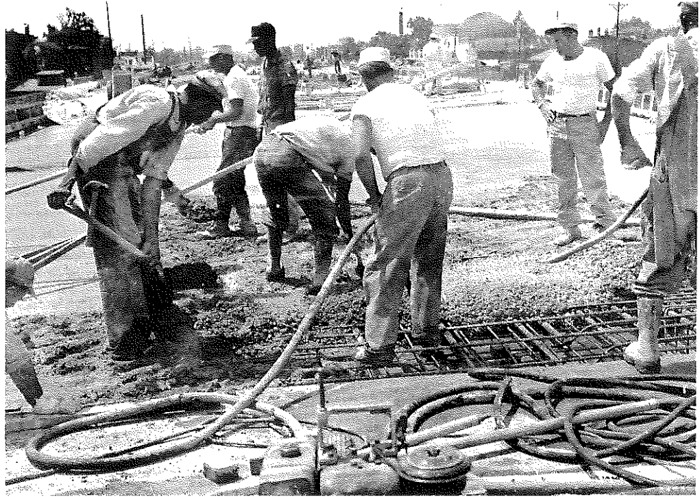
Fig. 1. Broadway Bridge, North-South Expressway, Louisville; I-65-6(6)134; June-July, 1960.
