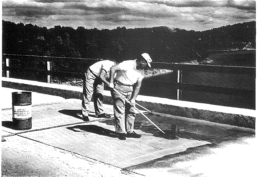
Fig. 97. Lake Cumberland Bridge; Eastbound Lane; Squeegee-Application of Dow 331 Epoxy Resin, September, 1961.
