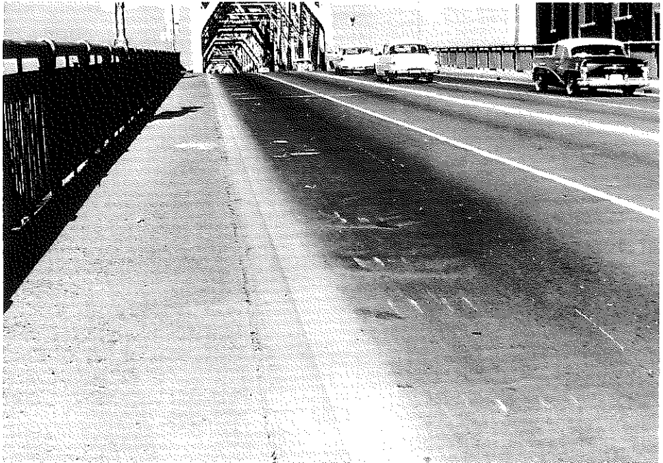
Fig. 22. Clark Memorial Bridge, South Ramp, November, 1959. Ripples in foreground are caused by deep sand-asphalt patches; one year after surfacing with sand-asphalt.
