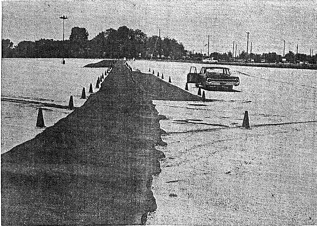
Fig. 10. Kentucky State Fairgrounds. The section containing all limestone aggregate and 16.6 percent SS-lh is on the left in the background. The section composed of blended sand, 1.25 percent portland cement, and 14.0 percent SS-lh is in the background between traffic hats. The section composed of blended sand, 12.0 percent SS-lh, and 2.5 percent portland cement is in the foreground.
