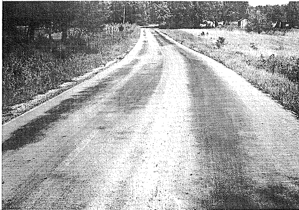
Fig. 4. Section of Surface Containing 6.5 Percent Asphalt (9-13-62).
