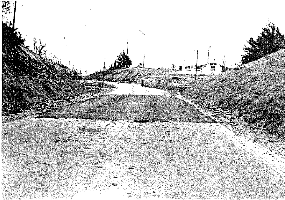
Fig. 9. Large Failure in Cut-Section. The failure occurred during the winter of 1962-63, and is located near the failure shown in Fig. 7. The surface contains 7.0 percent asphalt (4-8-63).
