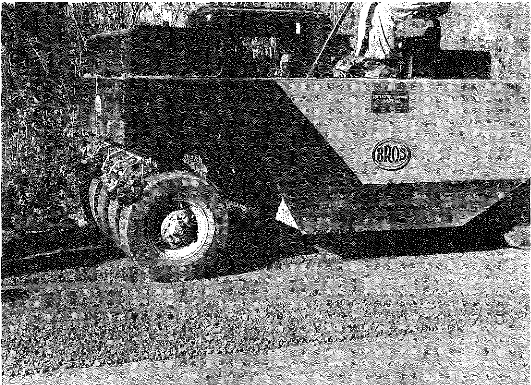
Fig. 4. RS 35-750. Compaction with the Pneumatic Tired Roller.
