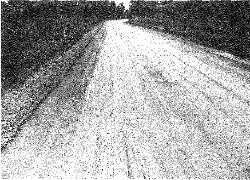
Fig. 5. RS 2-415. Compacted Granular Base, July, 1962.
