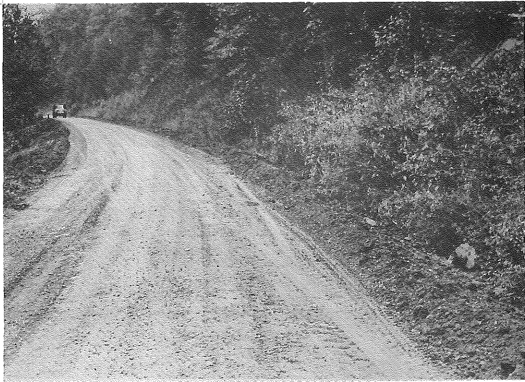
Fig. 2. RS 95-376. Existing Roadway Prepared for Application of Stone, September, 1962.
