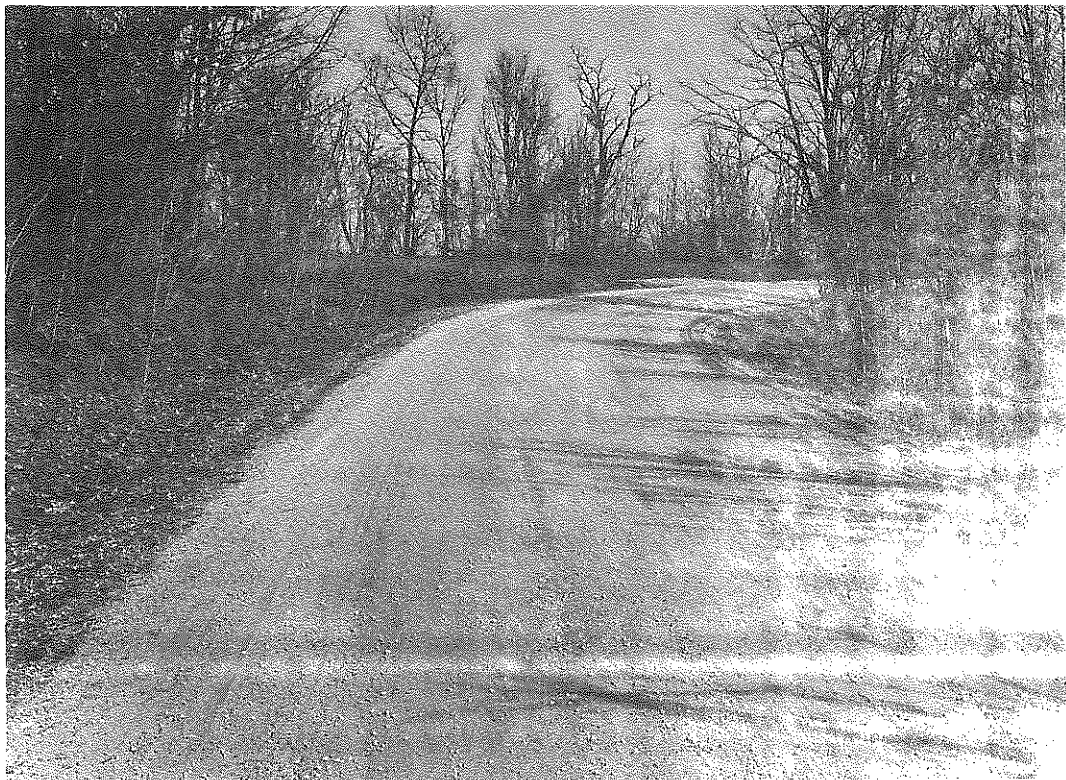
Fig. 4. RS 32-189. Condition of Roadway on February 5, 1963.
