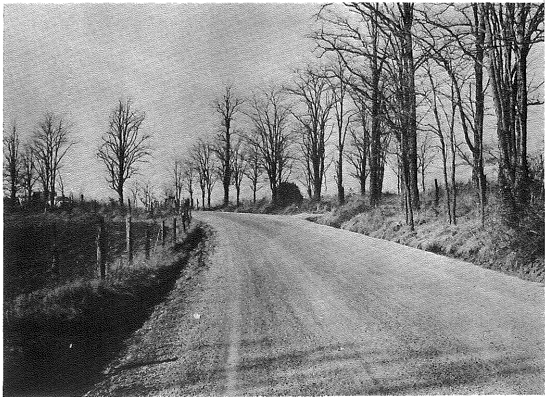
Fig. 6. RS 100-615. Condition of Roadway on January 22, 1963.
