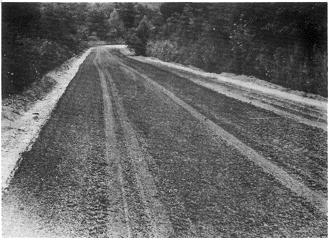
Fig. 4. RS 2-415. Granular Base Mixed and Spread Ready for Compaction.
