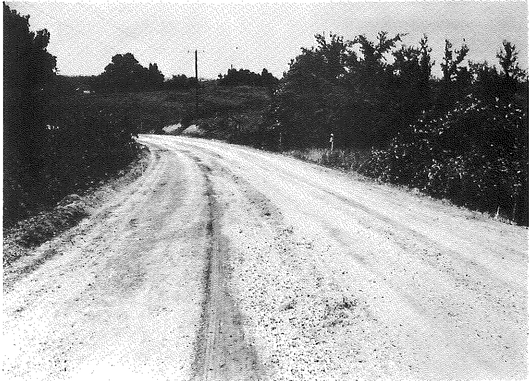
Fig. 1. RS 2-415. Existing Roadway Shaped and Prepared For Application of Stone.
