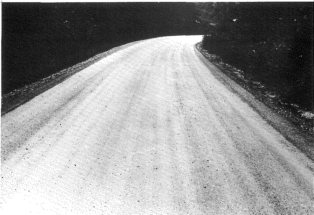
Fig. 4. RS 95-376. Compacted Granular Base, September, 1962.
