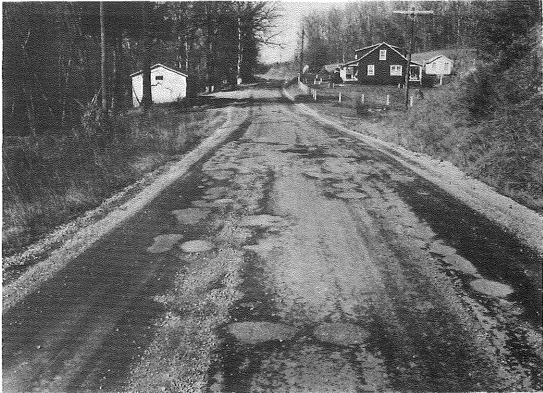
Fig. 9. RS 95-376. Condition of Roadway on February 6, 1963.
