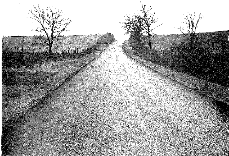
Fig. 1. RS 40-326. Condition of Roadway on February 13, 1962.
