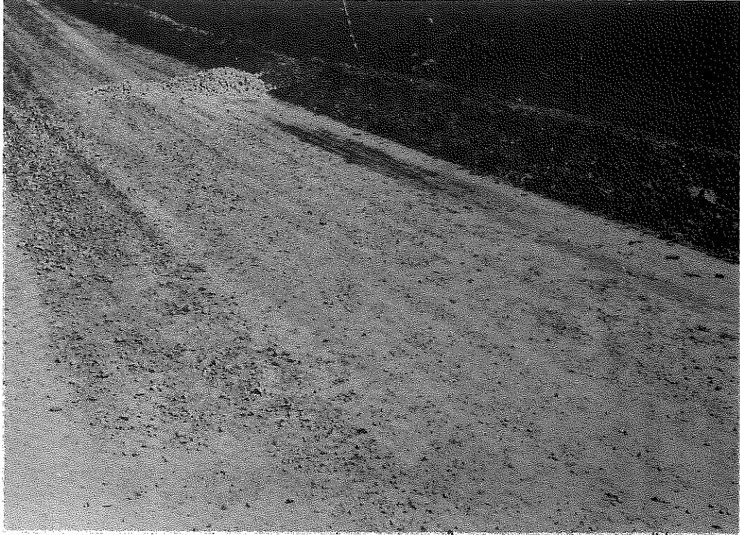
Fig. 3. RS 24-655-1. Shaped Roadway Prepared for Application of Stone. Note Drains.
