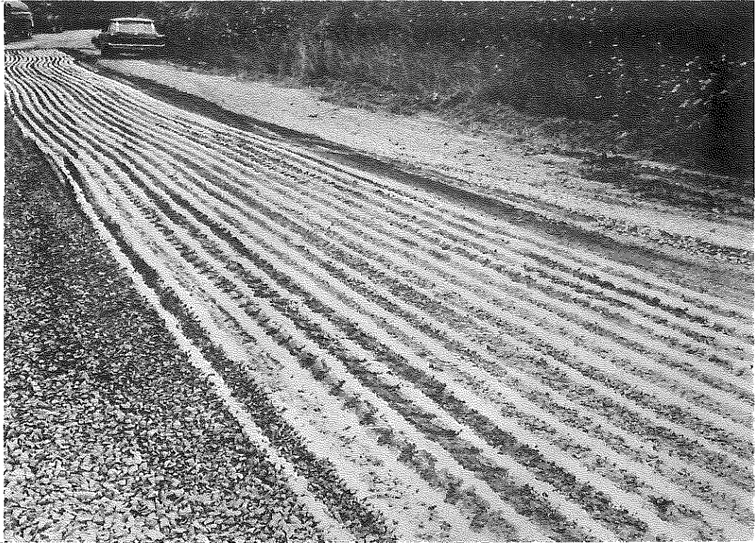
Fig. 3. RS 2-415. Application of Calcium Chloride.
