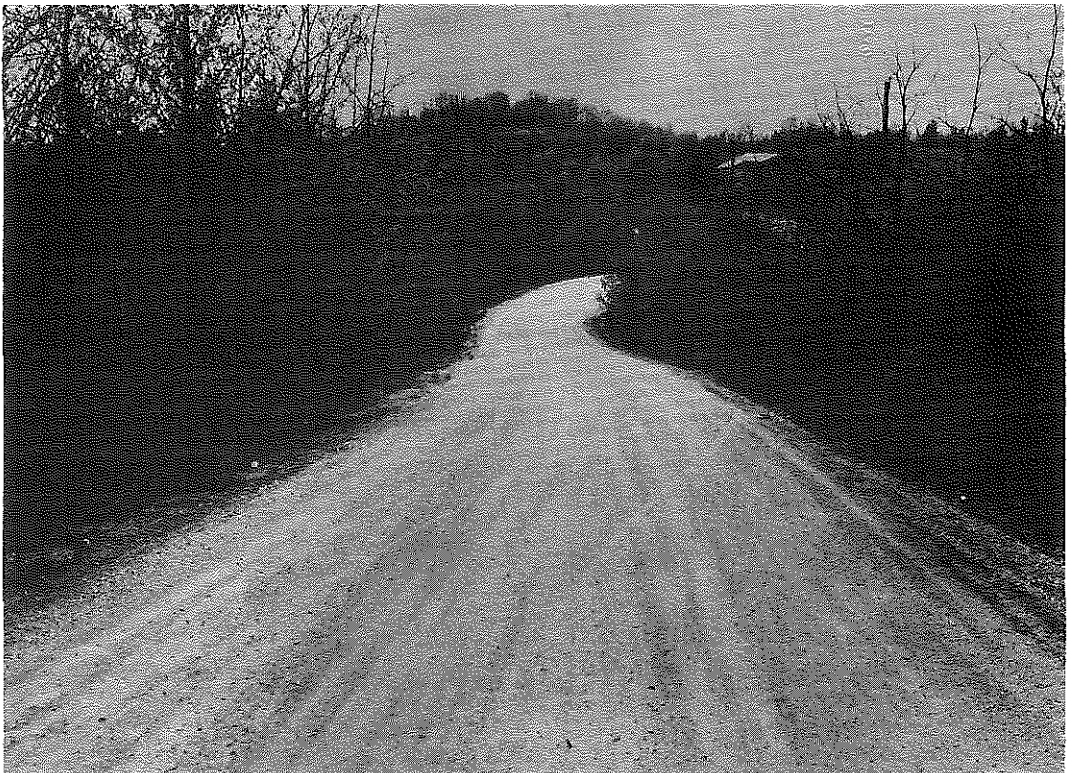
Fig. 8. RS 32-189. Condition of Roadway on April 23, 1963.
