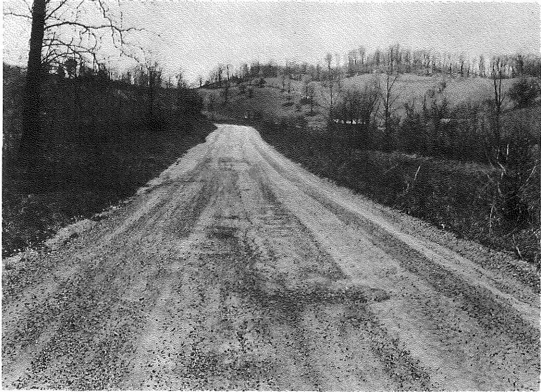
Fig. 11. RS 95-376. Condition of Roadway on April 15, 1963.
