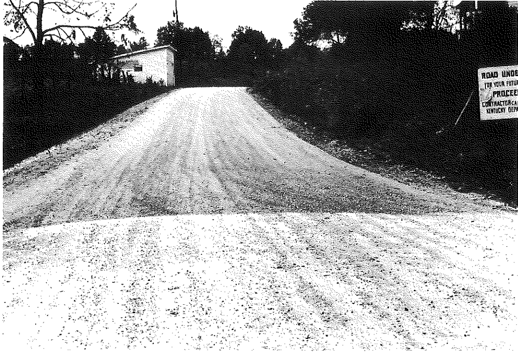
Fig. 7. RS 95-376. South End of Completed Project, September, 1962.
