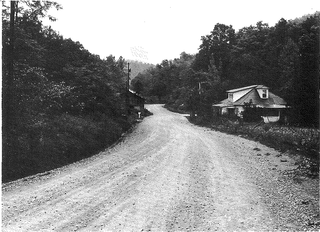
Fig. 1. RS 65-289. Condition of Roadway on May 23, 1962.
