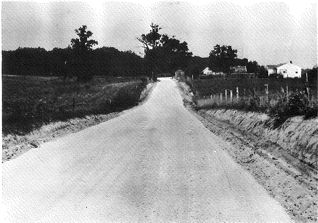
Fig. 2. RS 100-615. Shaped Roadway Prepared for Application of Aggregate, August, 1962.
