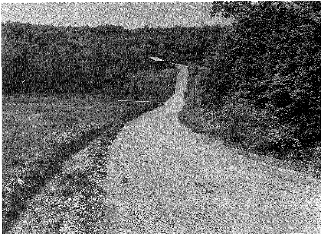
Fig. 2. RS 24-655-1. Condition of Western Portion of Project on May 9, 1962.
