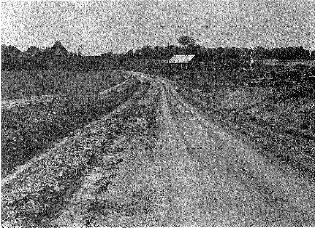
Fig. 1. RS 24-655-1. Condition of Roadway on Eastern-Most Mile of Project on May 9, 1962.
