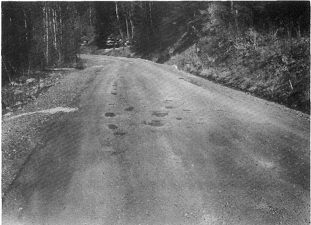
Fig. 4. RS 65-549. Condition of Roadway on February 6, 1963.
