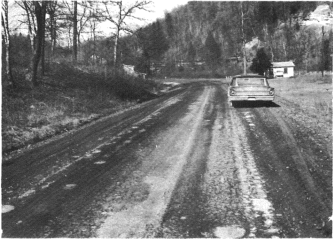
Fig. 3. RS 65-289. Condition of Roadway on February 6, 1963.
