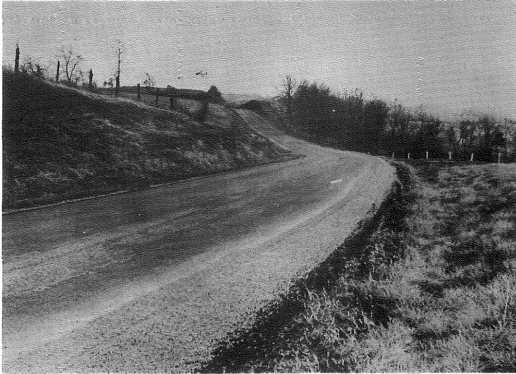
Fig. 3. RS 40-326. Condition of Roadway on December 27, 1962.
