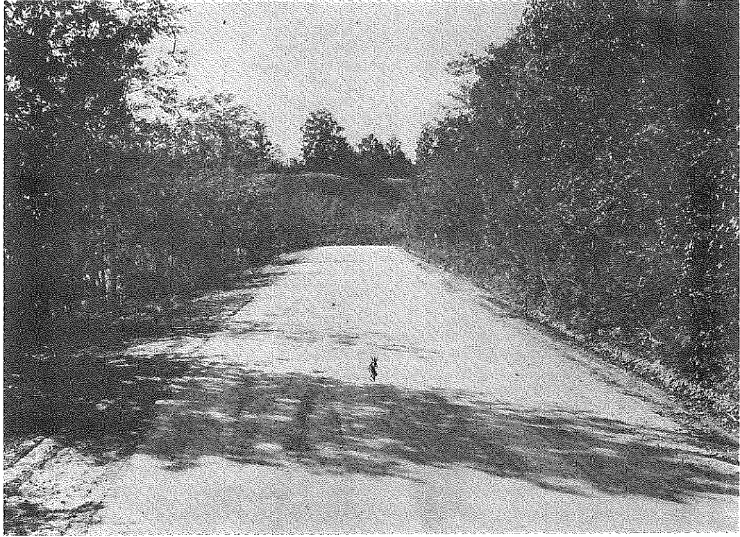
Fig. 3. RS 32-189. Compacted Granular Base, September, 1962.
