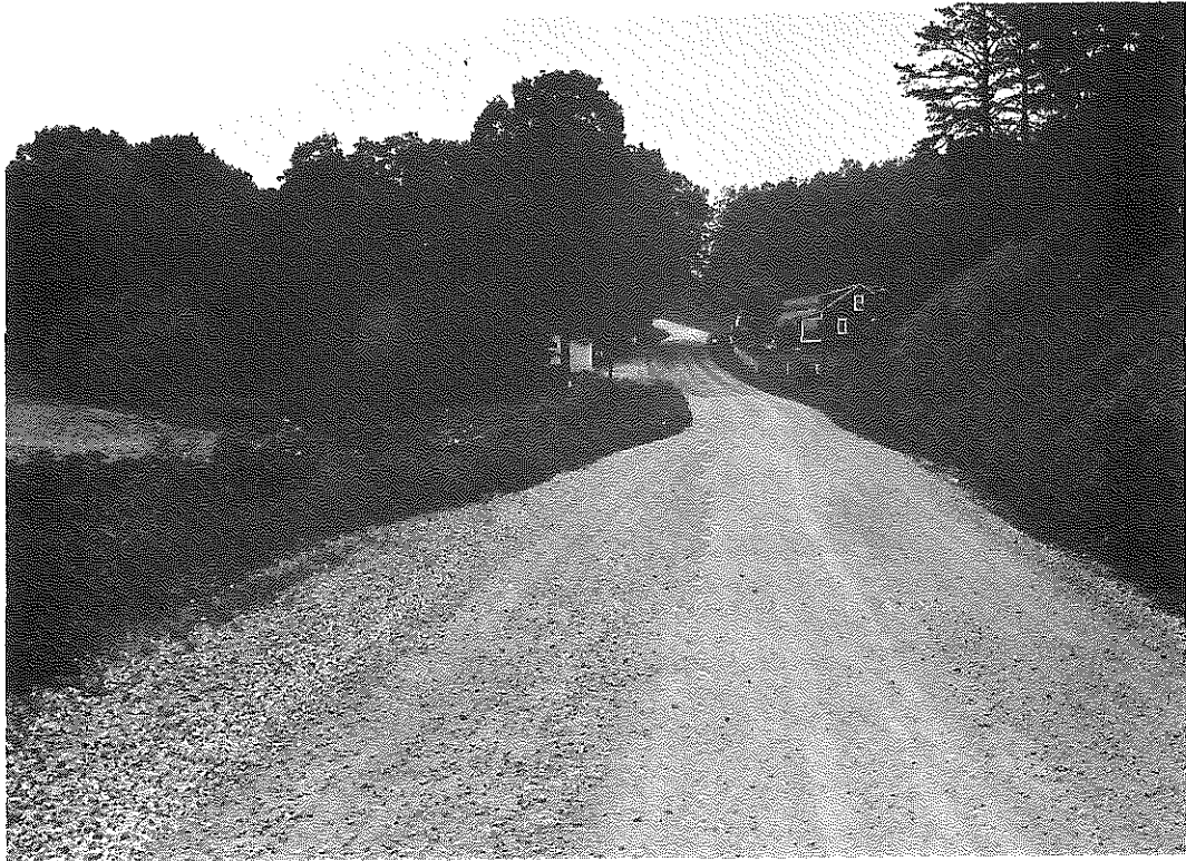
Fig. 1. RS 95-376. Condition of Roadway on May 23, 1962.
