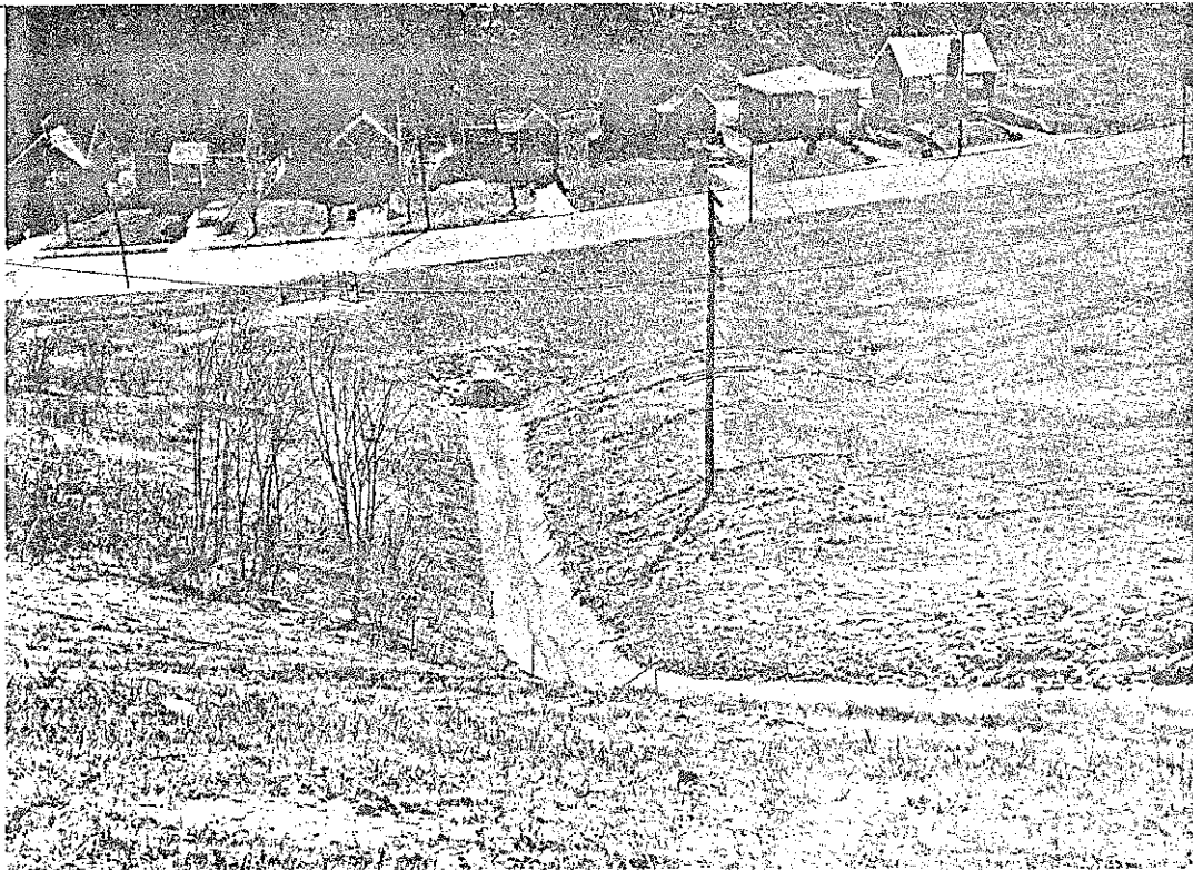
Fig. 9. Embankment Slope Shown in Figure 8. Note That Ditch Had Been Paved. Photograph Taken March 27, 1963.
