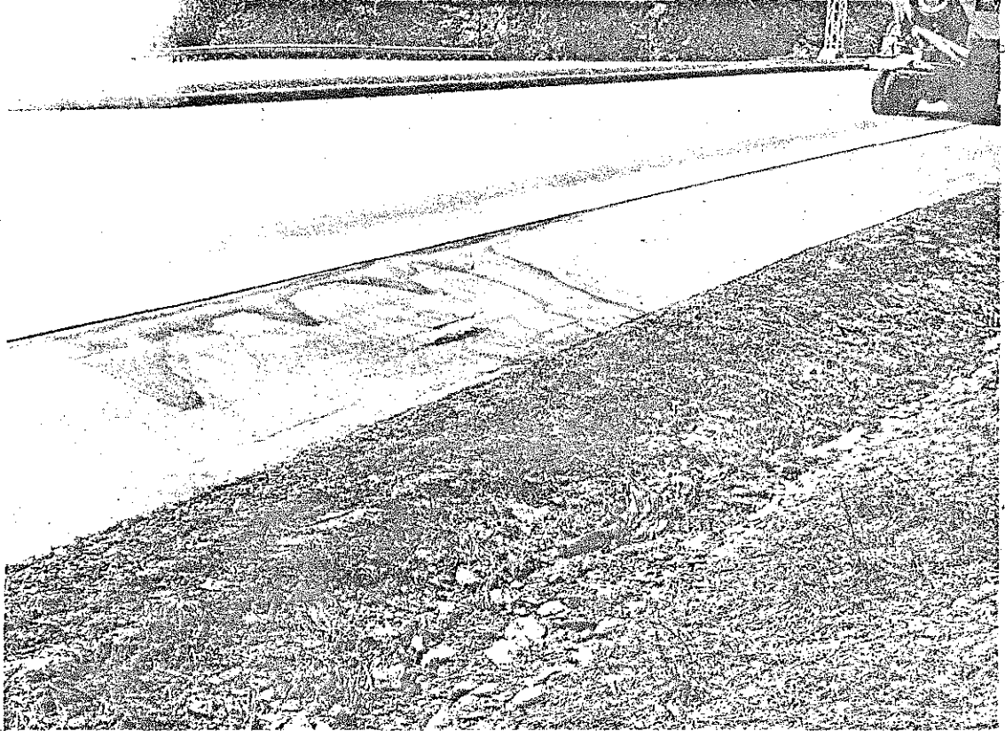
Fig. 16. Water Flowing Through the Joint Between the Shoulder and and Pavement, March 27, 1963.
