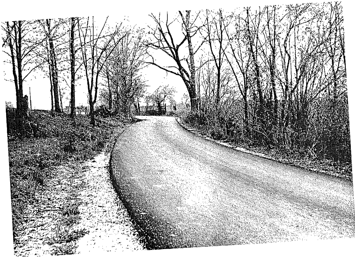
Fig. 1. Anderson County, RS3-911. General Condition of the Leathers Road (4-27-64)
