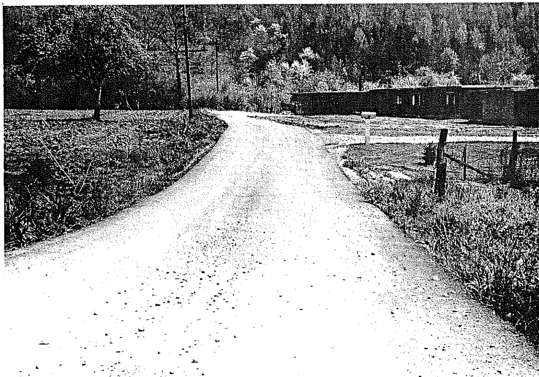
Fig. 18. Harlan County, RS48-898. General Condition of the Dupree Road (4-24-64)
