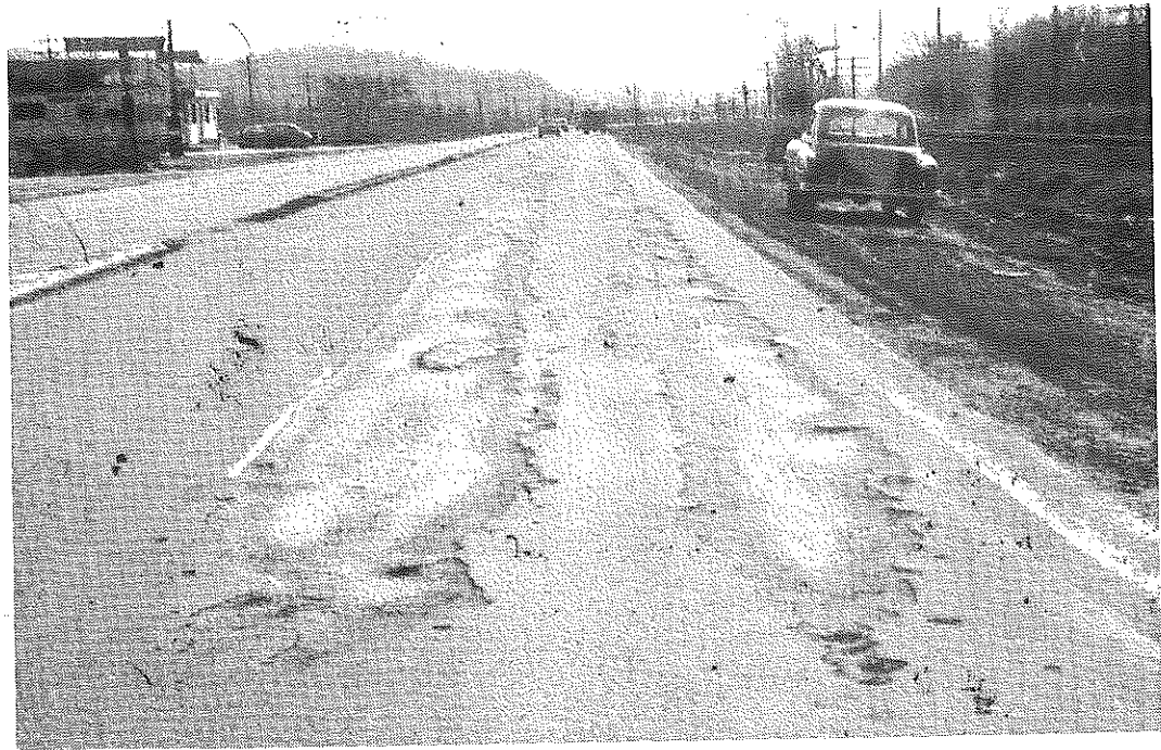
Figure 6. Illustration of Poor Performance Exhibited by Kentucky Rock Asphalt.
