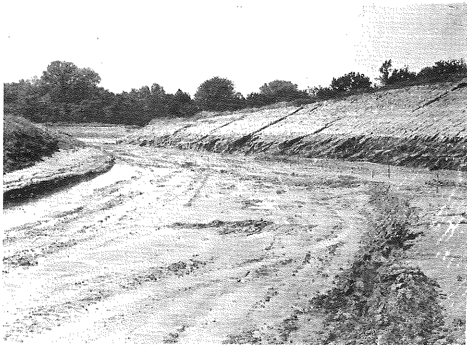
Figure 37. Photograph Showing Susceptibility of Wind-Blown Silt to Erosion.
