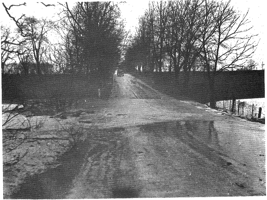
Figure 8. Illustration of the Importance of Hydrological and Hydraulic Criteria in the Design of Highway Drainage.
