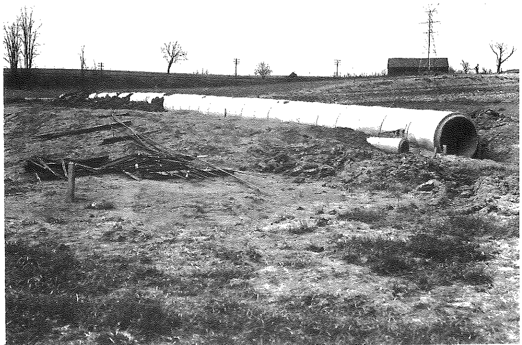
Figure 29. Field Installation of a Pipe Culvert Showing the Cambered Flow Line.
