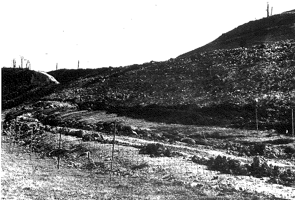
Figure 2. View of Upheaval at Toe of Failed Embankment.
