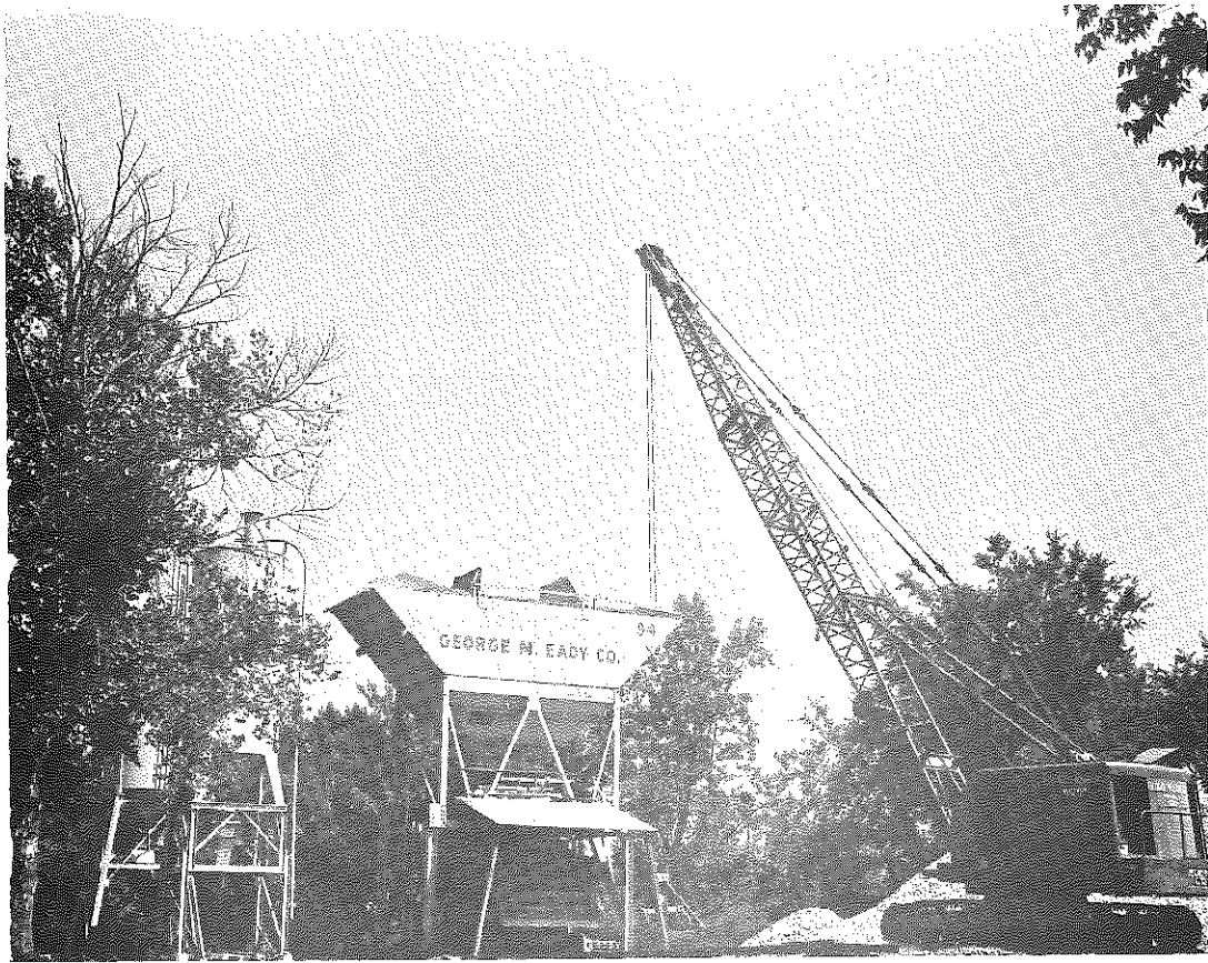
Fig. 3 - Dry-Batch Plant Site
