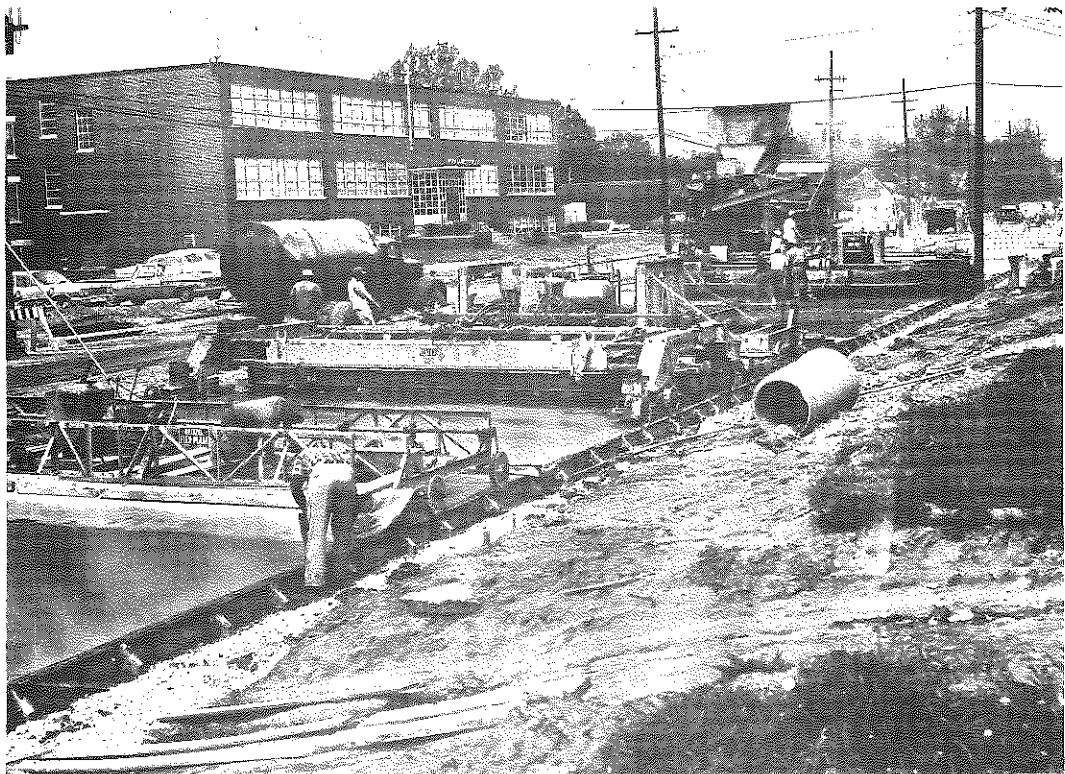
Fig. 6 - Consolidating and Striking-off
