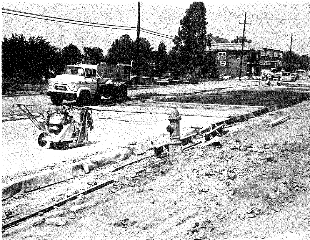
Fig. 11 - Pavement Initially Cured with Wetted Burlap; Final Cure with Kraft Paper.
