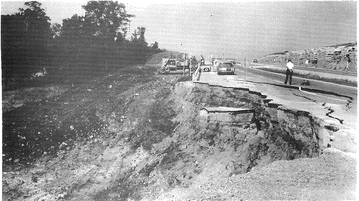
Figure 10-3. View of Slide Area, Looking West, in Late July, 1966.
