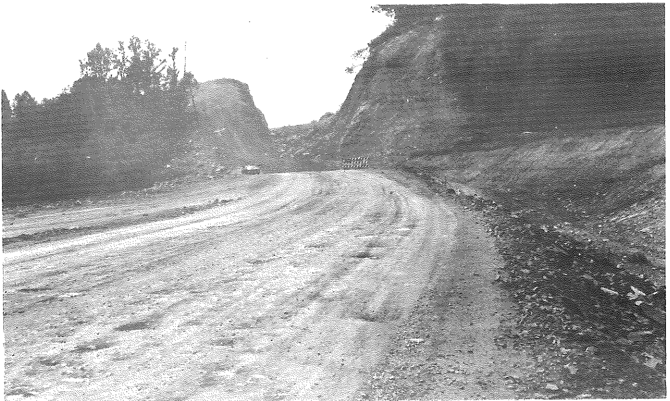
Figure 6-2. View of the Slide Area From the Northeast.
