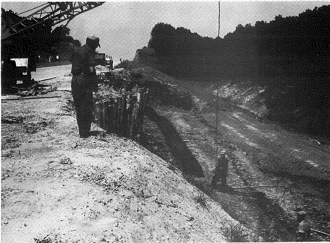
Figure 2-4. Site in Preparation for Driving Rail Piles, July, 1966.
