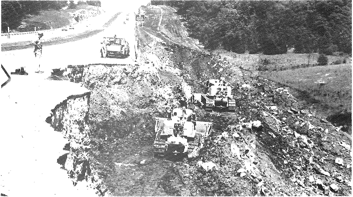
Figure 10-2. View of Slide Area, Looking East, Showing Removal of Unstable Material.
