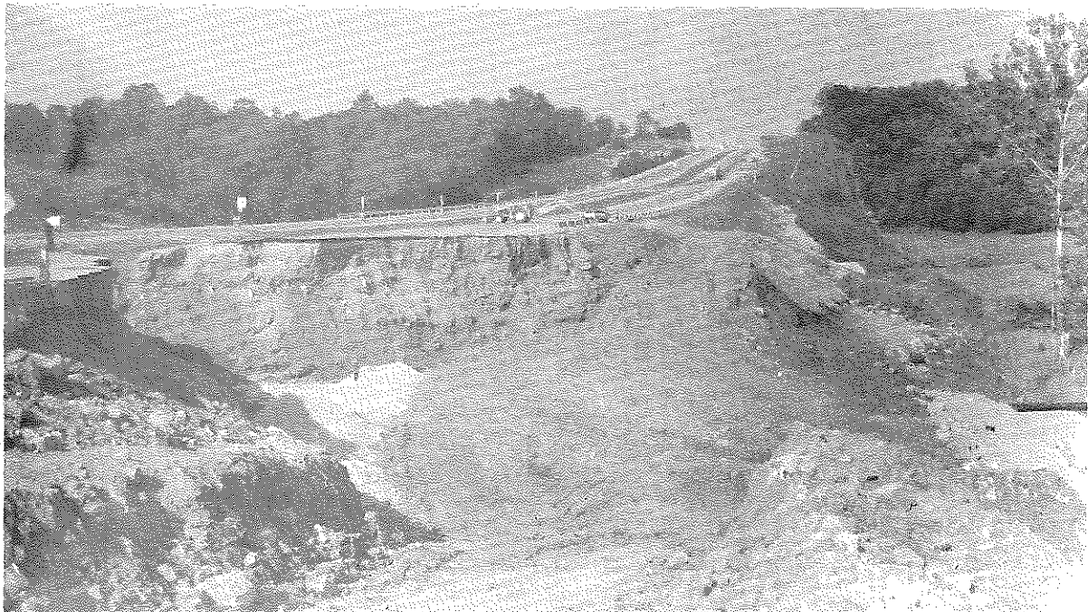
Figure 10-7. Free-draining, Granular Blanket and Pipe Outlet.
