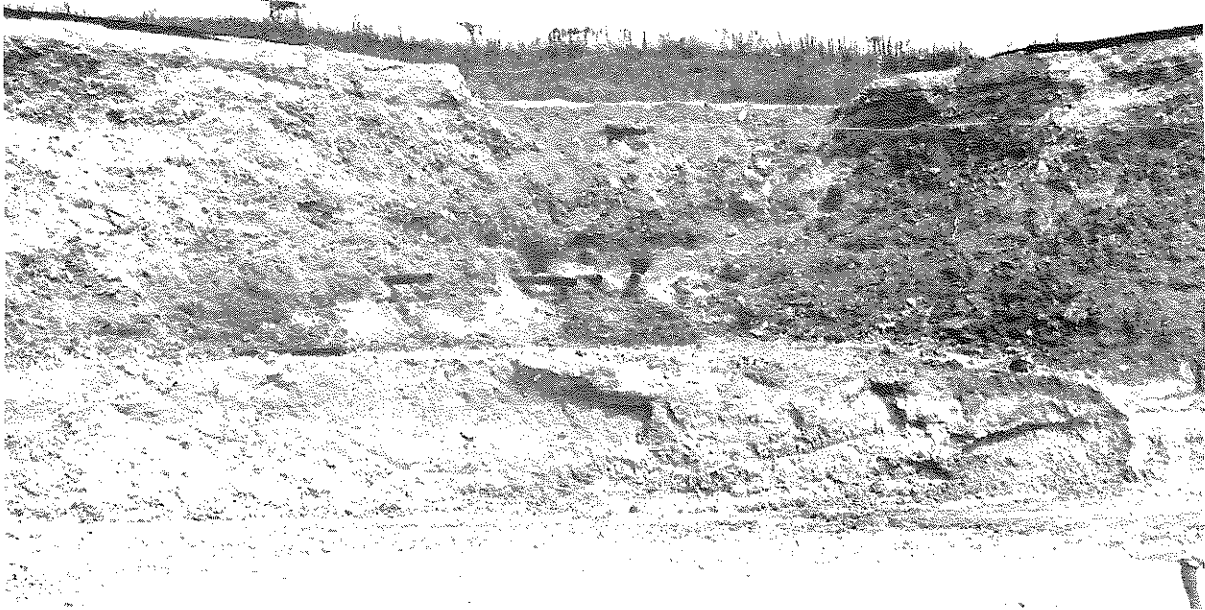
Figure 10-5. Excavated Slide Area Showing Benched Foundation and Horizontal Pipes.
