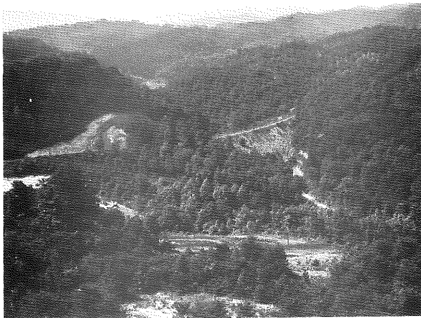
Figure 6 - The Rugged Terrain of the Eastern Coal Field. The photograph shows the deep cuts and high fills required in highway construction.
