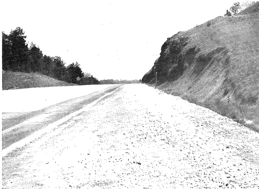
Figure 7. Typical Appearance of Anionic Emulsion-Treated Shoulder, May 1968. This section was covered with crushed stone shortly after treatment.
