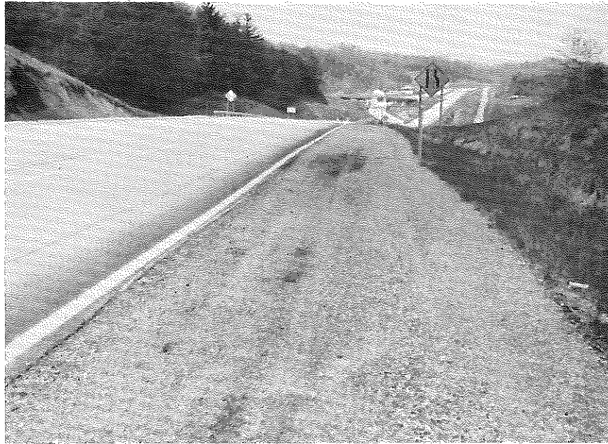
Figure 9. A Typical View of the Cationic Emulsion-Treated Shoulder, May 1968.
