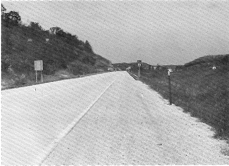
Figure 3. A Typical View of the Control Section at Mile Post 48.64, May 1, 1968.
