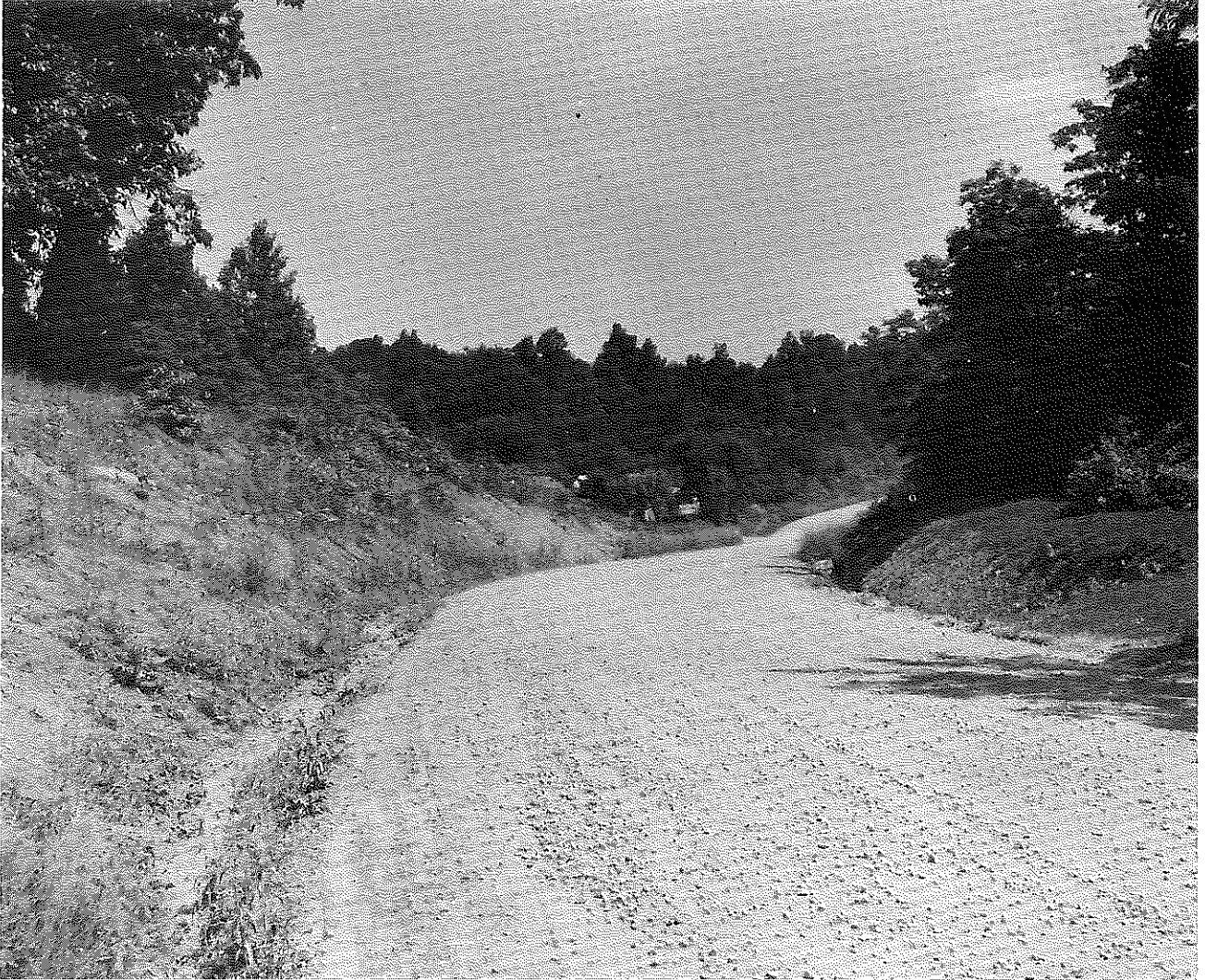
Fig. 2. View of the Roadway at Station 1+00 (South End of Project).
