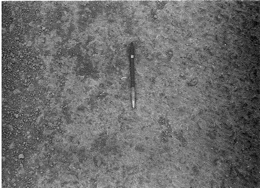
Fig. 12. Close-up View of the Untreated, Unsealed, DGA Base November 29, 1967. Note the loose stone (floaters) and the aggregate particles beginning to break from the surface.
