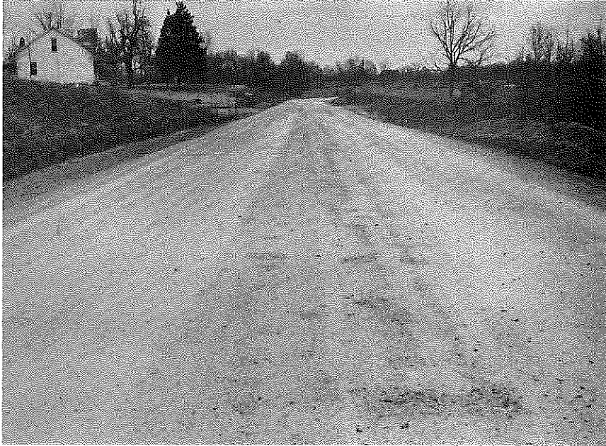
Fig. 13. An Overall View of the Salt-Treated, Unsealed, DGA Base, Station 38+00, November 29, 1967.
