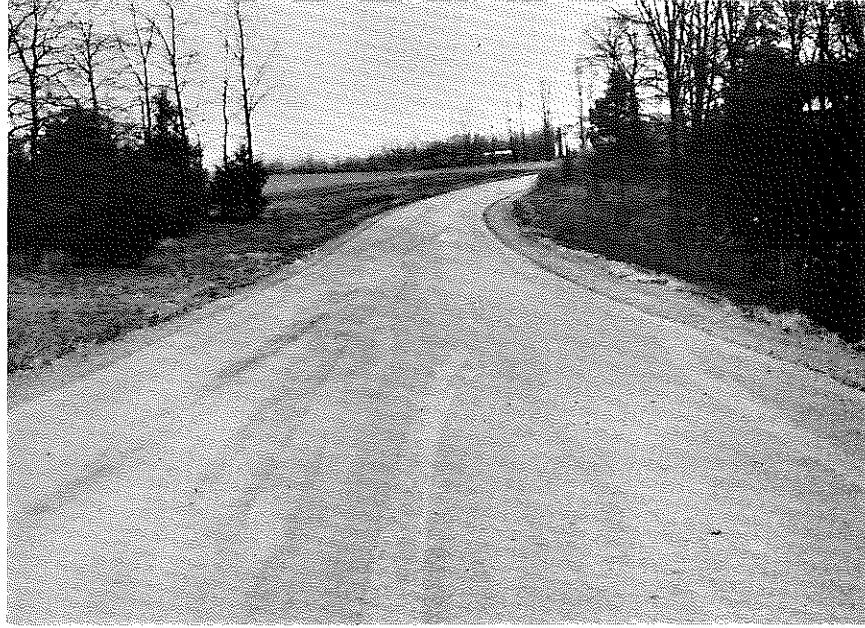
Fig. 15. Salt-Treated and Sealed, DGA Base, Station 68+00, November 29, 1967.
