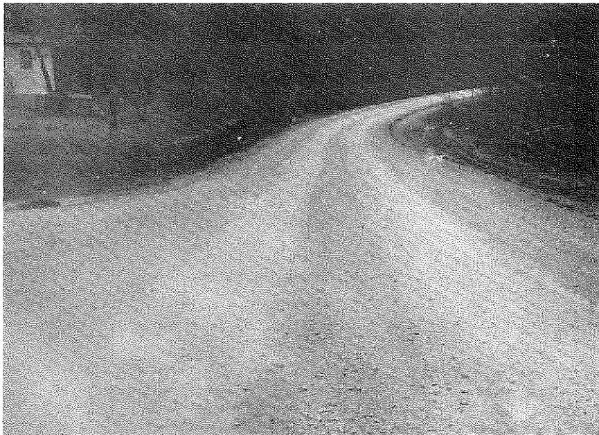
Fig. 16. Untreated and Unsealed, DGA Base, Station 5+00, November 29, 1967
