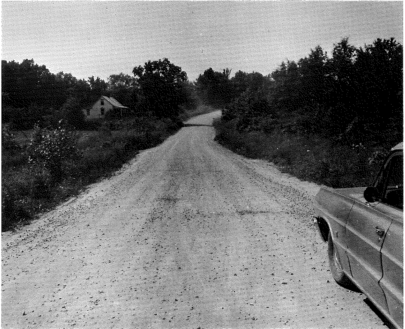
Fig. 3. View of the Roadway at Station 142+00 (North End of Project).
