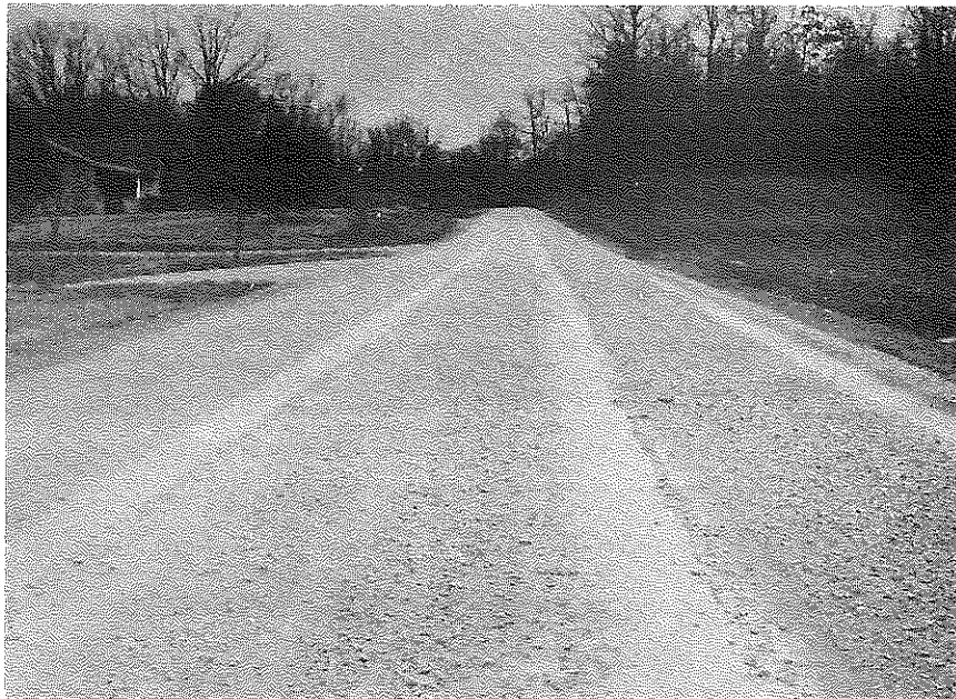
Fig. 14. An Overall View of the Untreated, Unsealed, DGA Base, Station 20+00, November 29, 1967. Note the large amount of loose stone from the base. The base, beneath the loose stone, was tight and dense.
