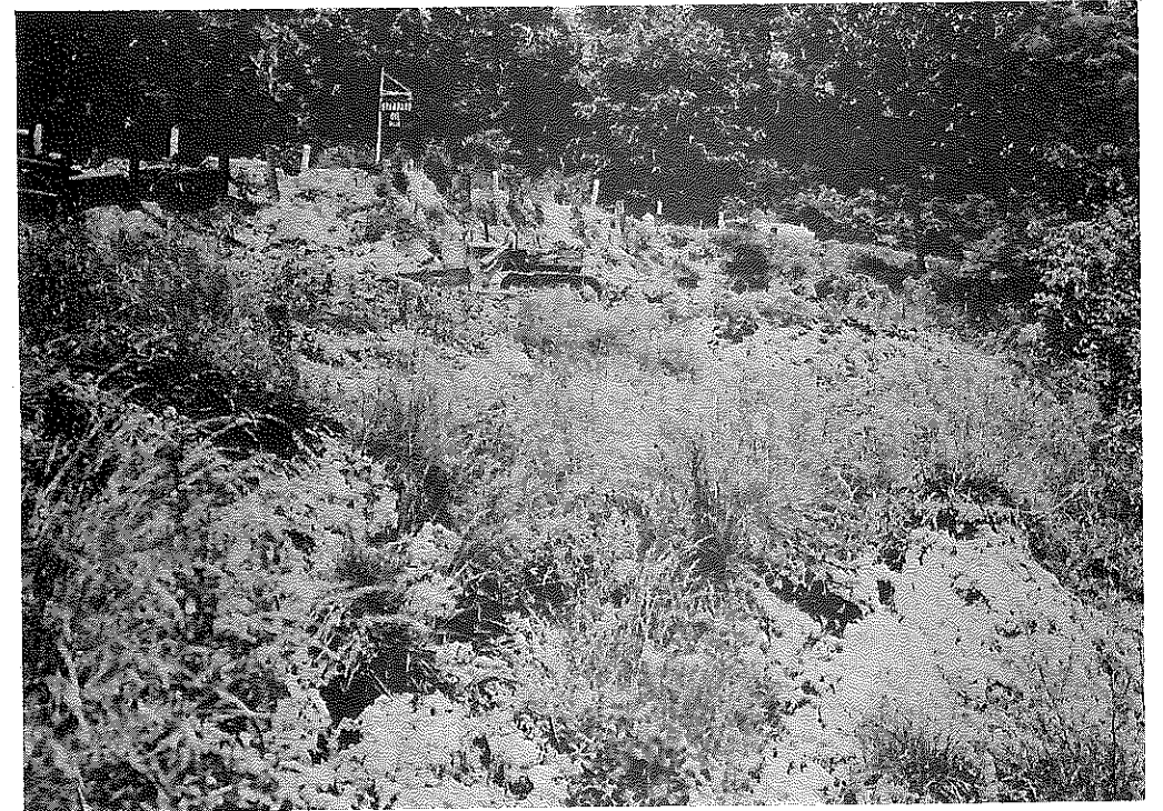
Figure 19. Photograph 3 (See Figure 15) of Slide Area, KY 89, Clark County.
