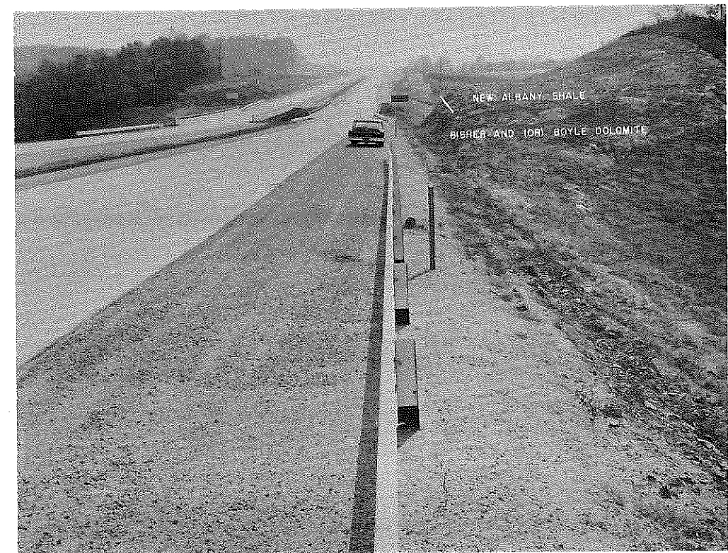
Figure 29. Slide Area, Mountain Parkway, Clark County.
