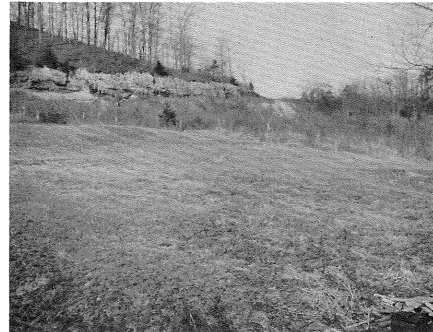
Figure 25. Landslide Area, KY 1840, Estill County.
