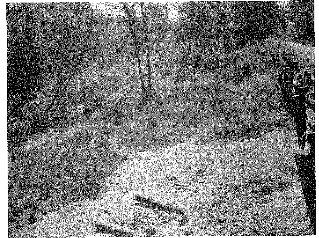
Figure 21. Photograph 5 (See Figure 15) of Slide Area, KY 89, Clark County.
