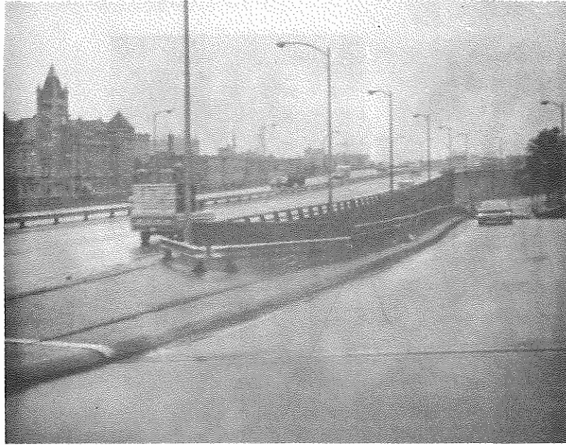
FIGURE 42. Location 12; Jefferson County, I 65 - Chestnut Street Interchange, Gore at Northbound Exit from I 65 to Chestnut Street
