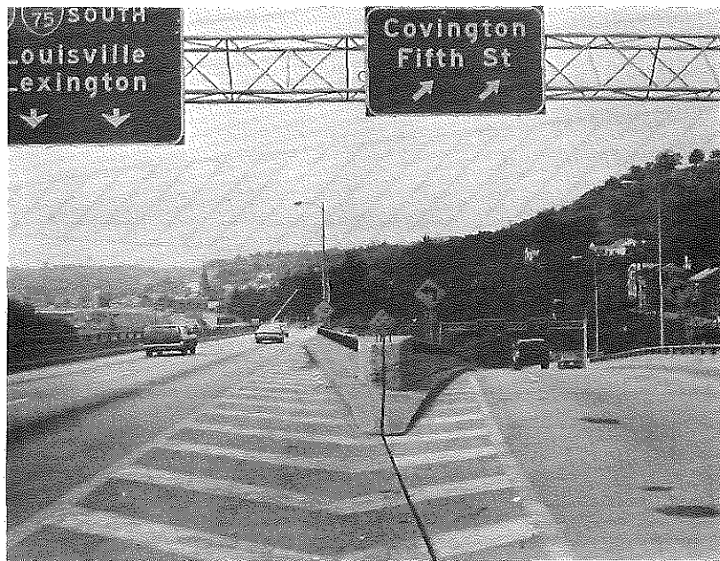
FIGURE 29. Location 7; Kenton County, I 75 - 5th Street Interchange , Gore at Southbound Exit Ramp, before Installation of FITCH Barrier
