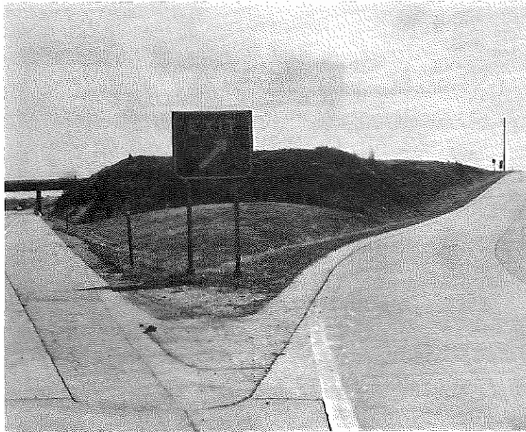
FIGURE 38. Location 9; Shelby County, I 64 - KY 395 Interchange, Gore at Eastbound Exit from I 64 to KY 395
