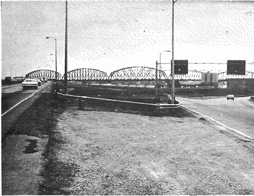
FIGURE 21. Location 3 (c) after Guardrail Removal and Contour Grading
