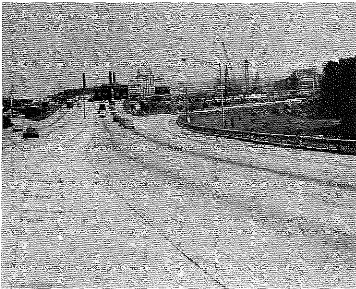
FIGURE 17. SINGLE-LANE EXIT WITHOUT TAPER (I 75 NORTHBOUND AT THE 5TH STREET EXIT IN COVINGTON)
